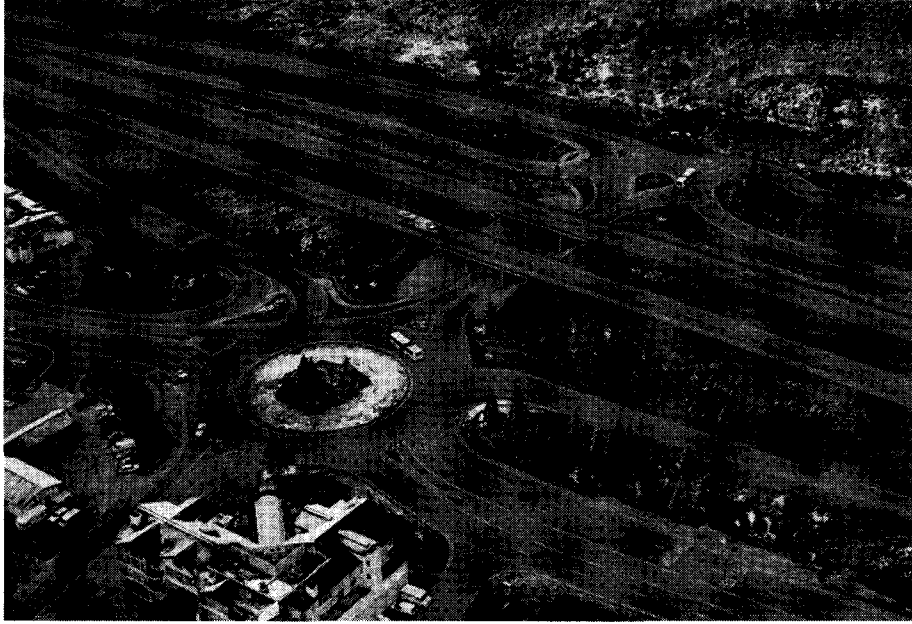
FIGURE 32 Aerial view of roundabout at I-70 and Vail Road, Vail Colorado ( courtesy of MK Centennial ).
