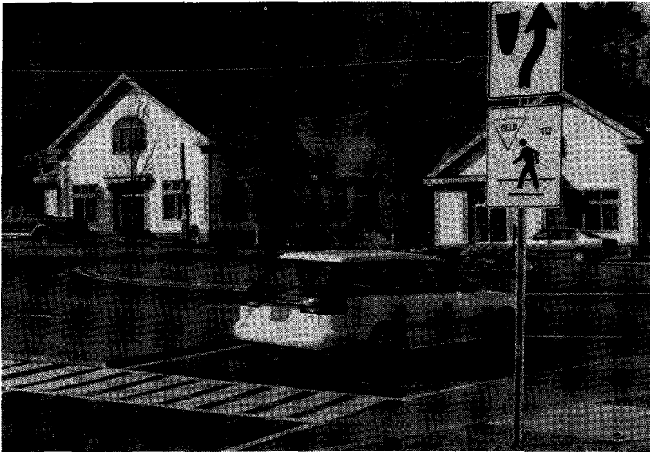
Mountable splitter island, signs and markings in Manchester, Vermont ( Courtesy of Tony Reddington ).
