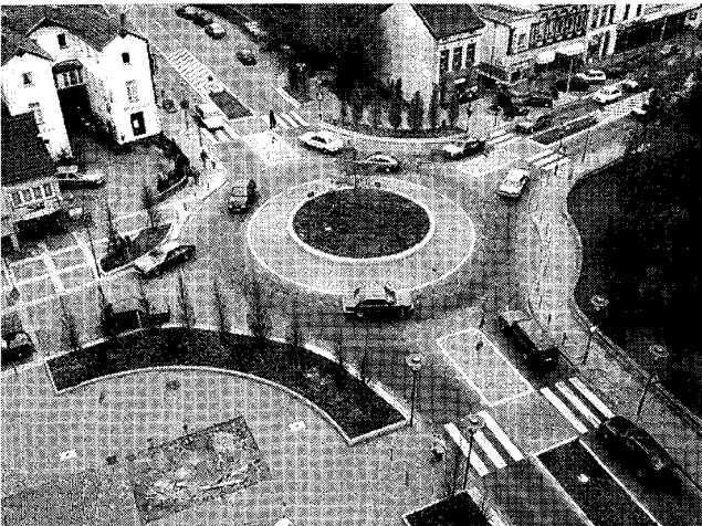
FIGURE 8 Before and after views of intersection in Brühl, Germany (11).
