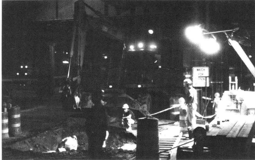
FIGURE 26 Aim construction lighting fixtures down when possible.
