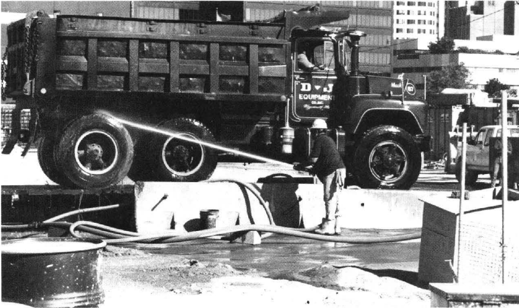
FIGURE 27 Urban project egress point wheel wash station.
