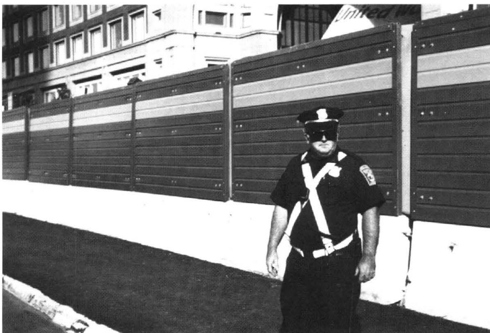
FIGURE 13 Movable noise barrier mounted on jersey bases.
