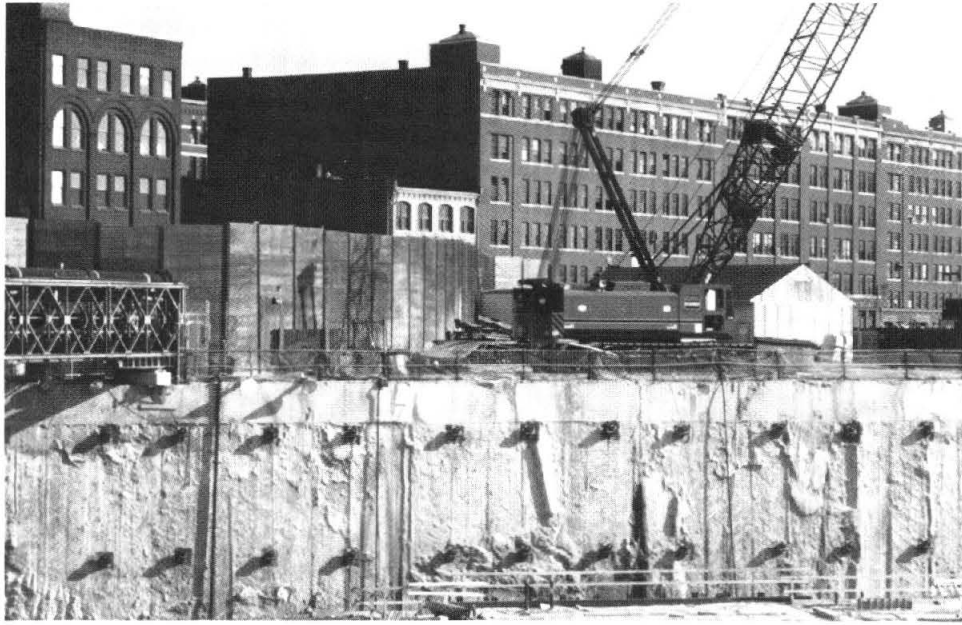
FIGURE 14 Semi-permanent noise barrier wall.
