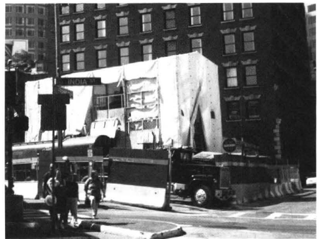
FIGURE 11 Slurry plant enclosure for audio-visual and dust control.
