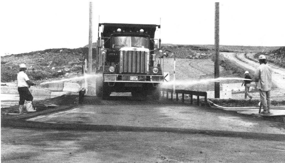
FIGURE 28 Dump site wheel wash station.
