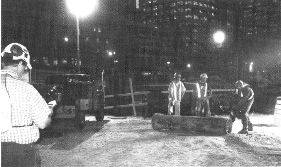
FIGURE C-1 Sound measurements for monitoring noise during construction.
