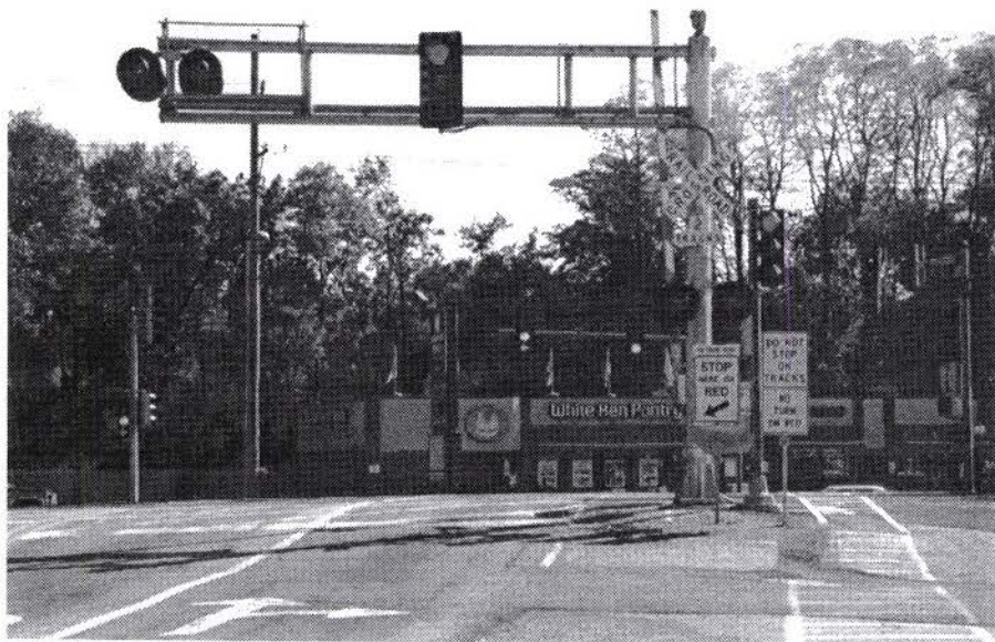
Algonquin Road Highway-Rail Grade Crossing (at US Route 14) Fox River Grove, Illinois (on the METRA/Union Pacific Northwest Line)
