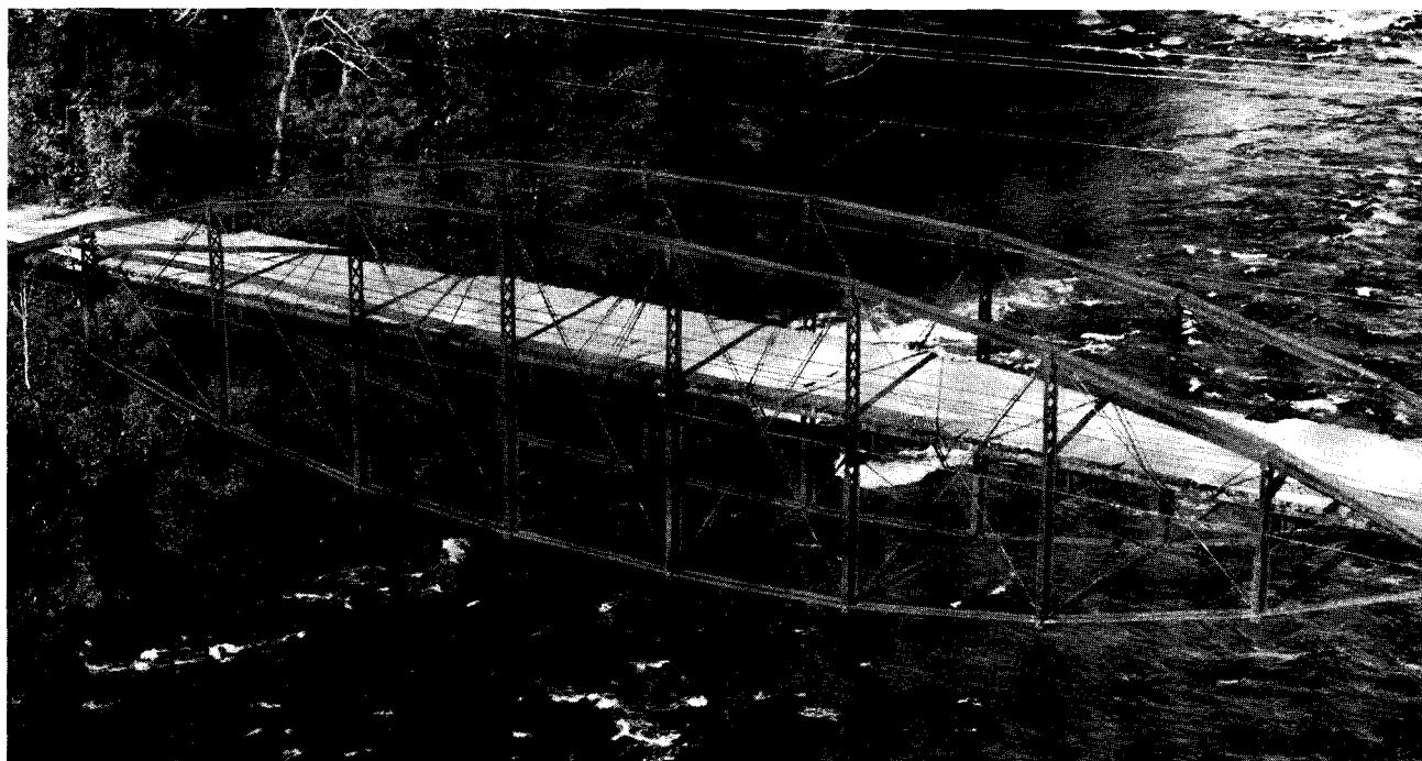
FIGURE 3 Old Corinth Road Bridge over the East Branch of the Sacandaga River, Hadley, New York (photo credit: Jet Lowe).
