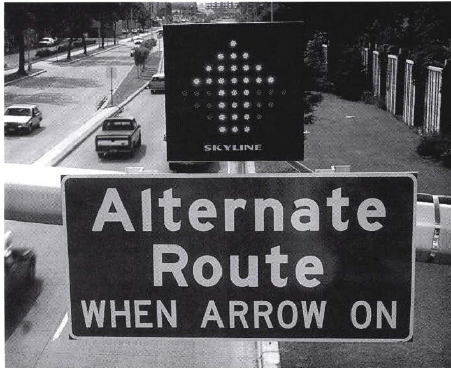
FIGURE 10 The Minnesota DOT has installed permanent route guidance signs on some preplanned alternate routes in the Twin Cities. (Photo courtesy of the Minnesota DOT.)
