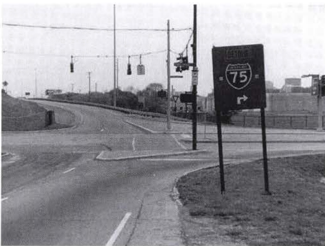
FIGURE 11 Dayton, Ohio, has erected permanent detour signs along six preplanned alternate routes for three sections of I-75 within the city limits. (Photos courtesy of the Dayton Police Department.)
