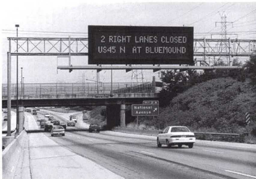
FIGURE 8 Dynamic methods of communicating a continuous flow of information to motorists makes for a more effective freeway management system. (Photo courtesy of the Wisconsin DOT.)
