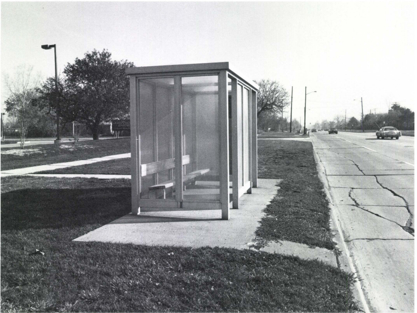
This photo clearly shows the bench inside the shelter and how the pad is connected to the sidewalk and road curbing with concrete paths. See Figure 29 for shelter space requirements.
