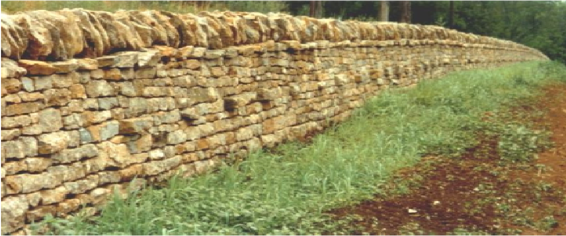
Figure 8. Relocated Dry-Laid Stone Fence on Paris Pike, Kentucky
