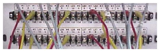
b) Controller Cabinet Backpanel (Must Connect Clips Here) **Figure 5-2:** Backpanel Mount Procedure (Requires Controller Cabinet)
