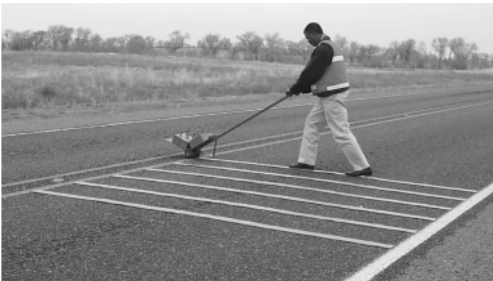
Figure 7. Portable Rumble Strips Installation.
