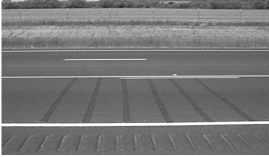
Figure 8. Removal of Rumble Strips.
