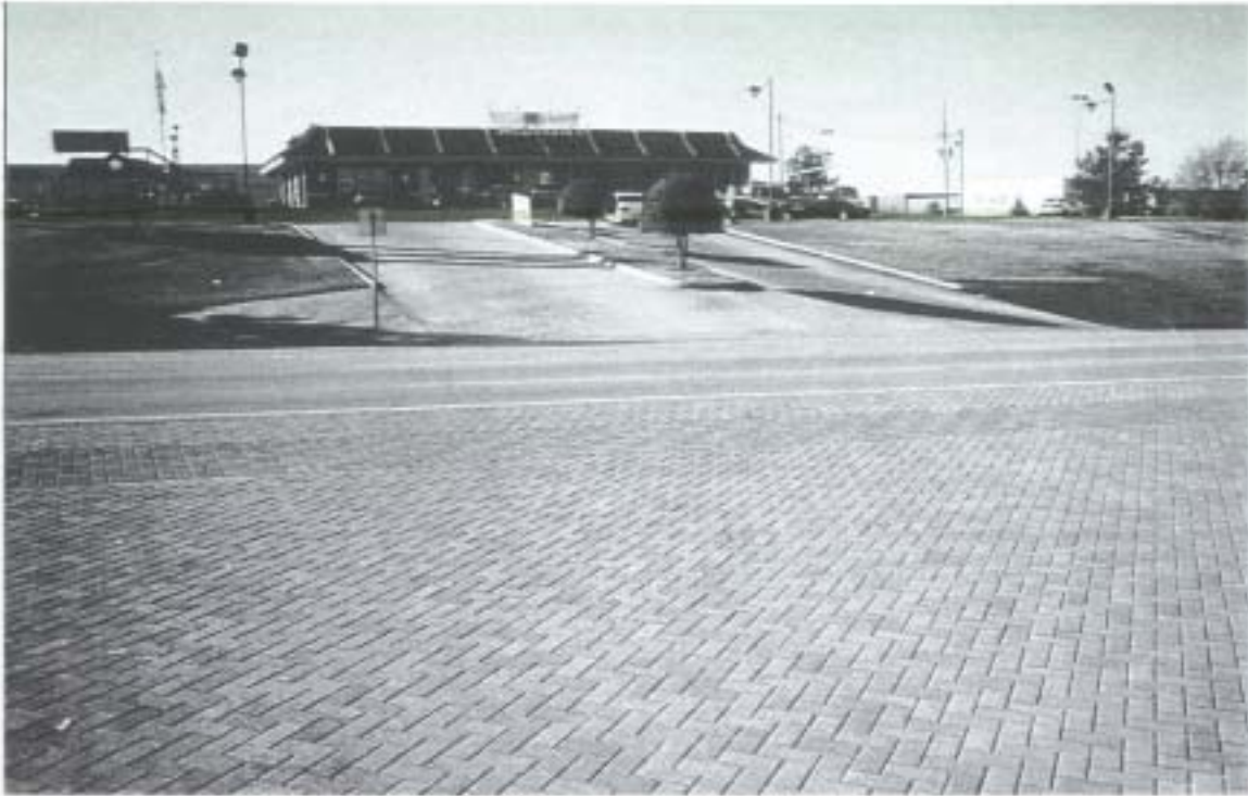
Figure 2-28. Facing South on Loop 281 West of Tuttle Road.
