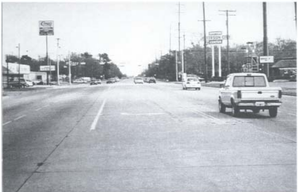
Figure 2-20. Southbound Twin Cities Highway at 33 rd Street.
