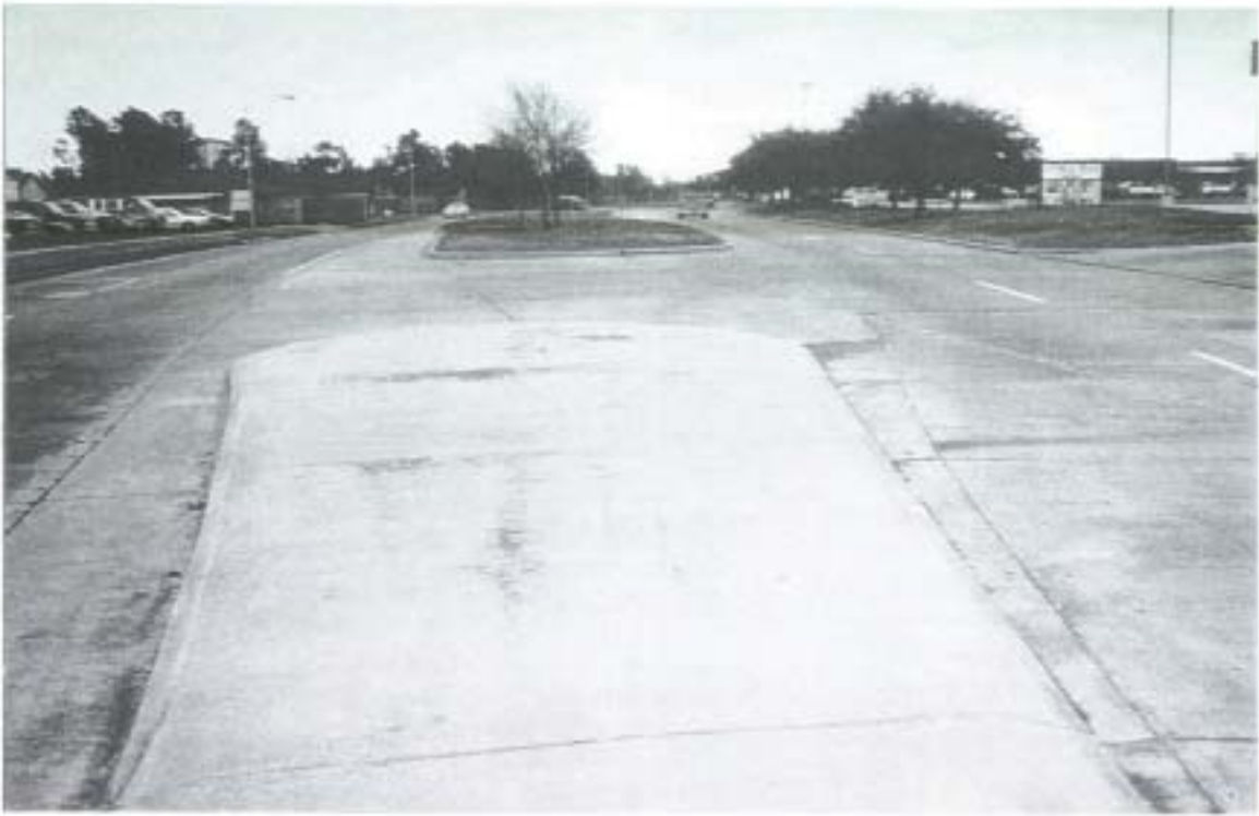
Figure 2-21. Southbound 9 th Avenue at Texas 365.
