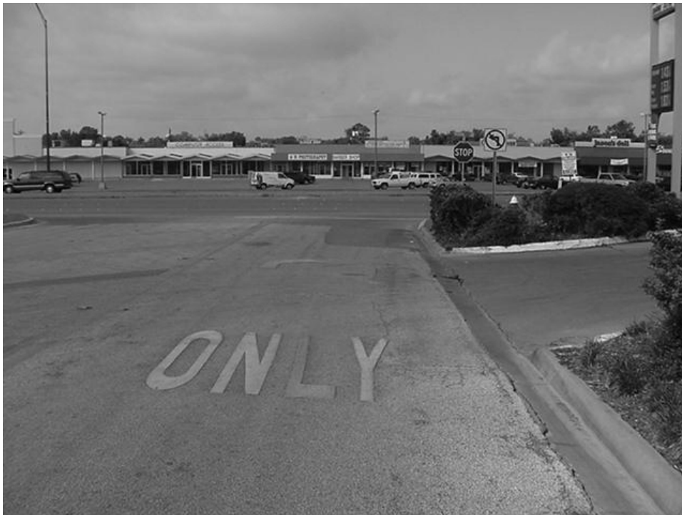
Figure 2-3. Dominik Drive at Texas Avenue without a Median Opening After Construction.
