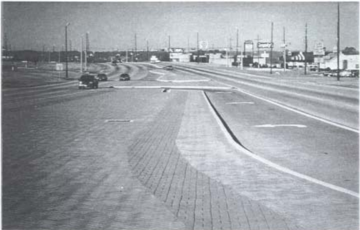
Figure 2-27. Westbound Loop 281 between Judson Road and Tuttle Road.
