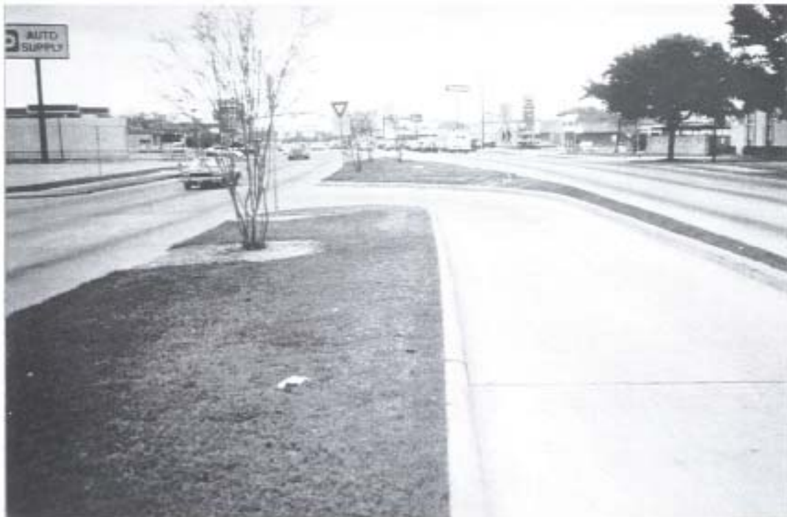
Figure 2-6. Southbound South Post Oak Road Illustrating Channelized Median.
