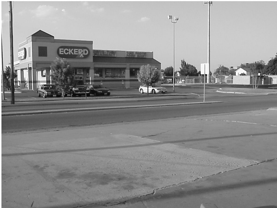
Figure 2-36. Line Avenue East of Georgia Street.
