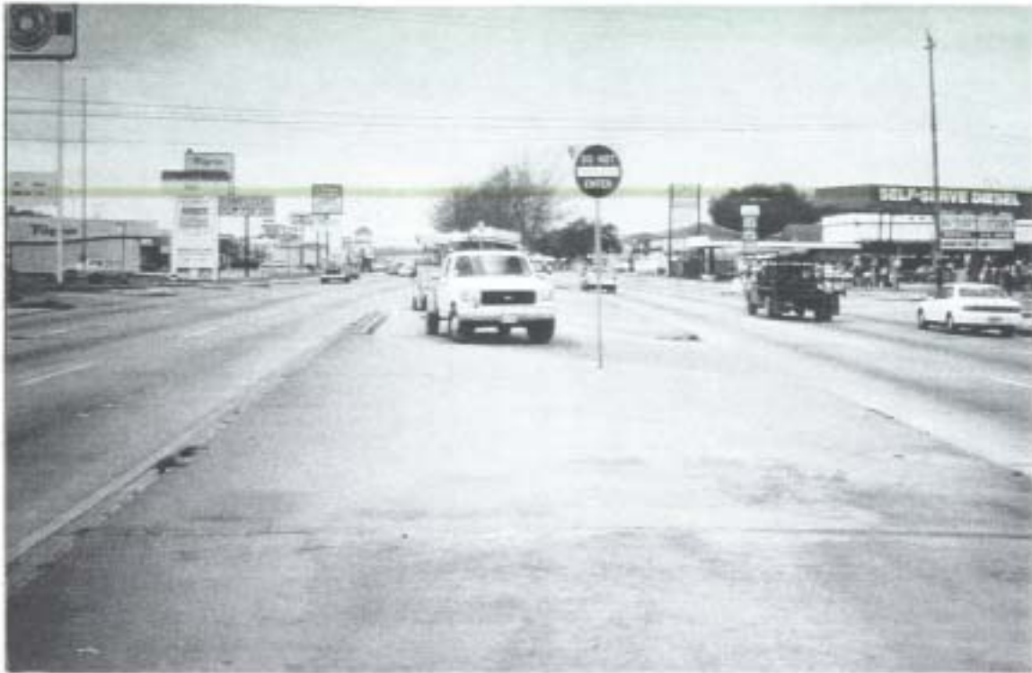
Figure 2-5. Southbound South Post Oak Road at the Northern End of the Project Limit.
