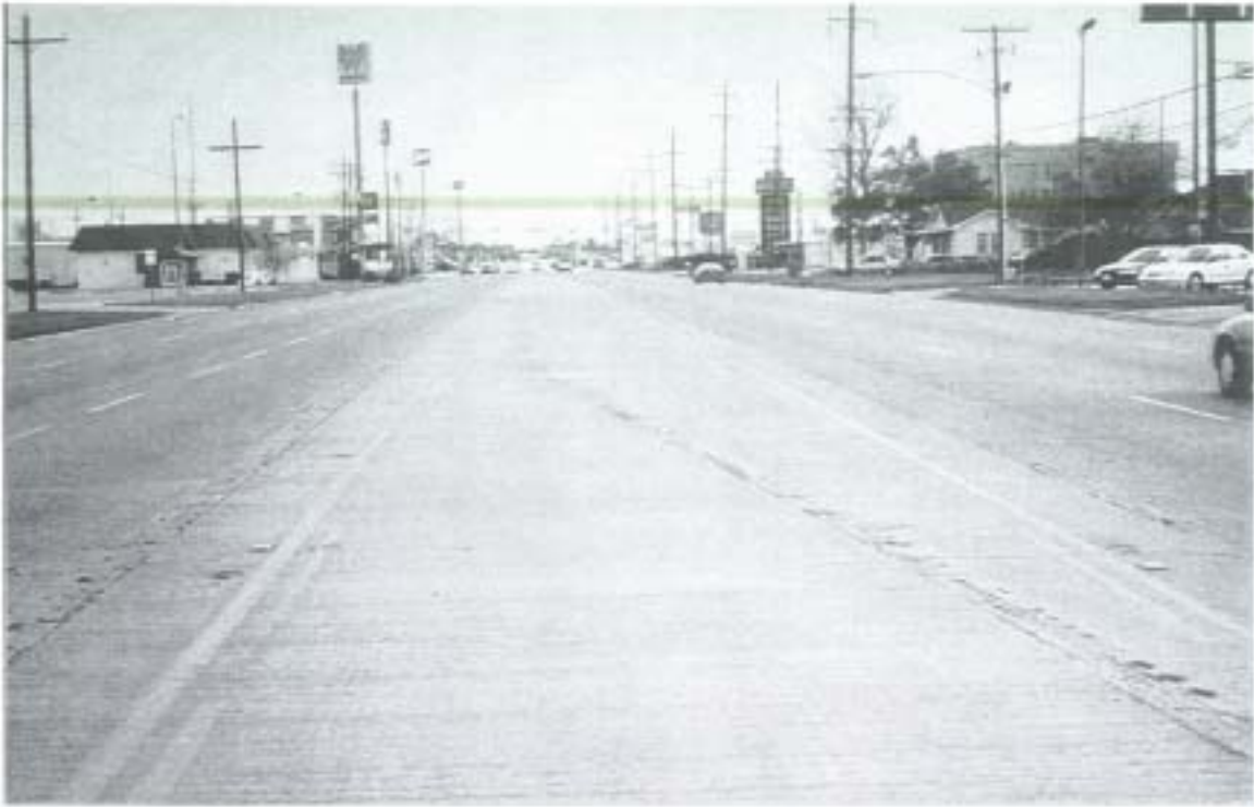
Figure 2-19. Southbound Twin Cities Highway North of Texas 73.
