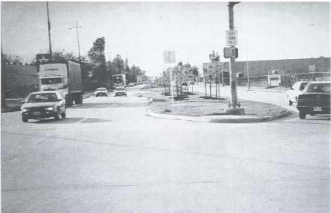
Figure 2-10. Westbound Clay Road at Hollister Road.
