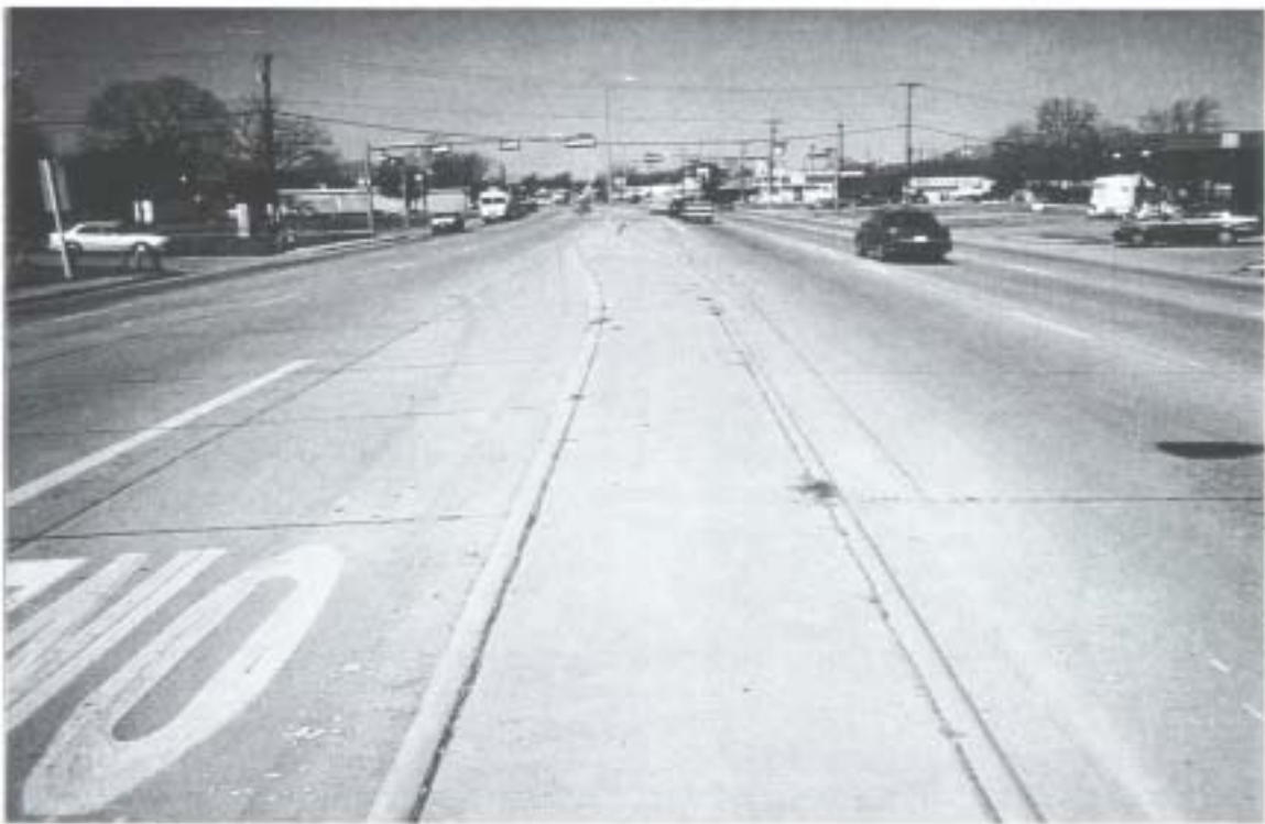
Figure 2-23. Westbound University Drive near Church Street.
