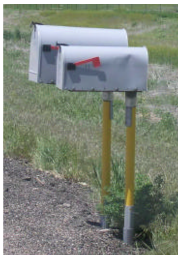
Figure 6. Damaged metal boxes on rigid post mounts. The post on the left is set at the edge of the pavement, while the two on the right are set about 8' from the edge of the shoulder with a small gravel turn-out to allow close access to the boxes.
