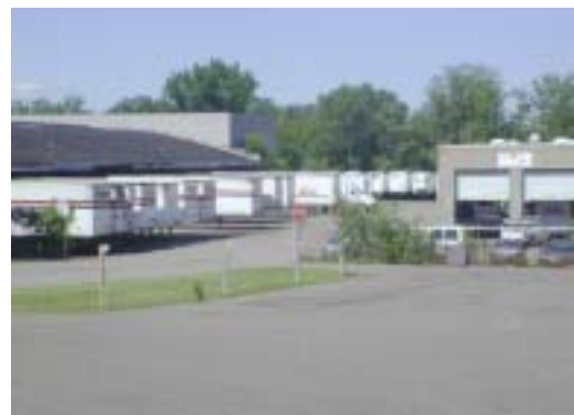
Figure 2.43. Most of the older industrial sites are paved and have minimal water retention strategies employed.
