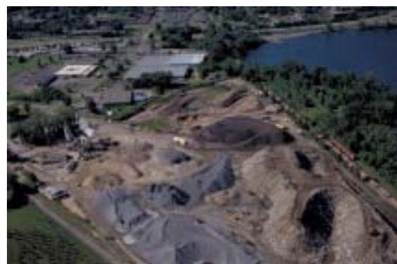
Figure 2.27. Asphalt plant in Northwest Quadrant.
