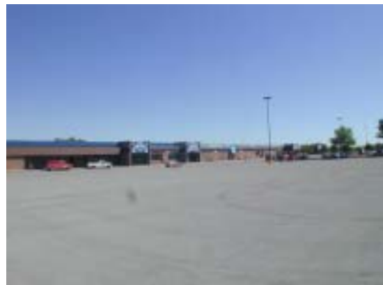
Figure 2.35. Surface parking lot in front of shopping center.
