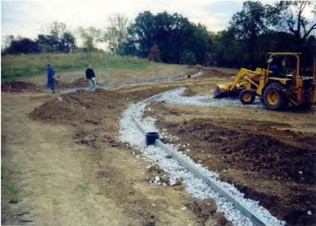
Figure 9.16 Installing a Level Spreader at Coffee Creek Center
