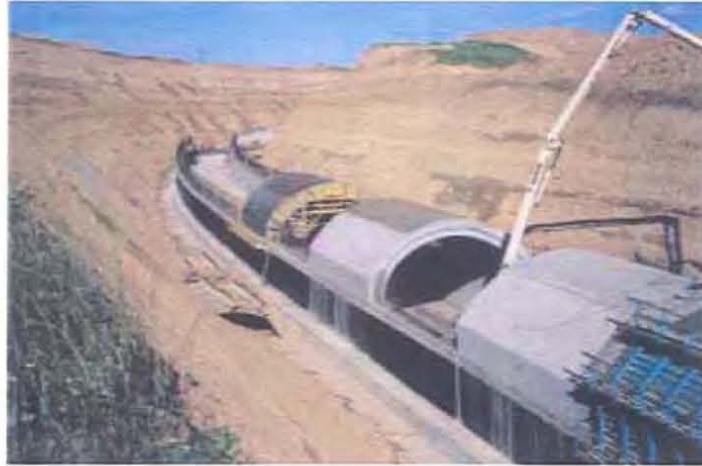
Concreting alternate sections of false tunnel roof.
