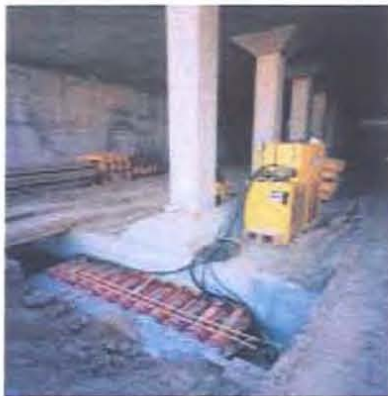
Box jacking arrangement to cross beneath RENFE tracks at F4 station.
