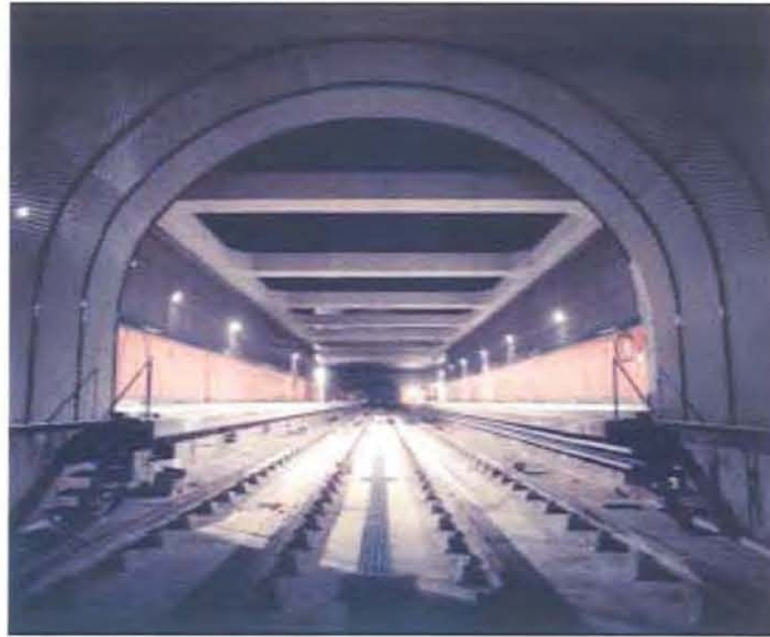
Internal view of El Casar station.
