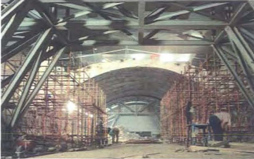
Cutting line 9 roof vault at Colombia station.
