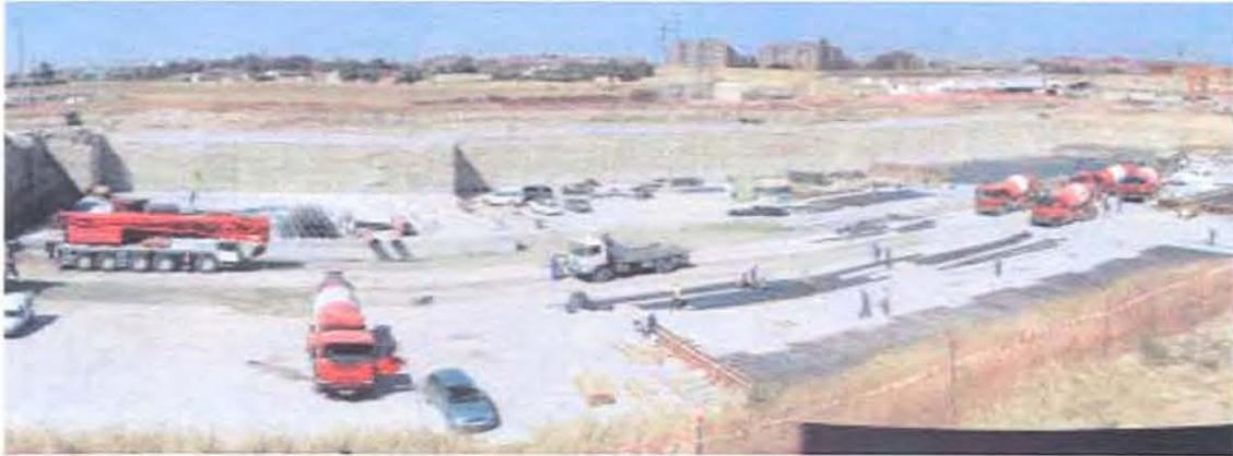
Panorama of open pit excavation of La Bercial station.
