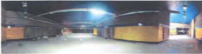
Loranca and Fuenlabrada Hospital stations nearing completion.
