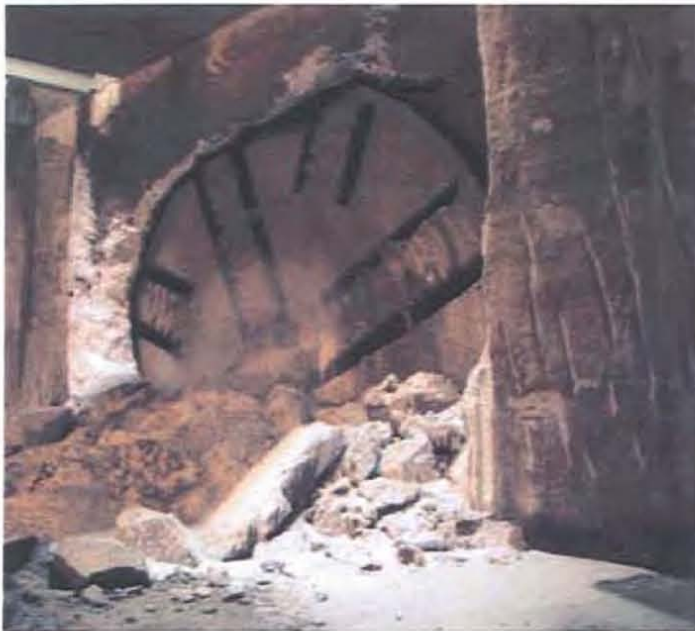
Mitsubishi NFM TBM arriving at Casa del Reloj station.
