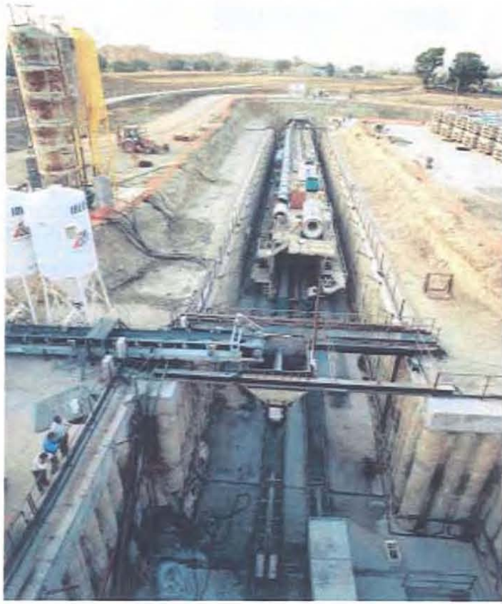
NFM TBM La Chata ready for launch outside Leganés.
