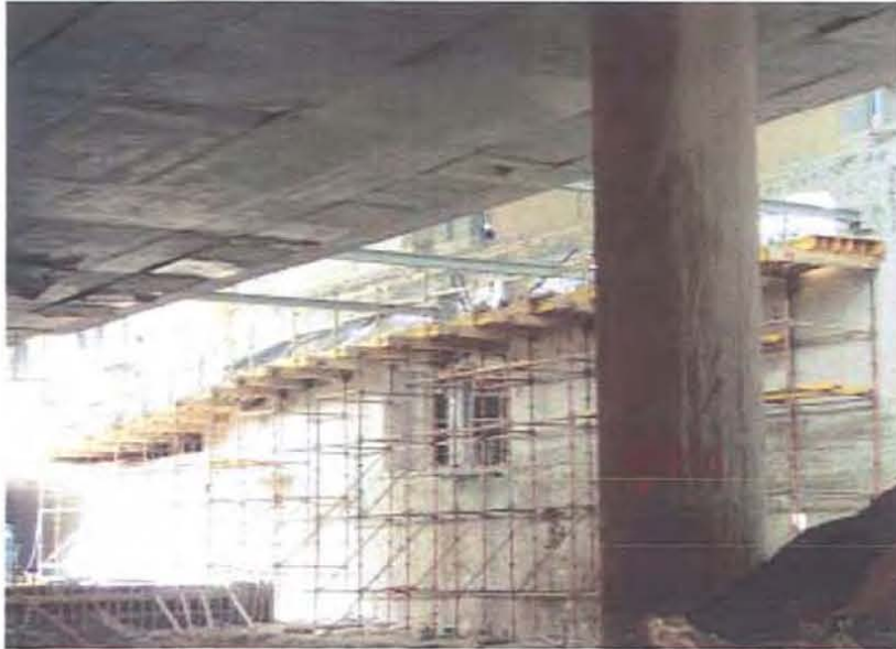
Voids for the passage of support and tying beams at Nuevos Ministerios arcade.
