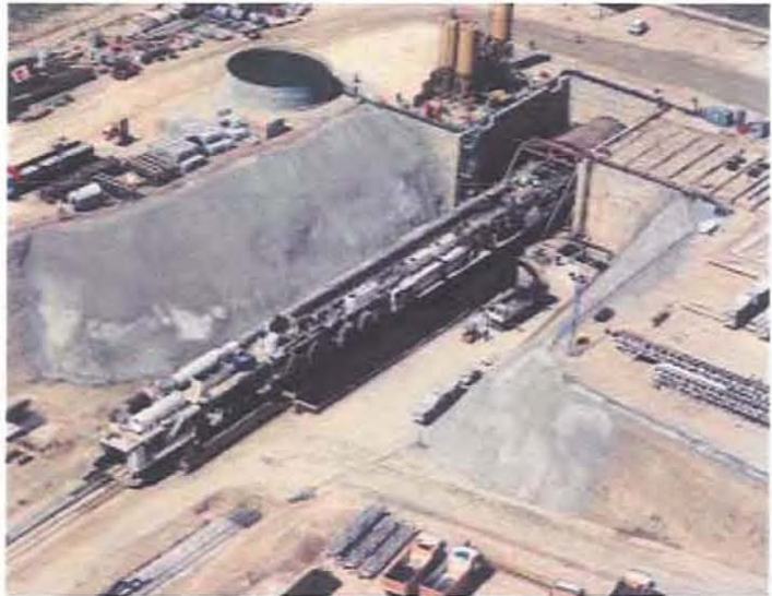
La Adelantada TBM launching at Manuela Malasana station.
