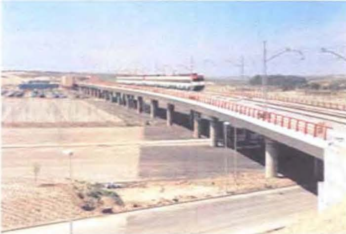
Theme park viaduct.
