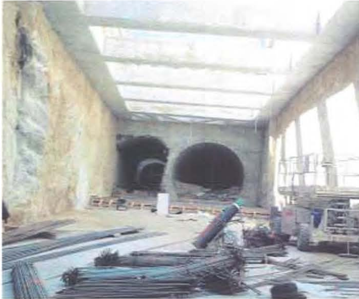
TBM removal point outside Cuatro Vientos station.
