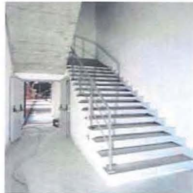
Emergency exit stairway.
