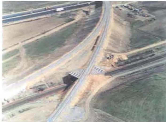
Flyover with embankments.
