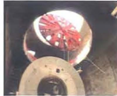
Lowering the cutterhead of the Herrenknecht TBM.
