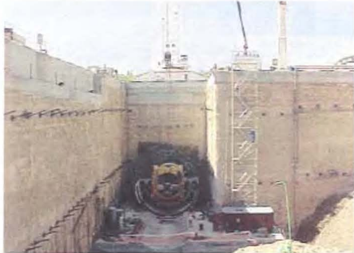
Building the TBM at Colonia Jardín station box.
