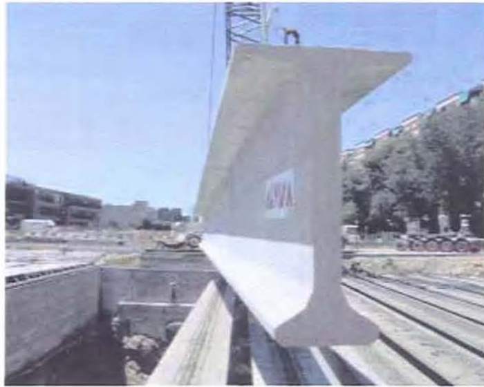
Placing the roof beams at a station.
