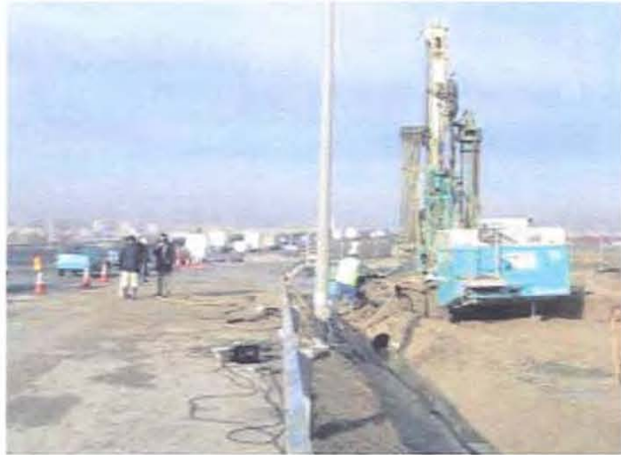
Cement injection on highway M-406.
