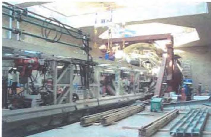
Assembling TBM for launch from shaft near Mar de Cristal station.
