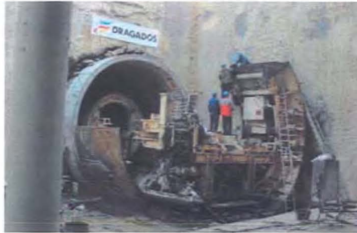
Final dismantling of Lovat TBM.
