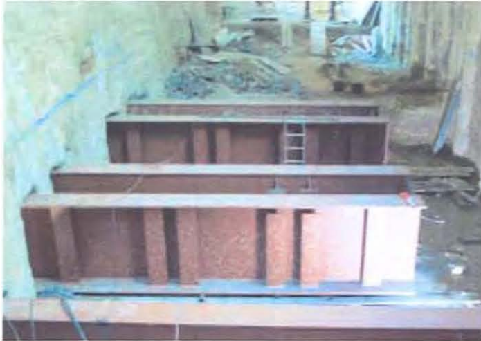
Supporting beams for the carpark slab.
