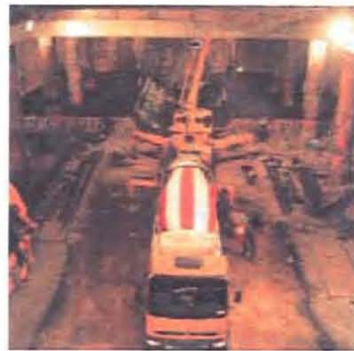
Preparation for arrival of TBM at Casa del Reloj station.
