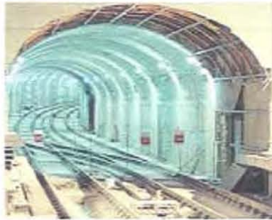
Traditional tunnel from Loranca station.
