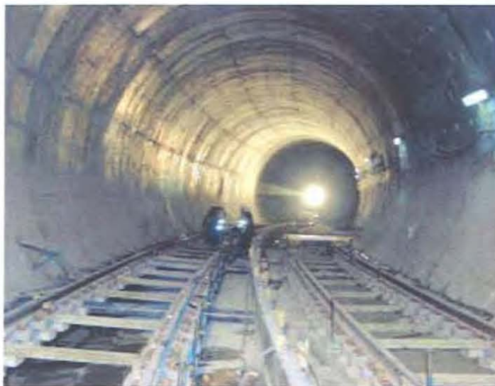
Tracklaying in the completed TBM tunnel.
