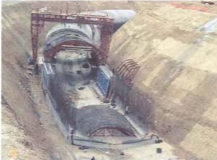
Open cut tunnel under construction.
