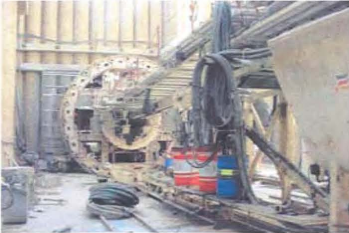
TBM assembly at telescope 2.
