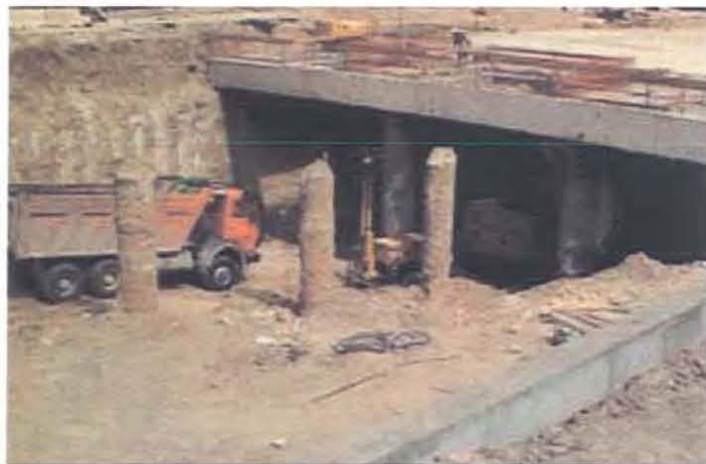
Excavation beneath the roof slab of Joaquín Vilumbrales station.
