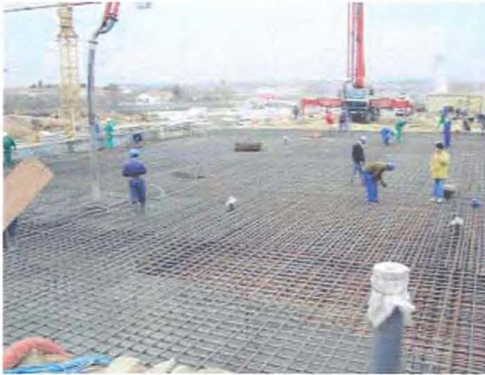
Laying the concourse roof at Colonia Jardín.
