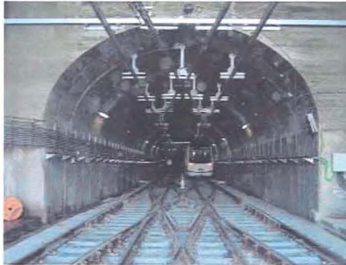
Access tunnel portal.
