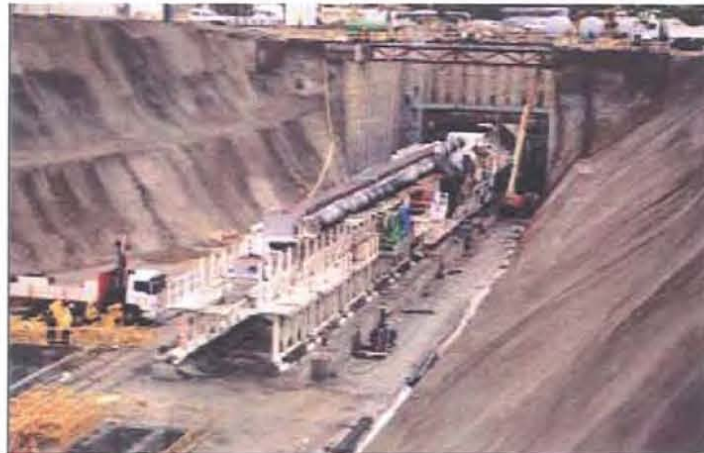
Launch pit for Herrenknecht TBM at El Bercial.
