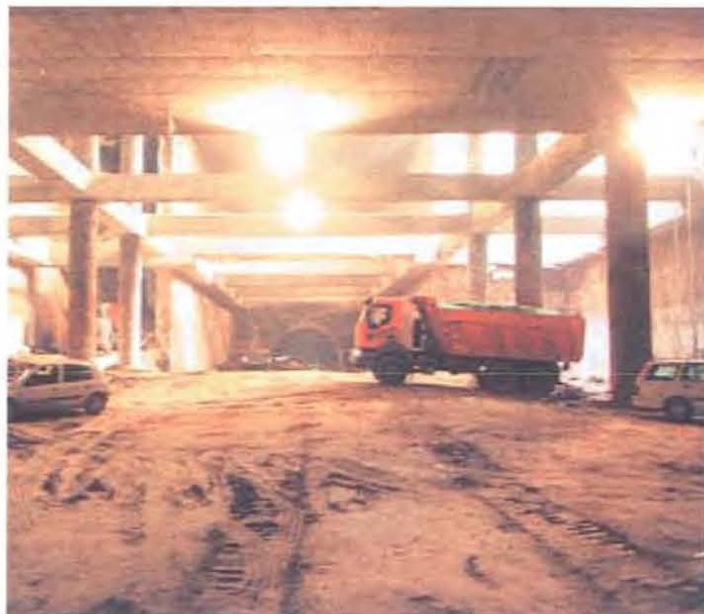
Julián Besteiro station under excavation.
