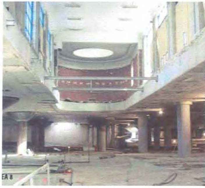
Final stages of construction of Nuevos Ministerios arcade, following successful underpinning.
