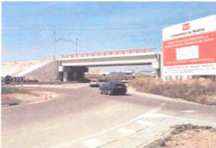
Overpass at the M-301 road.
