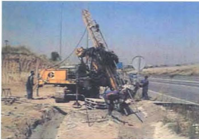
Jet grouting columns alongside M-40 motorway.
