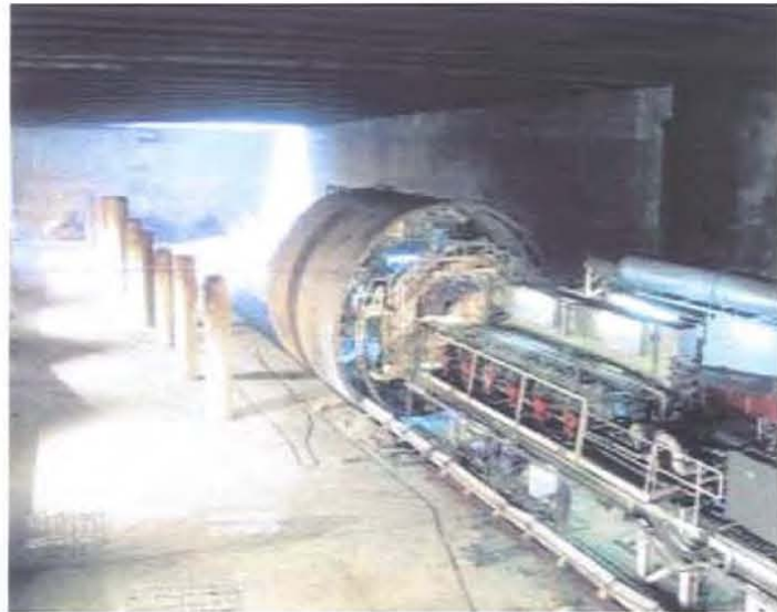
TBM transit through station box.
