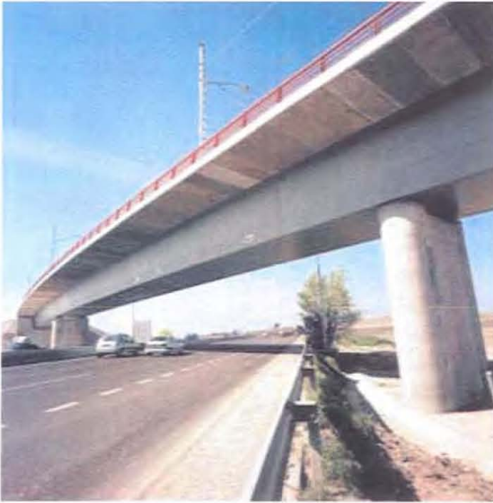
Viaduct over the N-IV highway.
