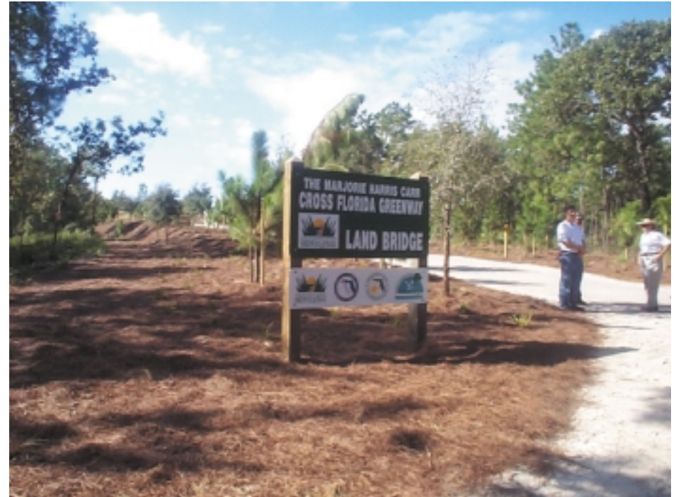
Eastern approach to the Land Bridge
