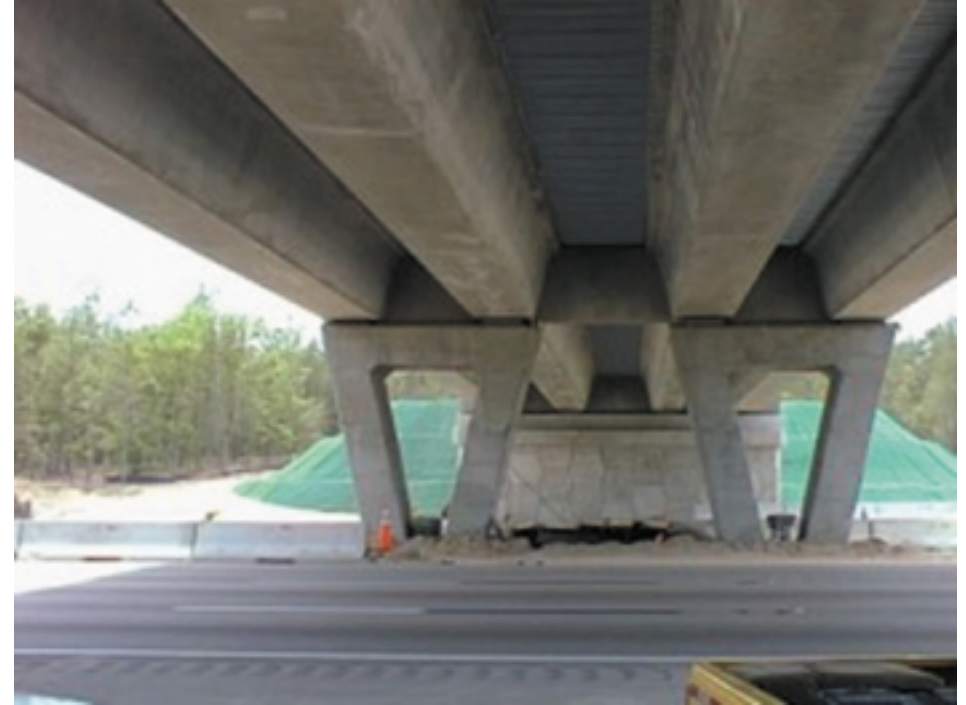
A view of the U-beams
