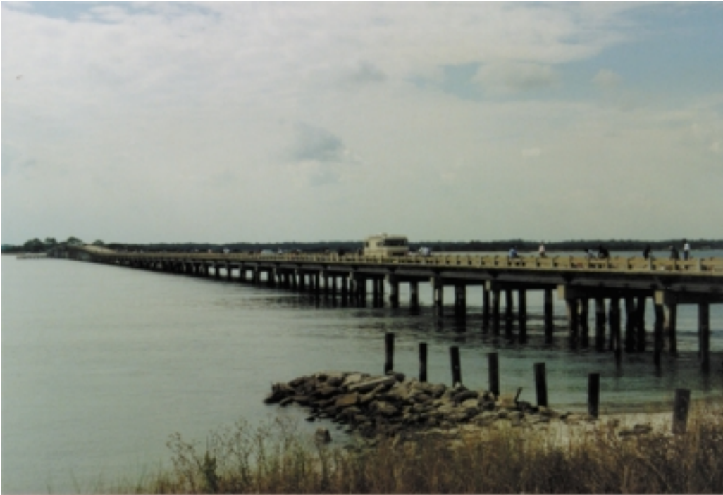
Before: The old bridge with fishers and traffic
