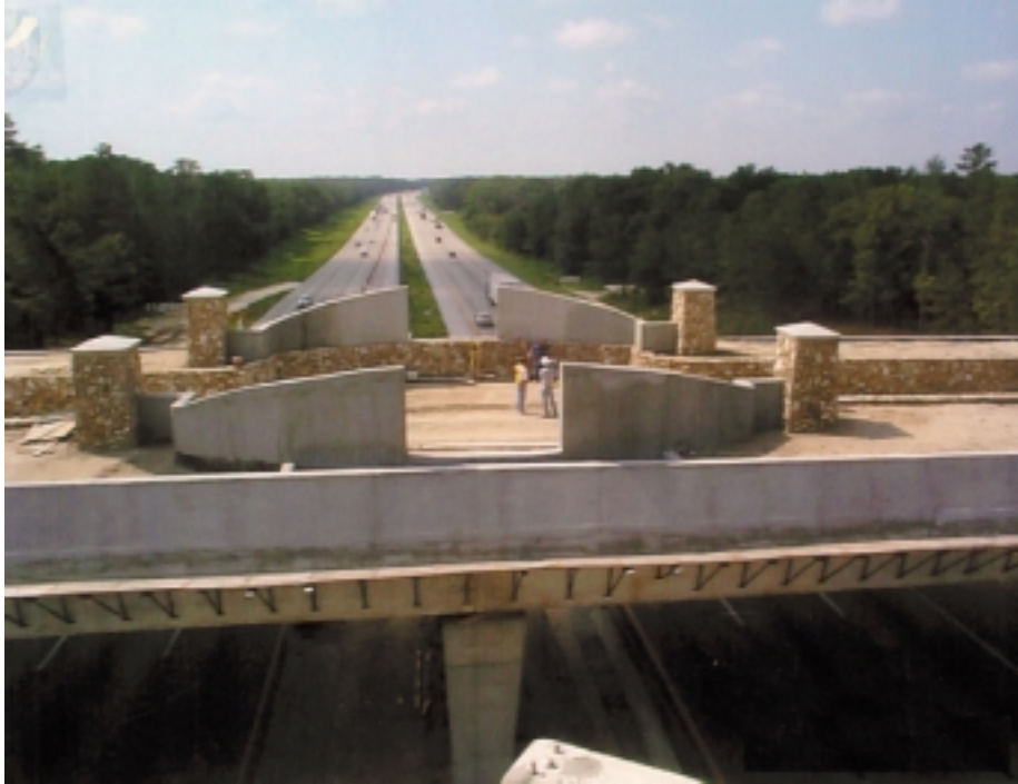
An aerial view of the bridge, while under, construction and I-75
