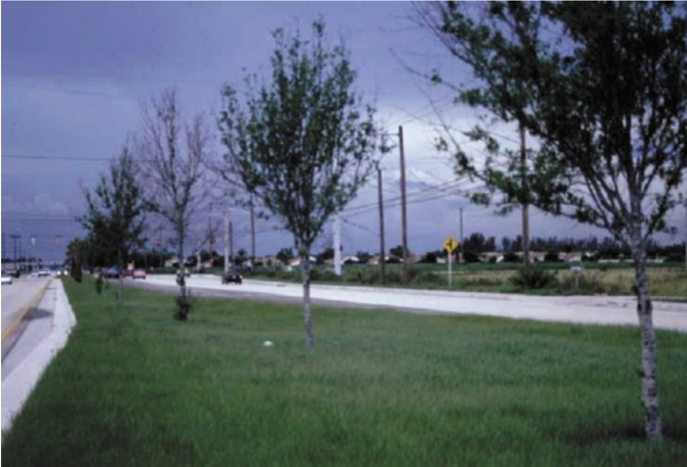
New landscaping along Broward Boulevard
