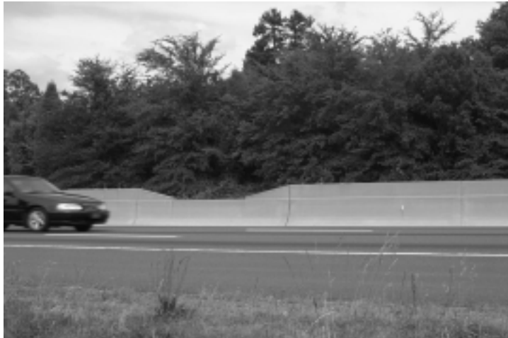
Figure 8-7. Concrete Barrier Opening in Charlotte, NC.
