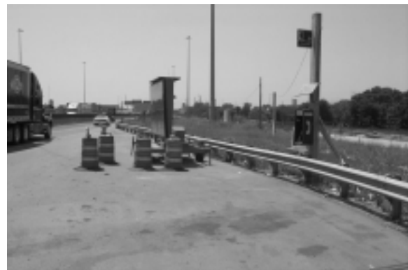
Figure 4-17. AIS in Construction Area.
