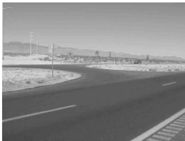
Figure 5-1. Shoulders with Rumble Strips.
