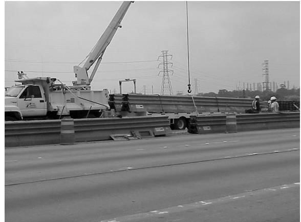
Figure 3-10. EA BarrierGate Installation.
