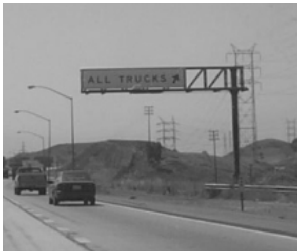
Figure 9-8. Exit Sign for Truck Lane.
