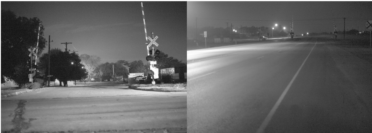
Figure 8. Railroad Grade Crossings with Visibility Affected by Roadway Illumination.
