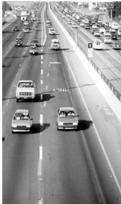
Figure 5. Entry/Exit for Concurrent-Flow HOV Lane in Southern California (2).
