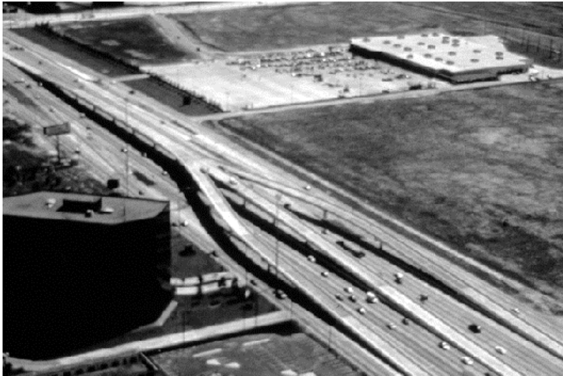
Figure 12. IH-45 North Freeway Y Ramp or Wishbone Ramp in Houston, Texas (2).
