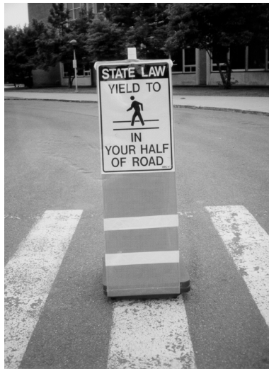
Figure 20. Supplemental Pedestrian Crossing Channelizing Device used in New York State. (Photo courtesy of Herman Huang, UNC Highway Safety Research Center)
