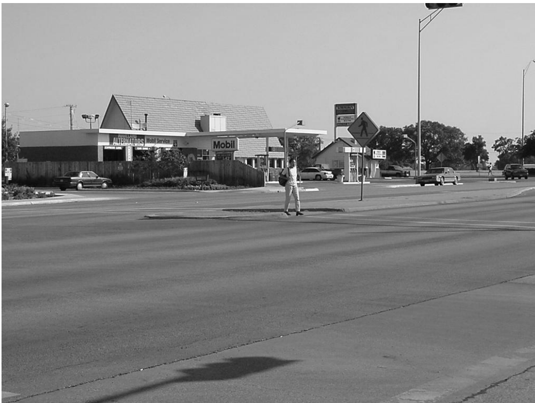
Figure 35. Use of Median Refuge Island on Eight-Lane Arterial Street – College Station, Texas.
