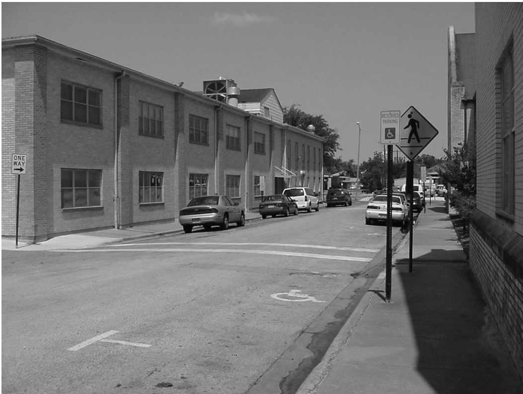
Figure 9. Basic Pedestrian Crossing with Crosswalk Sign and Markings.
