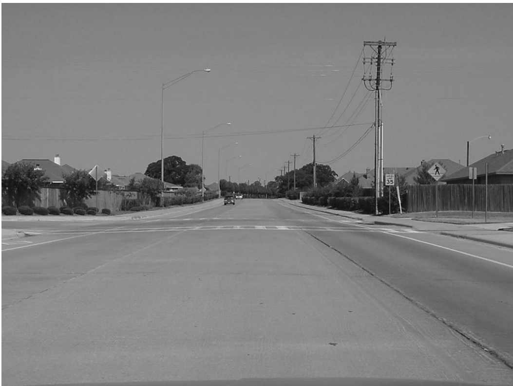
Figure 7. Mid-Block Marked Crosswalk on Straight, Wide Street with Inadequate Median Refuge.
