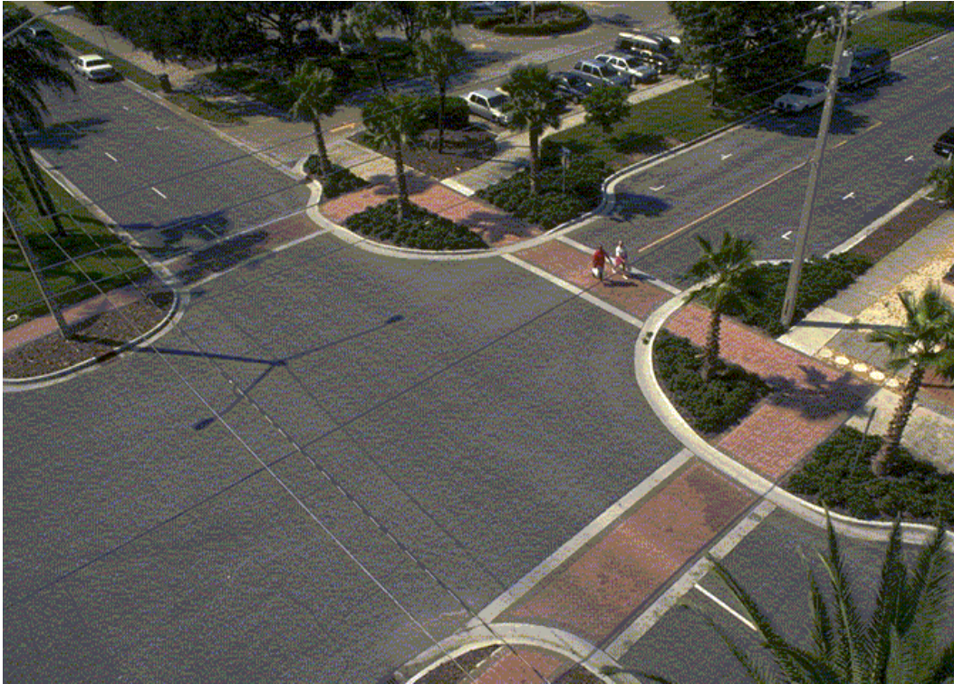
Figure 3. Use of Curb Extensions, Textured Crosswalks, and Median Refuge Islands. (Photo courtesy of Herman Huang, University of North Carolina (UNC) Highway Safety Research Center)
