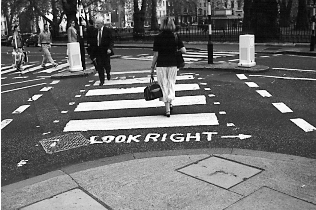
Figure 28. “LOOK RIGHT” Pavement Markings Used to Increase Awareness of Crossing Pedestrians – United Kingdom. (Photo courtesy of Gene Hawkins, Texas Transportation Institute)
