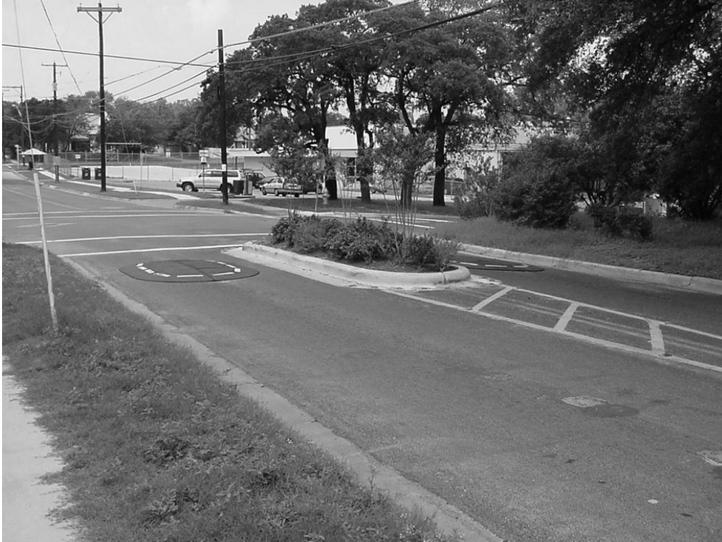
Figure 36. Center Island Narrowing with Speed Cushions – Austin, Texas.
