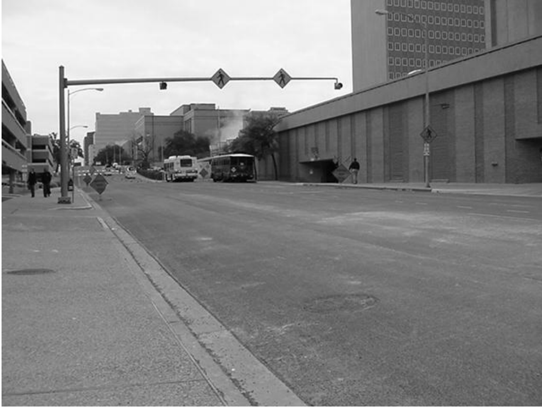
Figure 15. Use of Overhead Mast Arm and Flashing Beacons for Pedestrian Crossing Sign.
