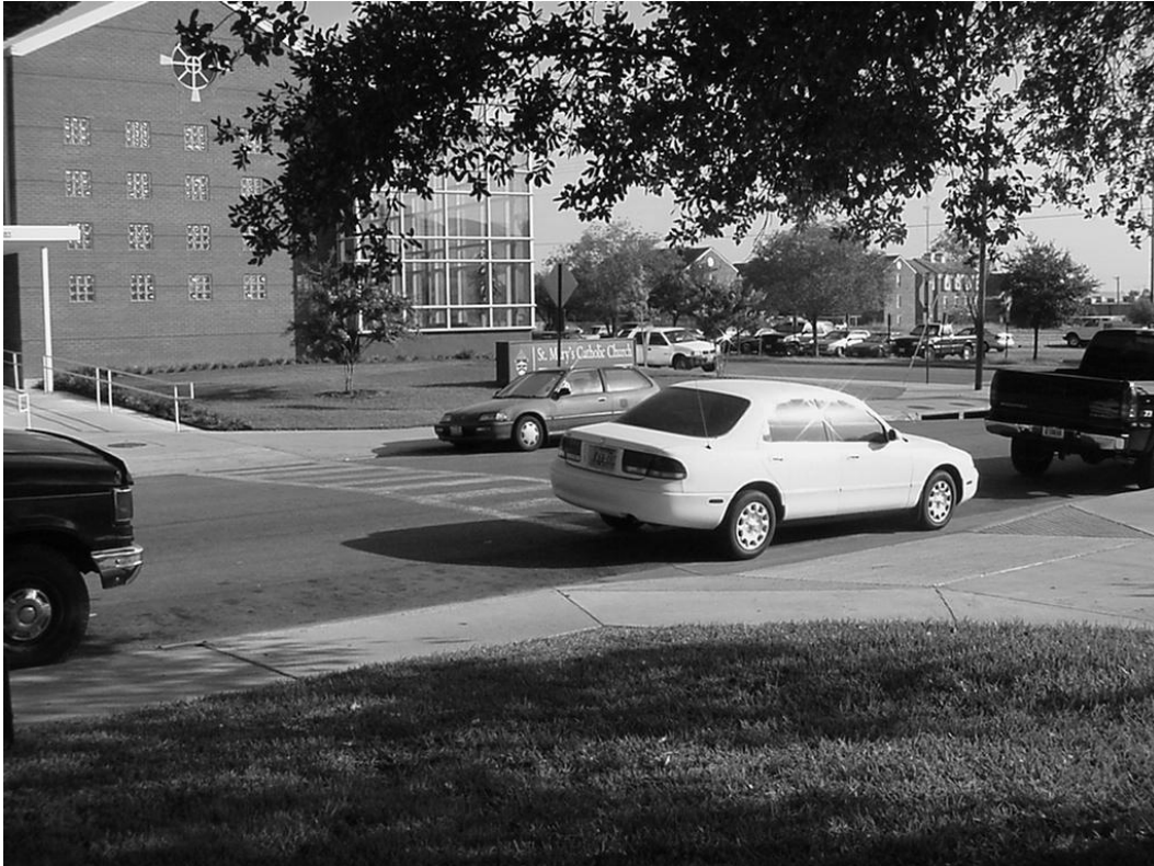
Figure 6. Mid-Block Crosswalk Blocked by On-Street Parking and within 200 Feet of Stop-Controlled Intersection.
