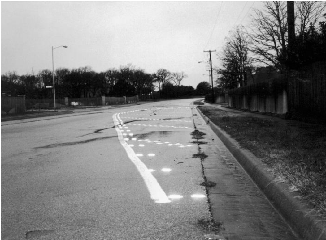
Figure 37. Roadway Narrowing Using Raised Pavement Markings – Arlington, Texas (24).
