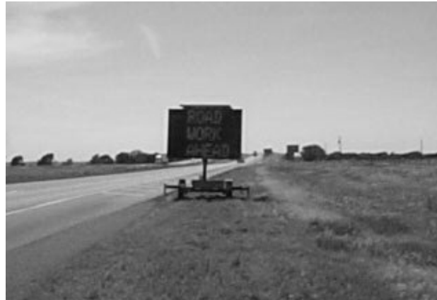
Portable Variable Message Sign.
