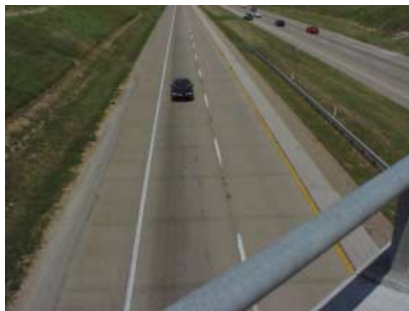
Figure 15. US 67 at Pleasant Run Road (southbound lanes).
