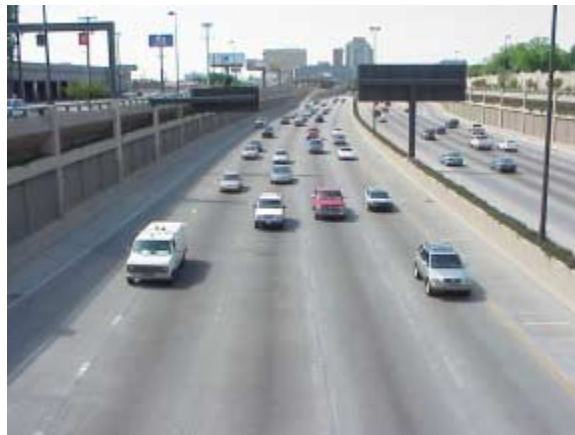
Figure 21. Site C – US 75 at Southwestern Blvd (northbound lanes).
