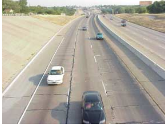
Figure 33. I-35E at Kirnwood Drive (southbound lanes).
