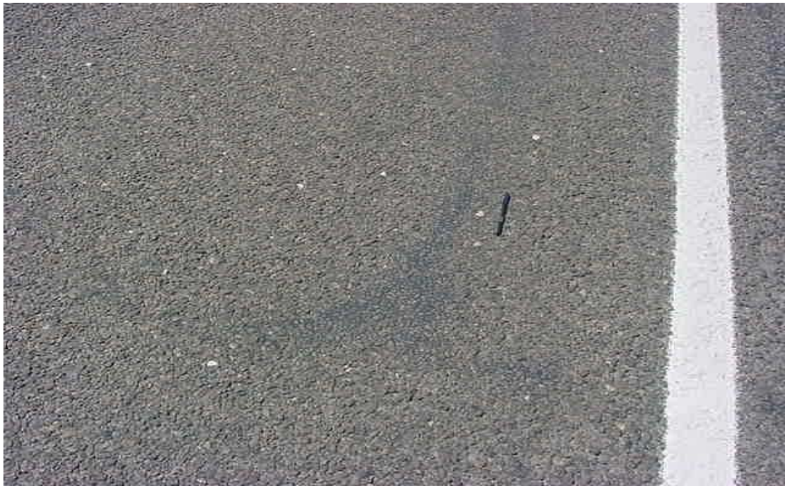
Figure 4.13 Lufkin, H3-covered test section during the August 20, 2002 investigation visit
