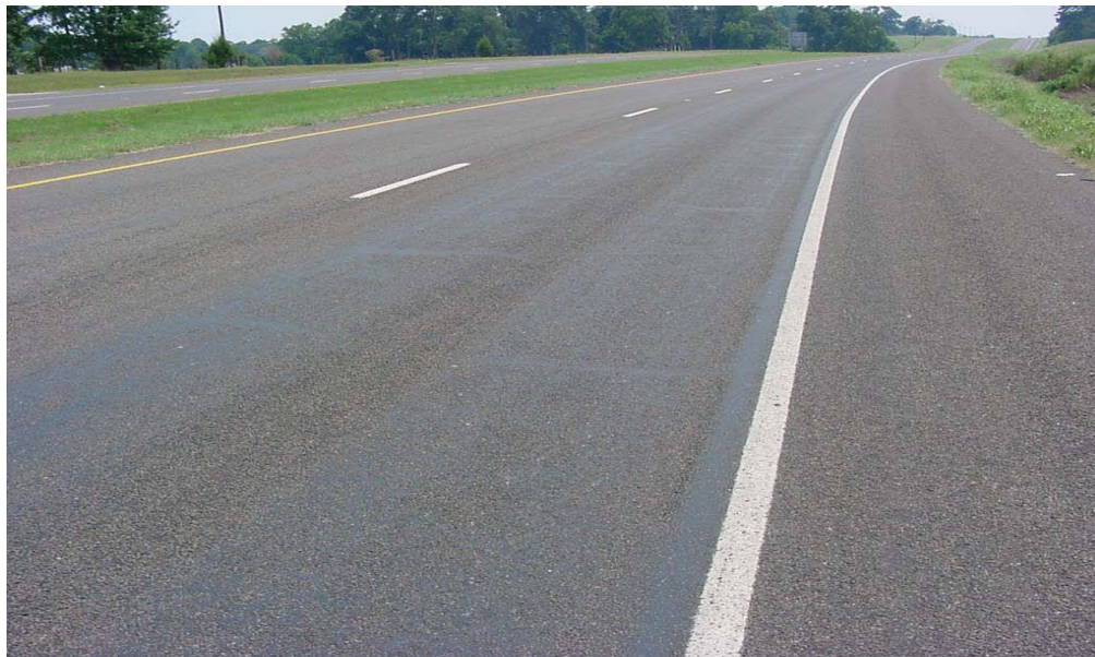
Figure 4.6 Atlanta, H1-covered test section during the August 8, 2002 investigation visit
