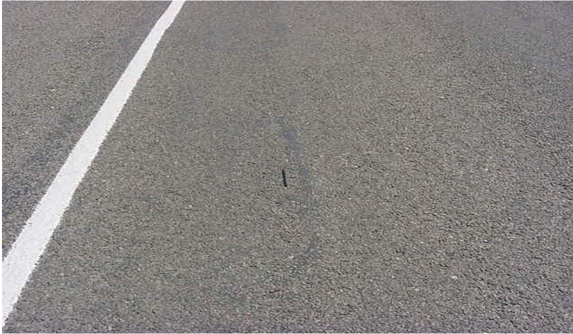
Figure 4.12 Lufkin, H1-covered test section during the August 20, 2002 investigation visit
