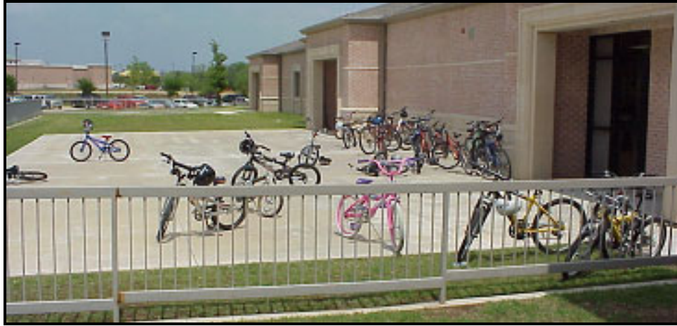
Figure 40. Fenced Concrete Pad Adjacent to School Building for Bicycle Storage.
