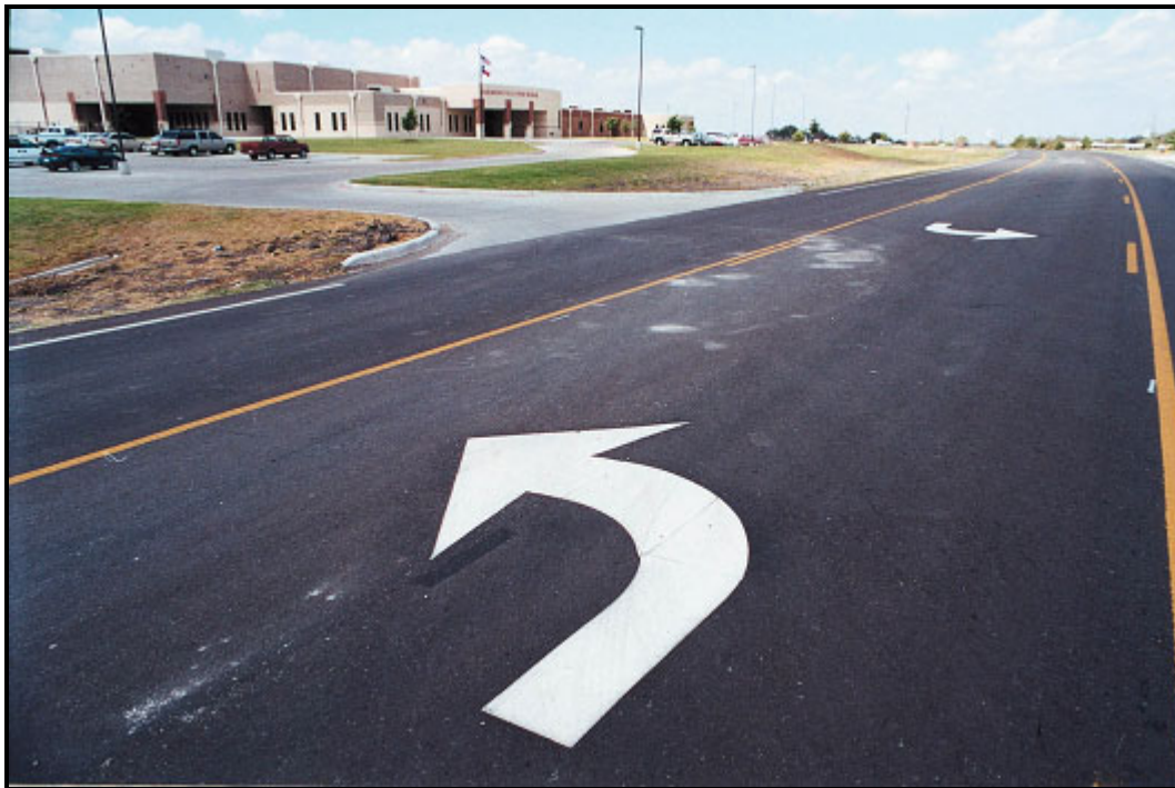
Figure 47. Newly Installed Left-Turn Lane in Front of an Elementary School.
