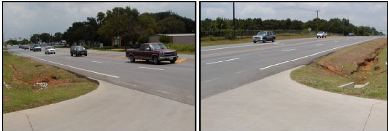
Figure 7. Good Example of School Driveway with Good Sight Distance in Both Directions.
