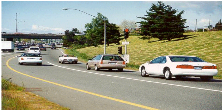
Figure 9. Example of Ramp Metering
