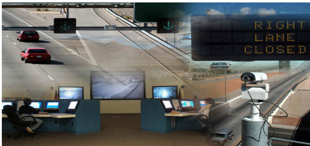
Figure 16. ITS Capabilities in El Paso Which Could be Applied to Planned Special Events – Overhead Lane Control, TMC, CCTV, and DMS (11)
