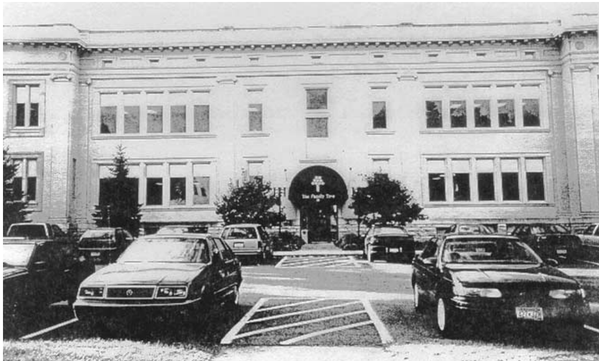
A social service agency, "The Family Tree," reuses the Richard Gordon School building.
