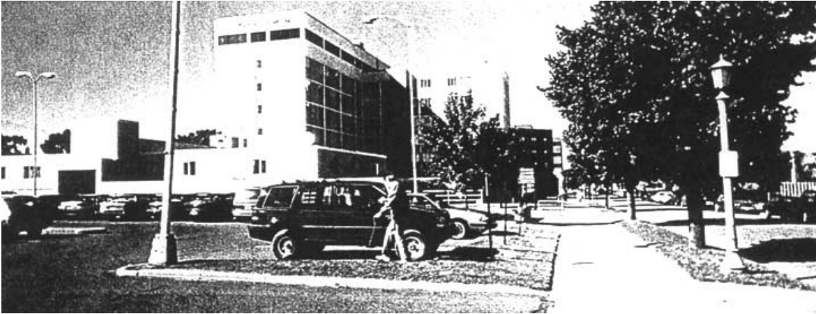
Current conditions of the former Midway Hospital, now HealthEast medical office building.
