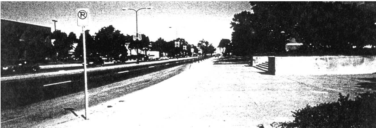
Potential transit stop on Snelling Avenue at Hamline campus and Hancock school.
