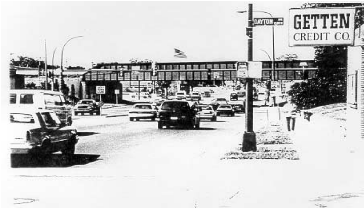
View looking north on Snelling at Marshall Avenue viaduct. Transit rider walking south to reach Selby shelter.
