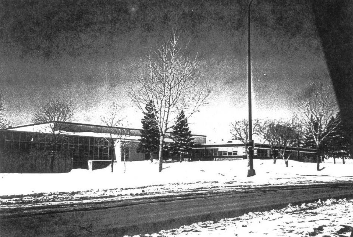
Existing conditions near potential transit stop at Highland Park High and Junior High School.
