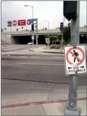
At 37 th Street and Hope Street facing west, showing the prohibited pedestrian crossing
