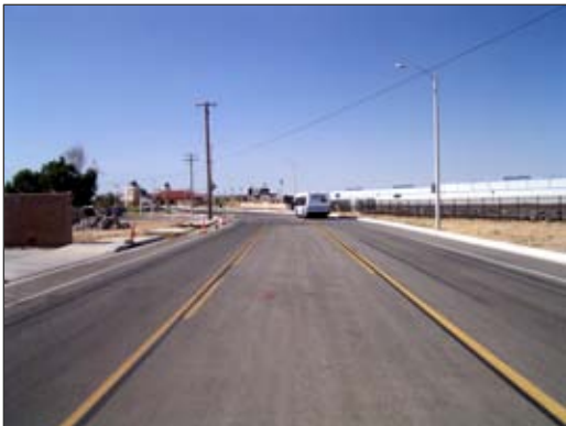
6 th Street East, facing north
