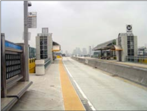
Harborway Transit Center at freeway grade
