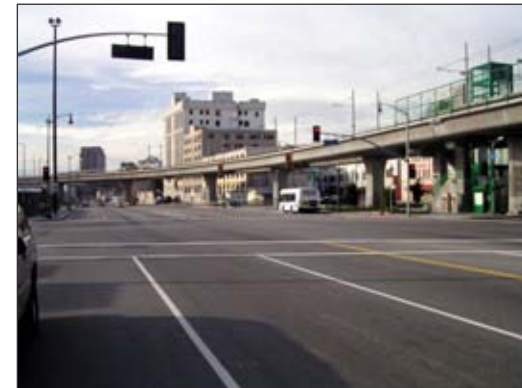
Alameda Street facing south across College Avenue
