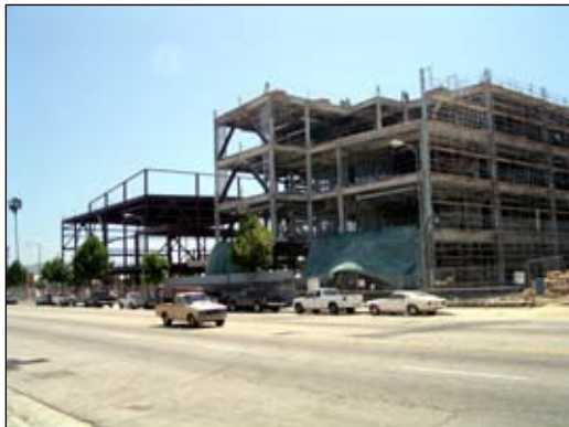
New High School on Vineland Avenue
