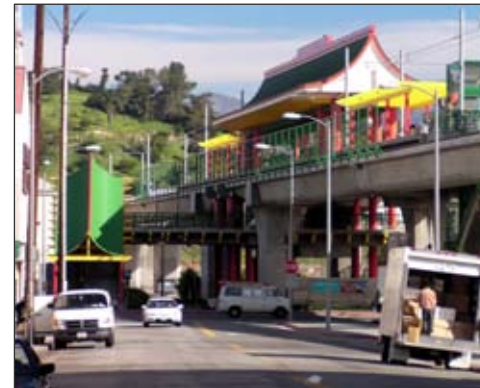
Spring Street facing north towards station
