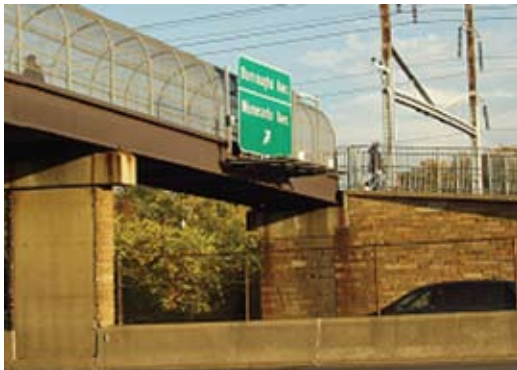
This grade-separated crossing over a freeway allows pedestrians to cross from their neighborhood to a nearby transit station.
