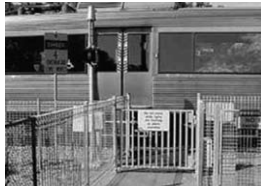
Multiple safety treatments are used at this pedestrian at-grade railroad crossing, including fencing, and warning signs.
