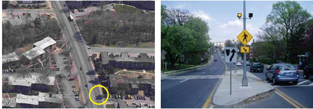
These pictures show a location where a median crossing island was installed to improve the safety of pedestrians accessing a well-used bus stop on a busy, high-speed roadway. The photo on the left was taken before and the photo on the right was taken after the improvement was made.
