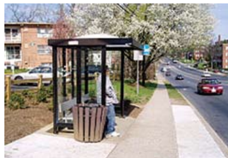
Enhancements to this bus stop include a shelter, bench, level landing pad, and an improved roadway crossing to increase pedestrian safety near the stop.
