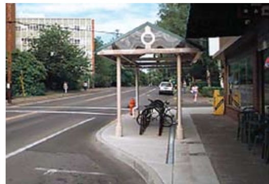
Curb extensions shorten pedestrian crossing distances by reducing the curb-to-curb distance across the roadway. They also add sidewalk space for transit stops, waiting areas, bicycle racks, or street furniture.
