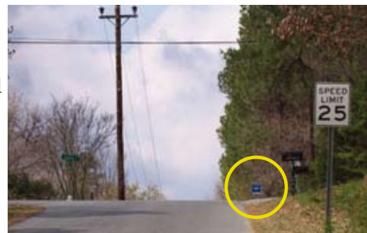
Pedestrians crossing the street to reach the bus stop circled in the photograph above will be hidden by the crest of the vertical curve.
