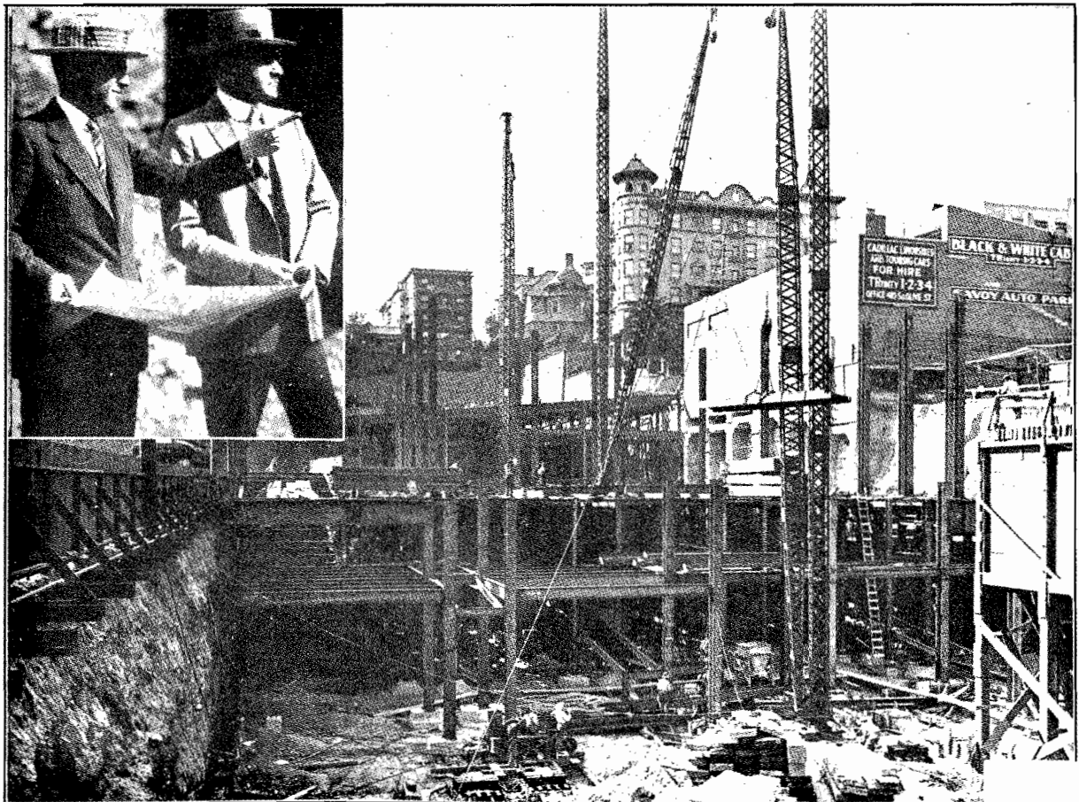
Structural steel workers are maintaining the same dizzy pace that has characterized the progress of other crews on terminal and tunnel project. Vice-President Pontius and Chief Engineer Johnson are seen on a tour of inspection.
