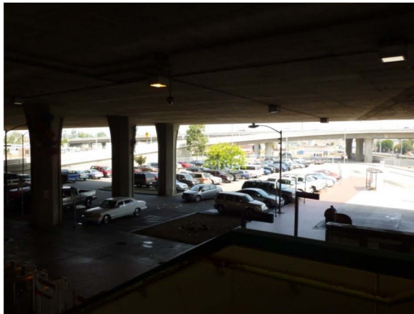
Figure 4-18. Northeast lot was 91% occupied during summer 2011.
