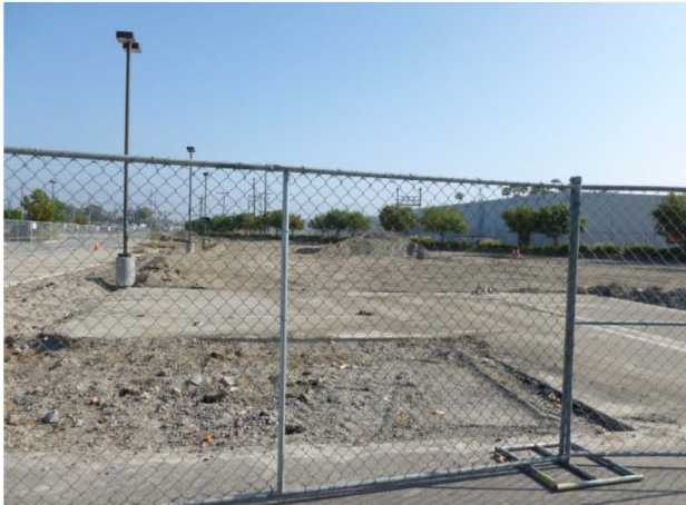
Figure 8-10. Half of the park and ride lot at Canoga Station has been closed off due to the extension of the Orange Line.
