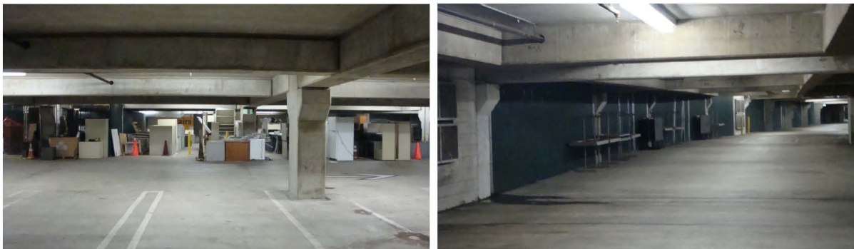
Figure 6-1 & Figure 6-2 show how several parking spaces (P4) are now used for storage, reducing the total parking capacity.
