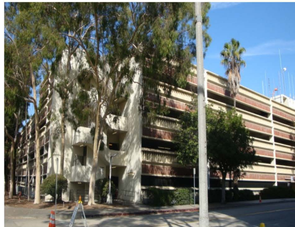
Figure 7-16. LA County parking structure at the corner of Ramona and Marengo (#2 on Table 7-11).
