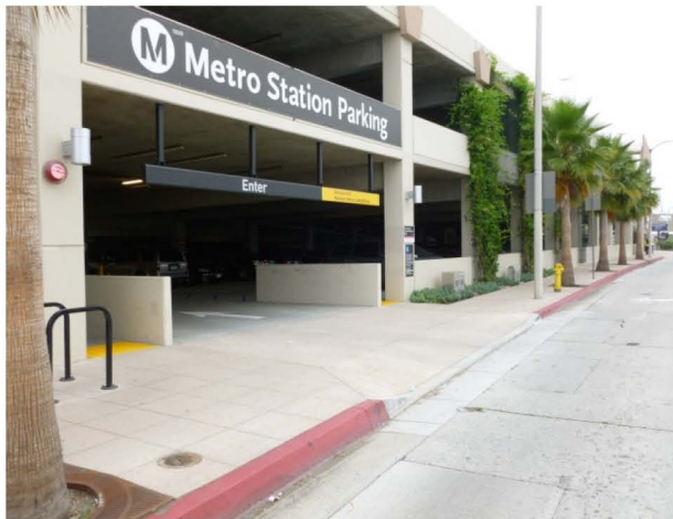
Figure 7-1. Parking structure entrance for the Atlantic Station.
