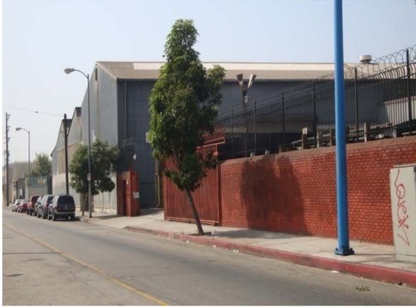
Figure 4-7. Surrounding uses to the station on Long Beach Blvd are predominantly industrial.
