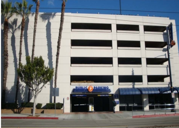
Figure 4-34. Public Parking on Pacific Ave (#1 on Table 4-18).
