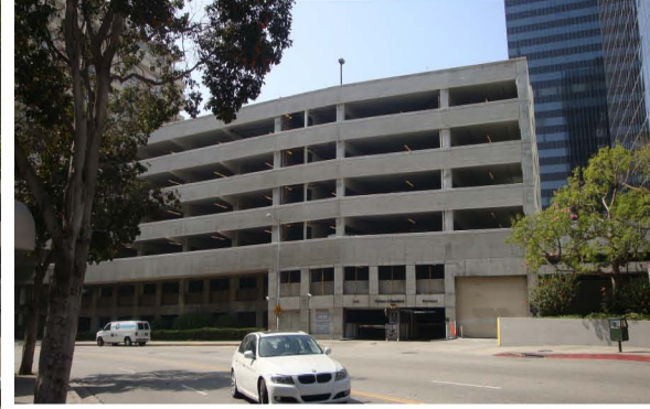
Figure 6-29 Public parking at Metroplex Wilshire
