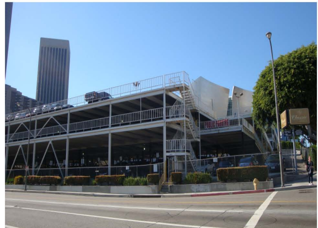
Figure 6-4 Public Parking structure on Olive. (#2 on Table 6-4)
