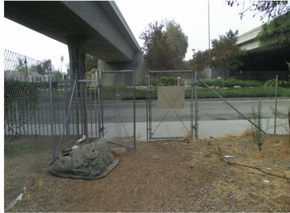
Figure 5-4. The lock on this fence has also been broken to access the station.
