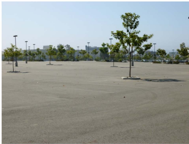
Figure 8-3. In 2011, utilization at the Sepulveda Station park and ride was 12%.
