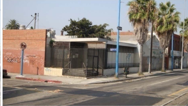
Figure 4-6. Connections to the station are unpleasant and inadequate.
