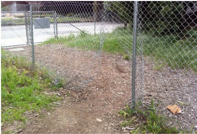
Figure 5-3. The chain link fence has been cut to access the station.
