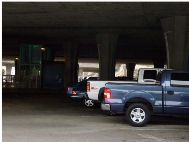
Figure 5-7. Portions underneath the freeway are dark and un-inviting.
