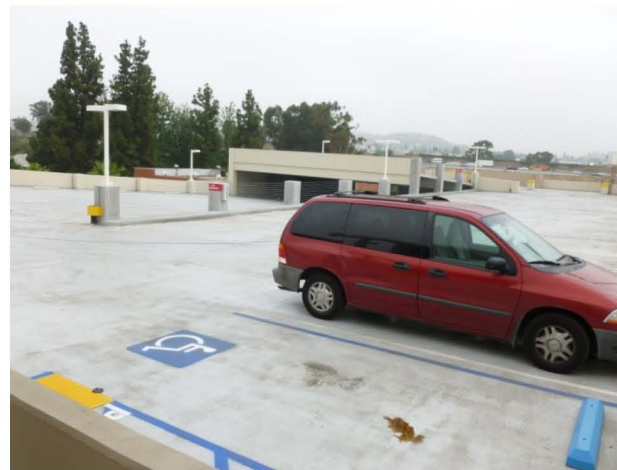
Figure 7-2. Rooftop level at the Atlantic Station Lot had a 53% occupancy rate in 2011.
