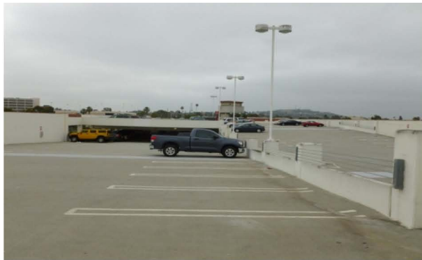
Figure 4-27. P4 Level of the parking structure at the Willow Station.
