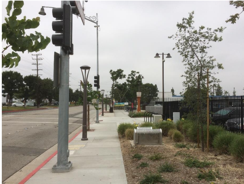
Photo 102: Sidewalk along Highland Ave. Connecting Parking to Station Platform
