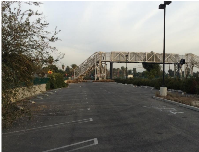
Photo 4: No Signage in Lot to Direct Riders to the Platform
