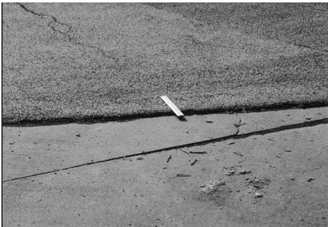
FIG. X1.45 Medium-Severity Shoving
