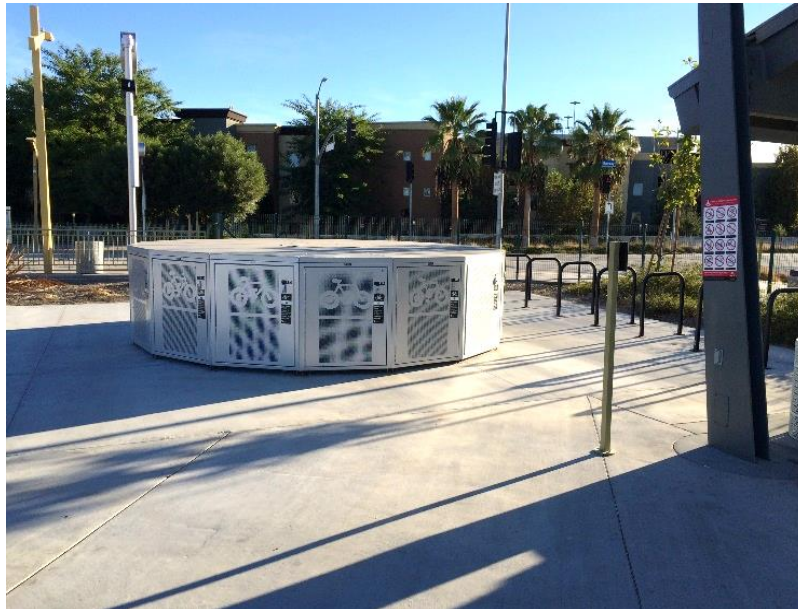
Photo 192: Bike Lockers and Racks
