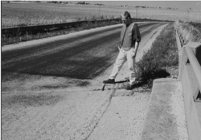
FIG. X1.44 Low-Severity Shoving
