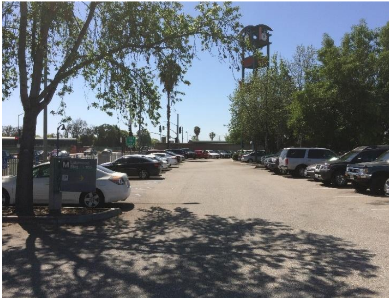
Photo 127: Faded Striping
