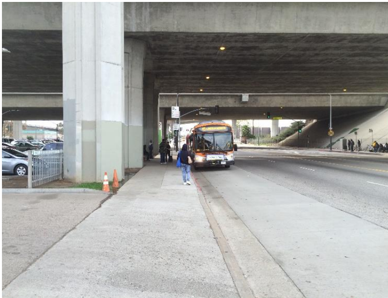
Photo 139: Sidewalk along Figueroa St.
