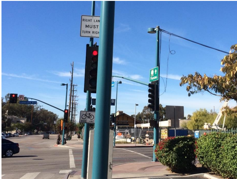
Photo 214: Wayfinding Sign on Lankershim Blvd.
