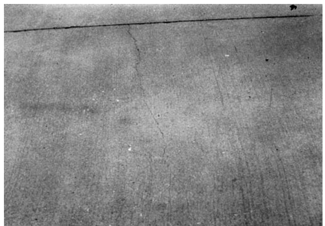
FIG. X2.44 Shrinkage Cracks
