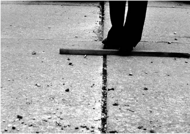
FIG. X2.13 Low-Severity Faulting
