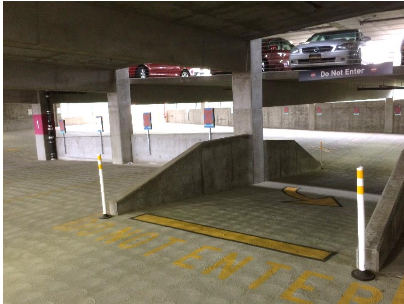
Photo 100: One-way Ramp Up from Lowest Level
