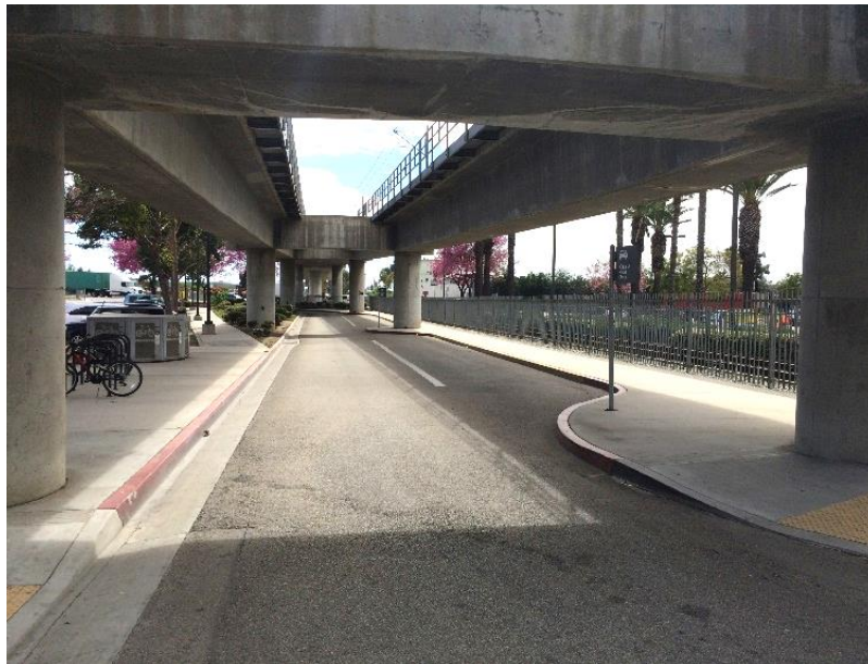
Photo 15: Bicycle Parking Underneath the Station Platform Area
