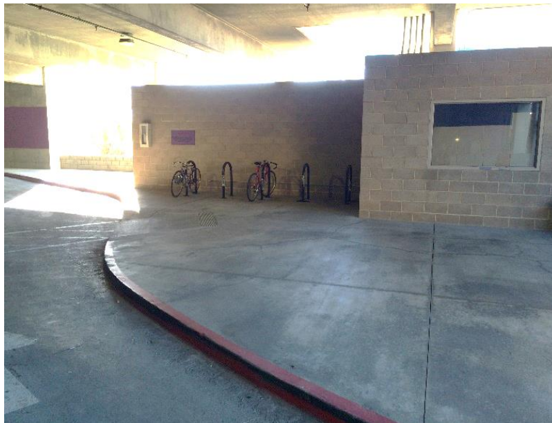
Photo 88: Difficult to Find Bike Racks
