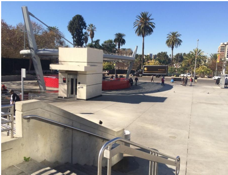
Photo 215: Plaza Area outside Station Portal
