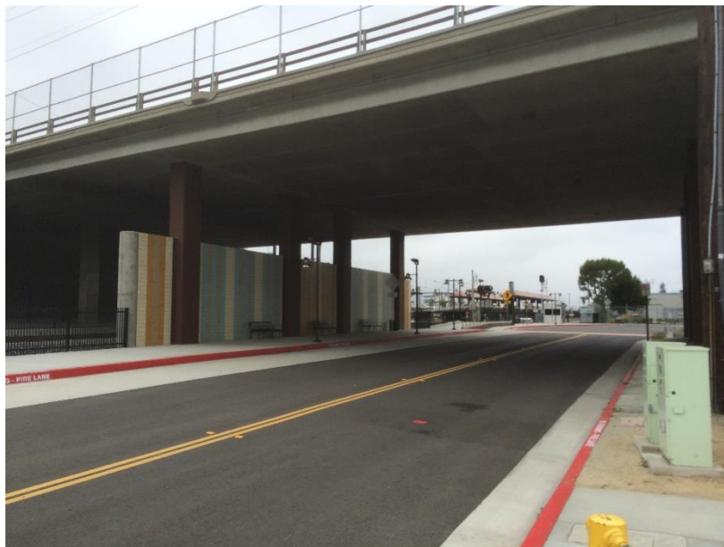
Photo 107: Sidewalk on North Side of Avenida Padilla
