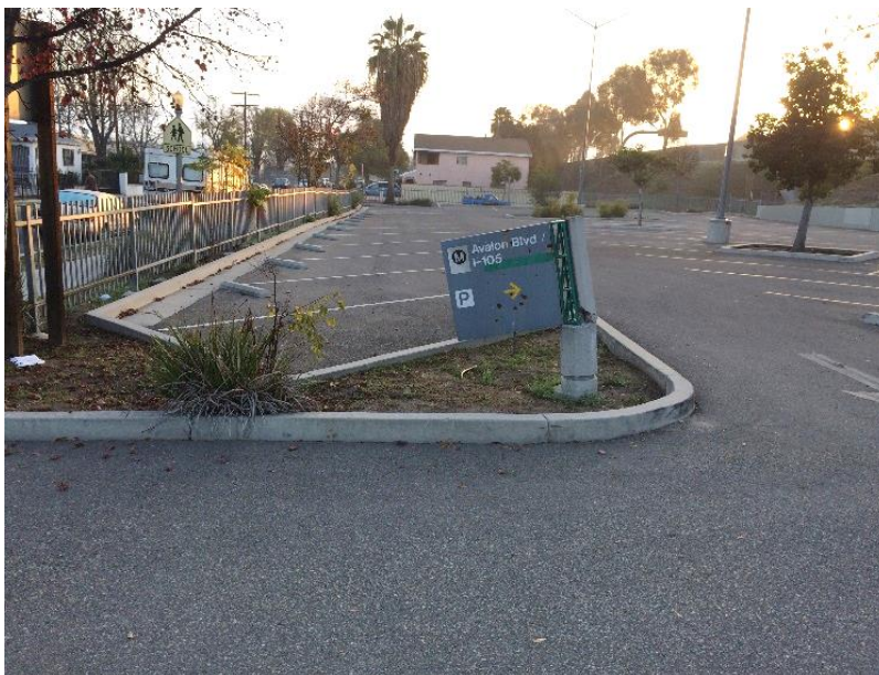
Photo 137: Broken Sign at Northeast Entrance to Lot
