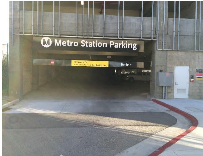
Photo 34: Parking Entrance Signage
