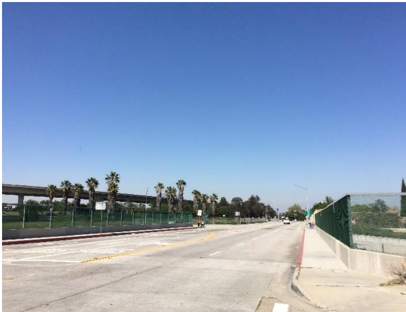
Photo 119: Sidewalk along Hoxie Ave.
