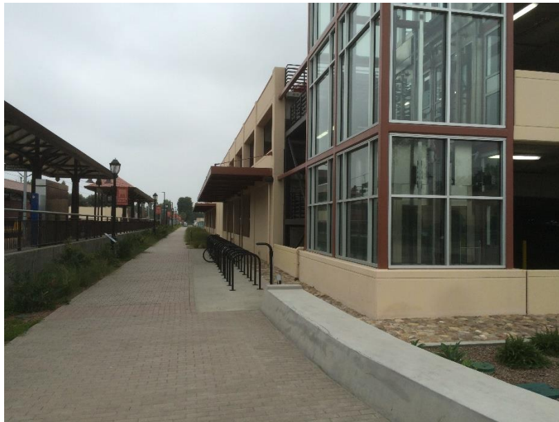
Photo 96: Bicycle Racks between Structure and Platform
