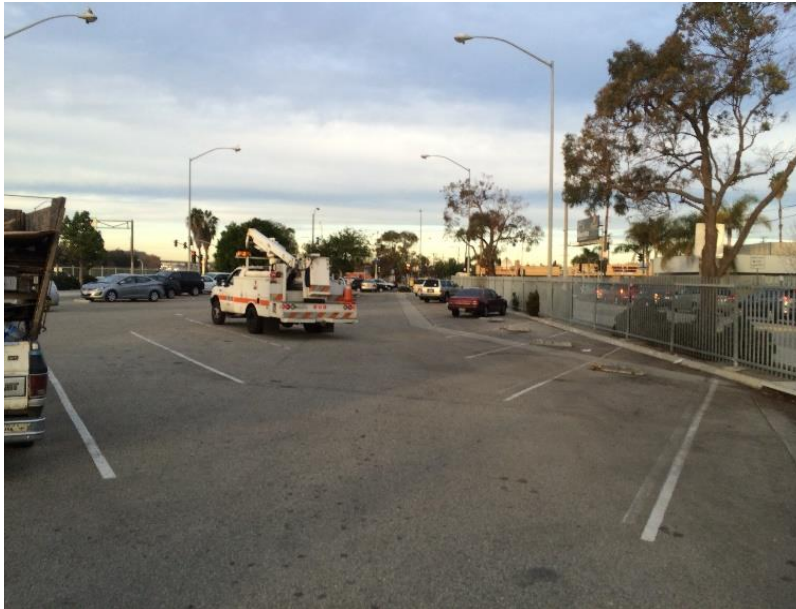
Photo 154: Faded Striping
