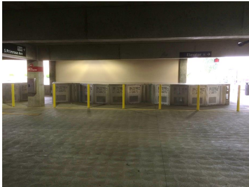
Photo 97: Bicycle Lockers inside Structure
