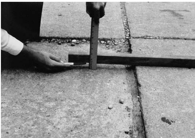
FIG. X2.15 High-Severity Faulting
