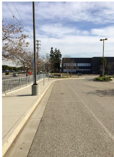
Photo 161: Sidewalks inside Station Parking Lot
