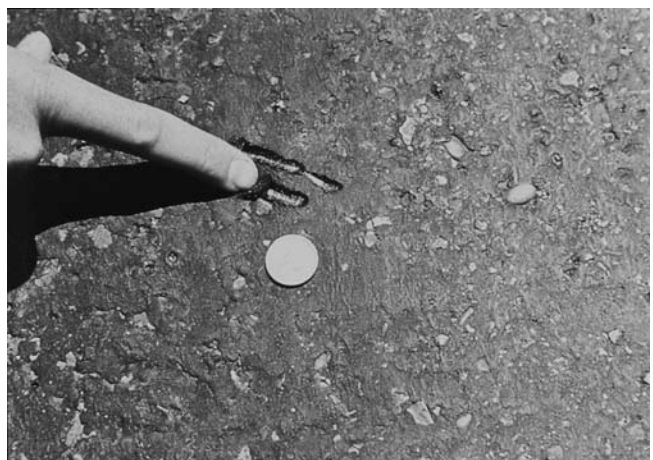
FIG. X1.5 Medium-Severity Bleeding
