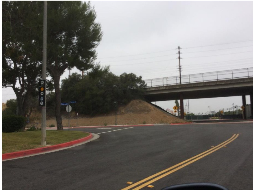
Photo 108: Signage along Avenida Padilla Directing to Platform and Parking
