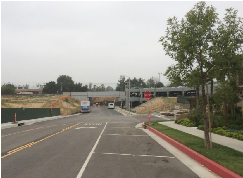
Photo 115: View along Citrus Ave. of Parking Garage
