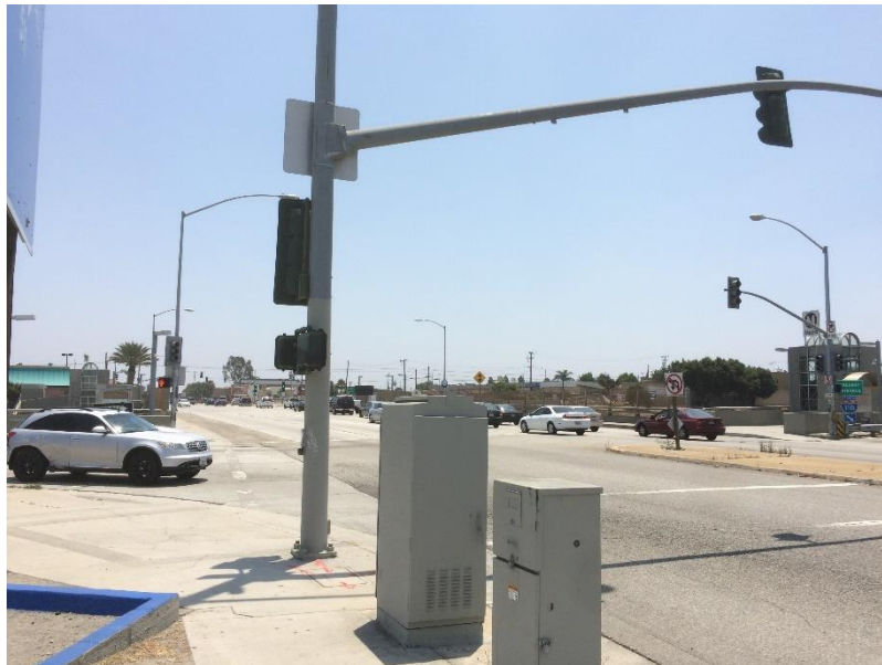
Photo 235: Intersection of I-110 and Carson St.
