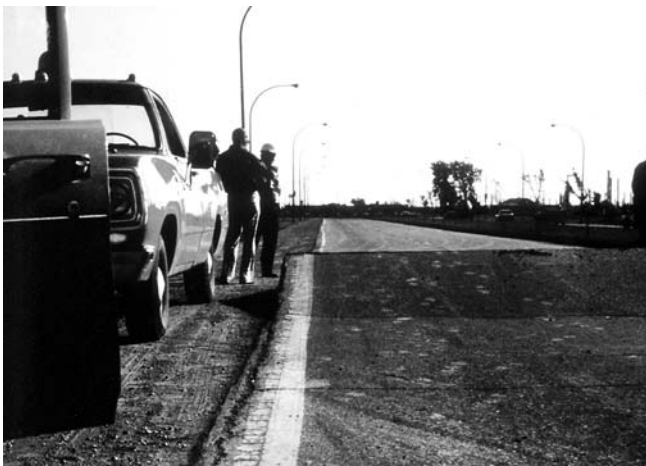
FIG. X2.3 High-Severity Blowup/Buckling
