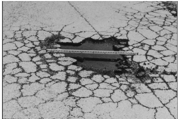
FIG. X1.37 High-Severity Pothole
