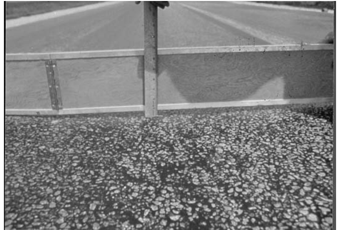
FIG. X1.42 Medium-Severity Rutting
