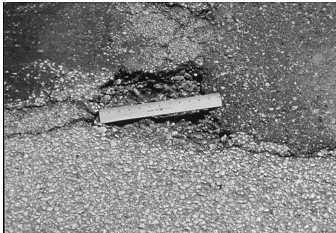
FIG. X1.35 Low-Severity Pothole
