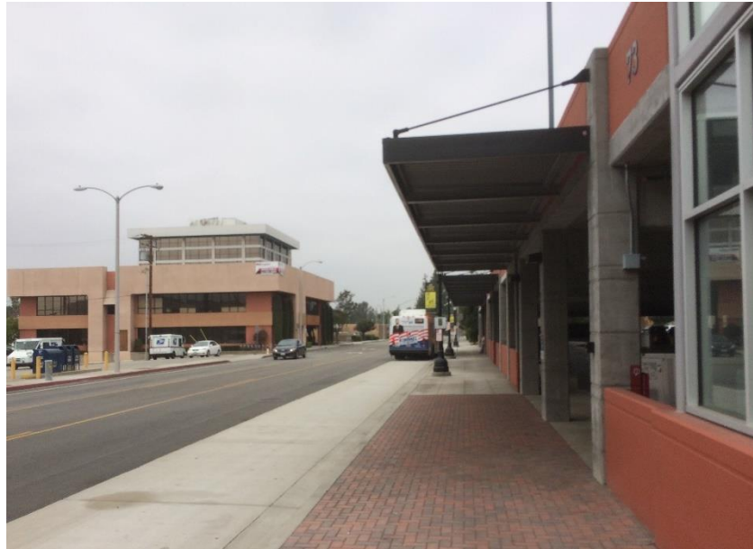
Photo 95: Bus Layover along East Santa Clara St. Prior to Garage Entrance/Exit
