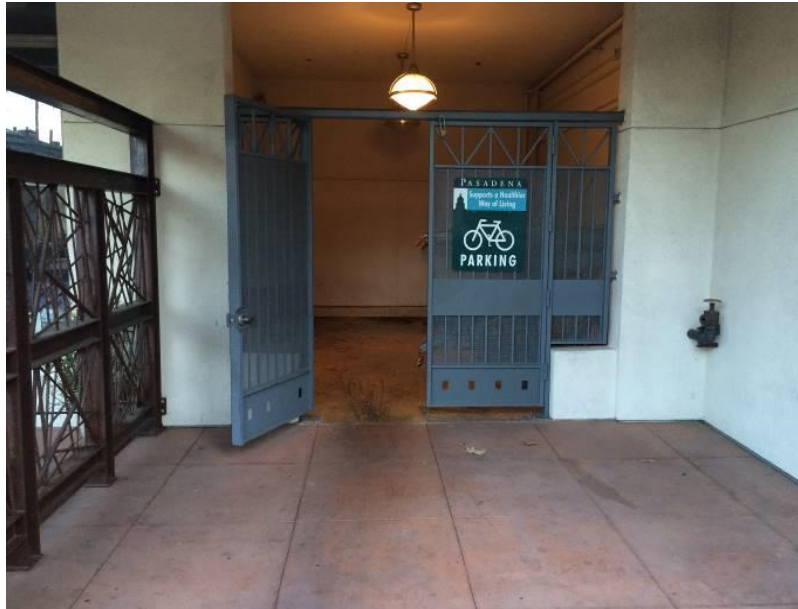
Photo 80: Entrance to Bicycle Room
