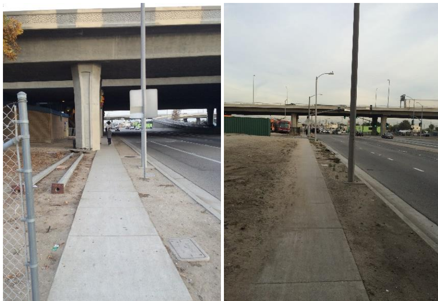
Photo 8: Sidewalks along Wilmington Ave.
