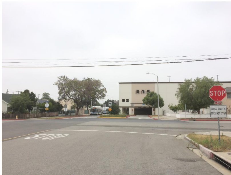
Photo 111: Parking Garage Entrance and Exit with Minimal Signage
