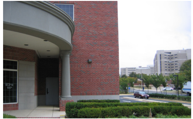
Figure 9(b). View from parking lot.
