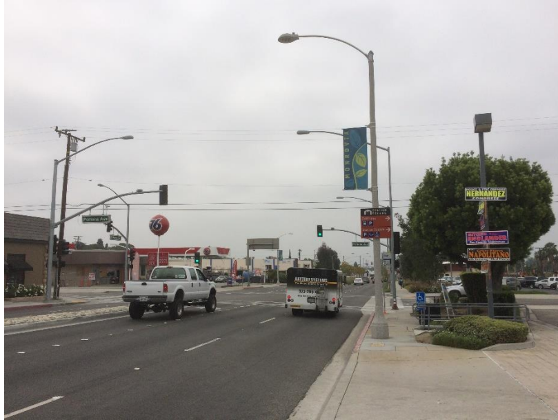
Photo 99: Signage along South Myrtle Ave. Directing to Station Platform and Parking
