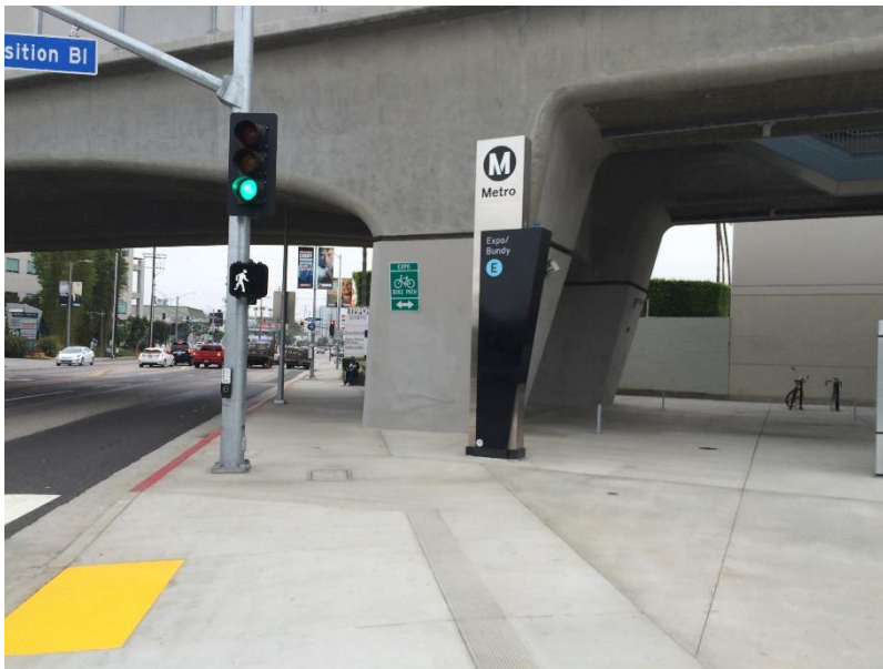
Photo 46: Sidewalks near Station Platform
