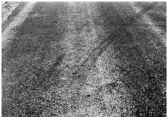
FIG. X1.4 Low-Severity Bleeding
