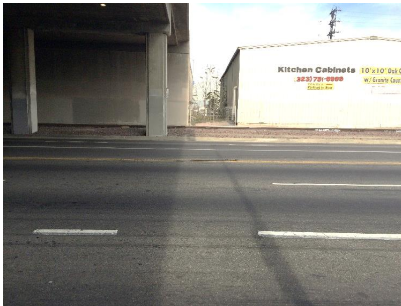
Photo 217: No Sidewalk on North Side of Slauson Ave.
