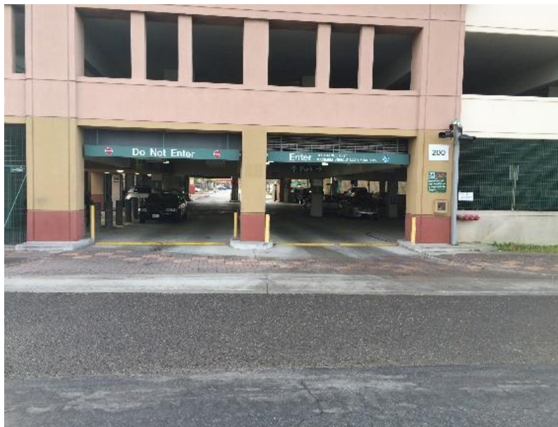
Photo 27: Parking Structure Signage at Willow St. Entrance
