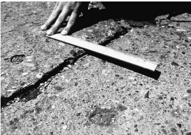
FIG. X2.14 Medium-Severity Faulting
