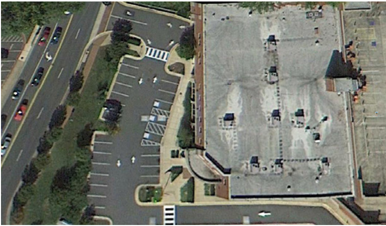
Figure 9(a). Site photo.
