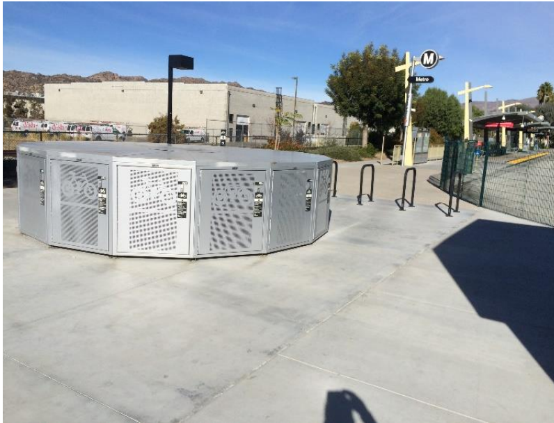
Photo 200: Bike Lockers and Racks
