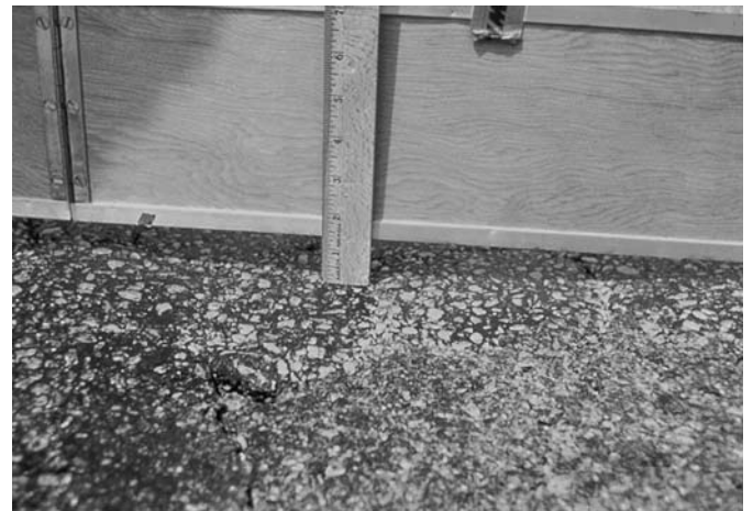
FIG. X1.43 High-Severity Rutting
