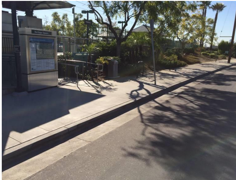
Photo 67: Bike Racks Adjacent to Platform along Marmion Way
