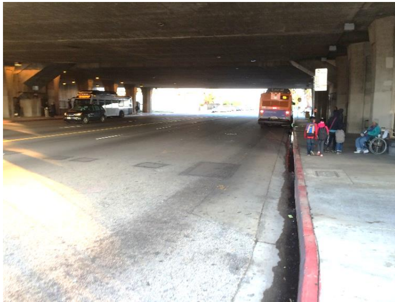
Photo 132: Station Entrance/Exit under I-105
