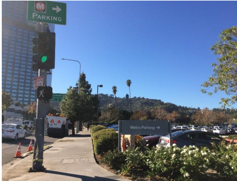
Photo 210: Sidewalk along Lankershim Blvd. Facing South
