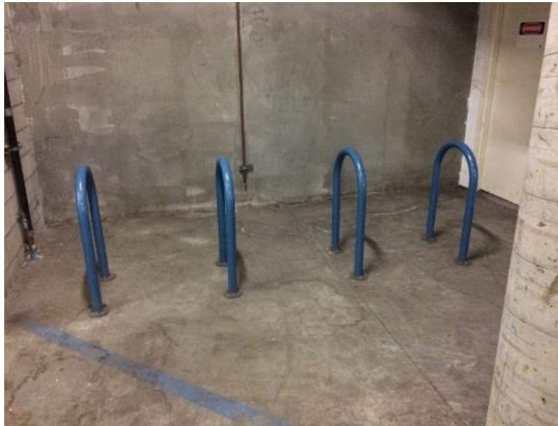
Photo 71: Bike Racks in Parking Structure
