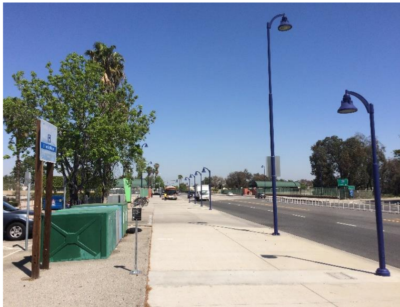
Photo 122: Bicycle Lockers Adjacent to Sidewalk
