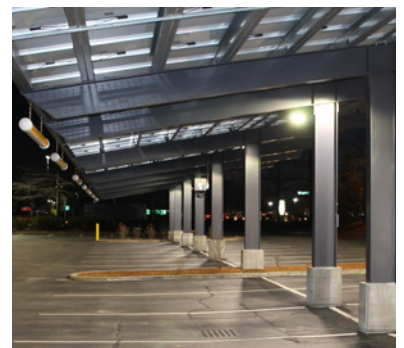
Figure 3. A parking lot recently retrofitted with covered parking. The covering incorporates PV panels that supply renewable energy to the site. Luminaires are mounted to the support structure for the PV panels.
