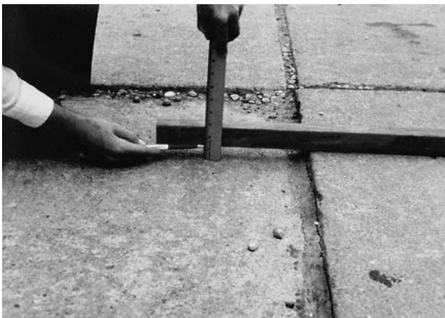
FIG. X2.15 High-Severity Faulting
