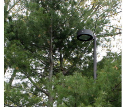
Figure 2. Tree foliage can block light from luminaires.
