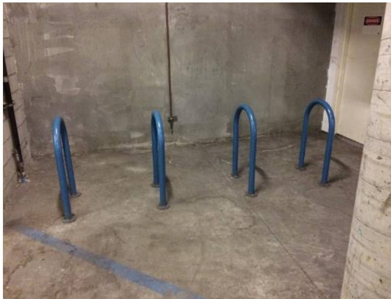
Photo 71: Bike Racks in Parking Structure
