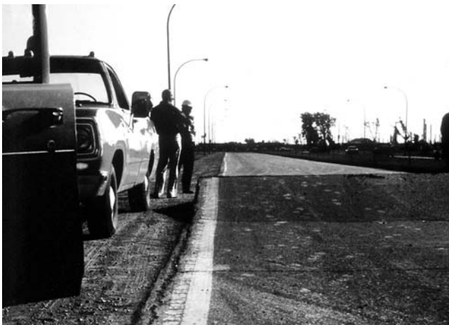
FIG. X2.3 High-Severity Blowup/Buckling
