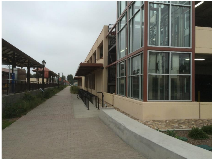
Photo 96: Bicycle Racks between Structure and Platform
