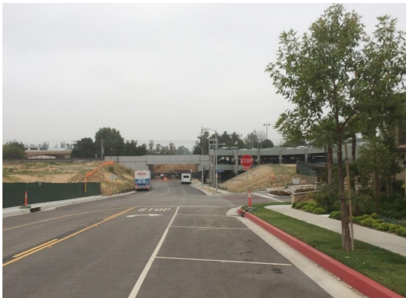
Photo 115: View along Citrus Ave. of Parking Garage
