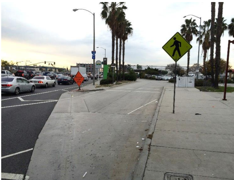
Photo 149: Walkway Leading to Station from Sidewalk on West Side of Crenshaw Blvd.
