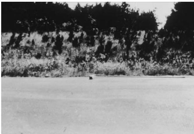
FIG. X1.50 Example Swell. Severity level is based on ride quality criteria.
