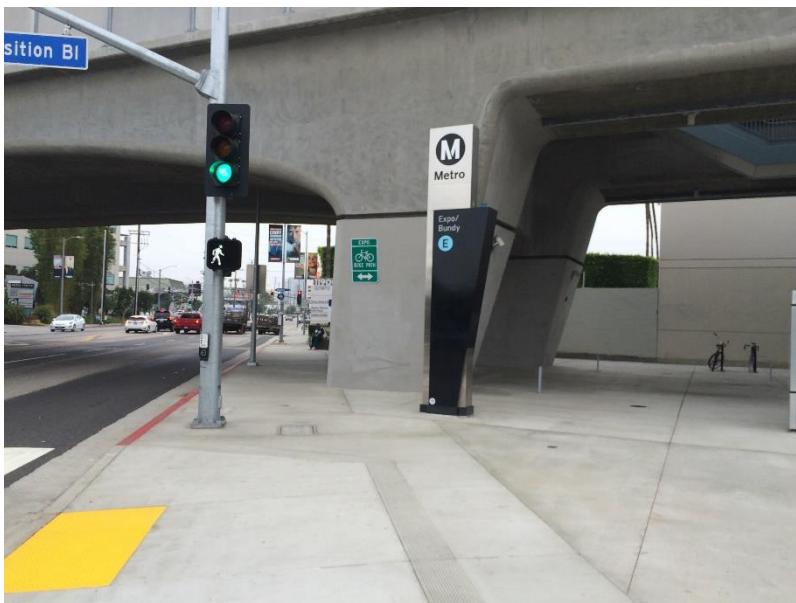
Photo 46: Sidewalks near Station Platform
