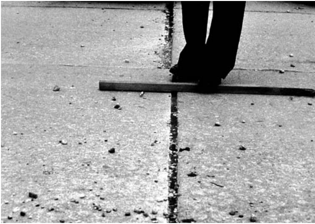
FIG. X2.13 Low-Severity Faulting
