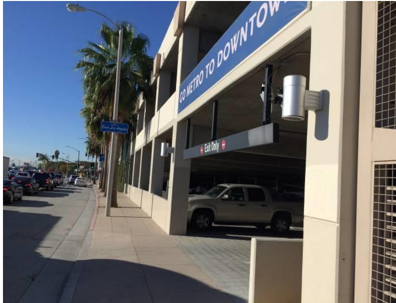
Photo 58: Signage at Entrance to Parking Structure
