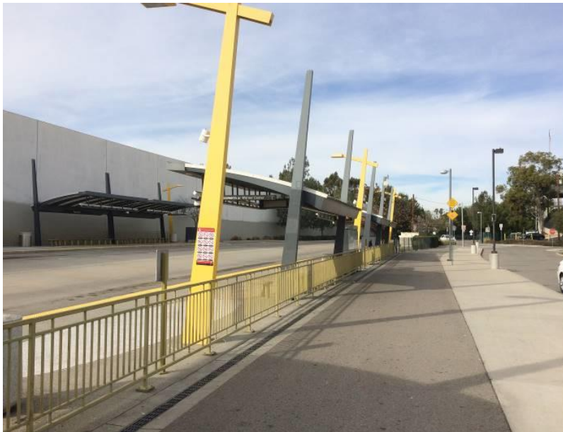
Photo 179: Orange Line Pedestrian and Bicycle Path
