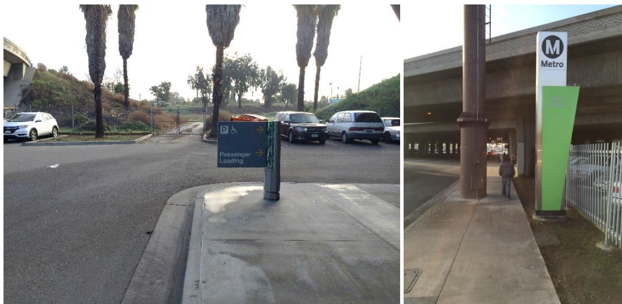
Photo 130: Minimal Signage at Lot Entrance (L); Station Monument Sign (R)
