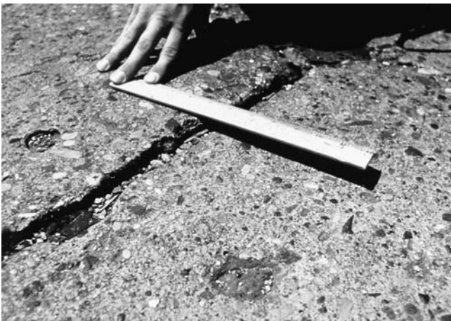
FIG. X2.14 Medium-Severity Faulting
