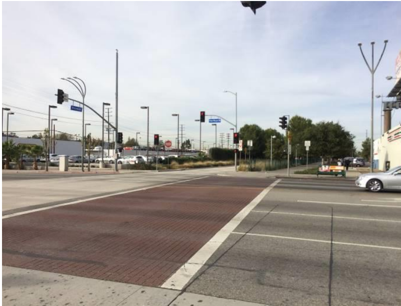
Photo 173: Orange Line Pedestrian and Bicycle Path
