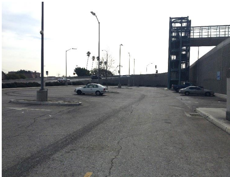
Photo 218: Staircase in East Lot to Provide Access to Station Platform
