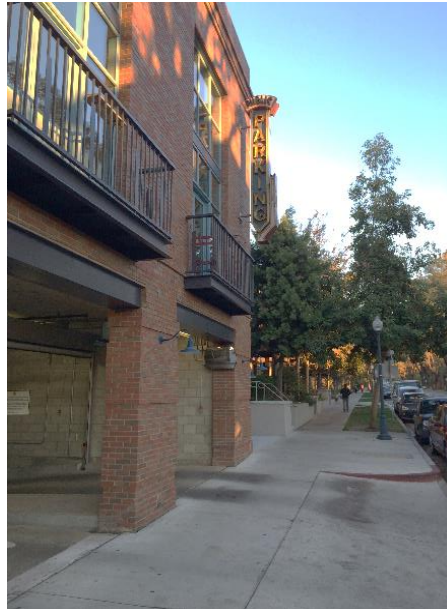
Photo 74: Parking Structure Entrance
