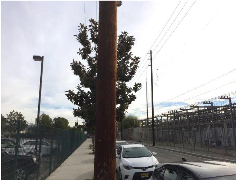
Photo 175: Sidewalk along Aetna St.
