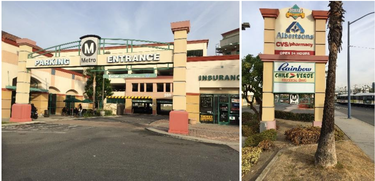
Photo 26: Large Monument Sign at Entry to Parking Structure (L); Small Metro Sign on Shopping Center Monument Sign (R)
