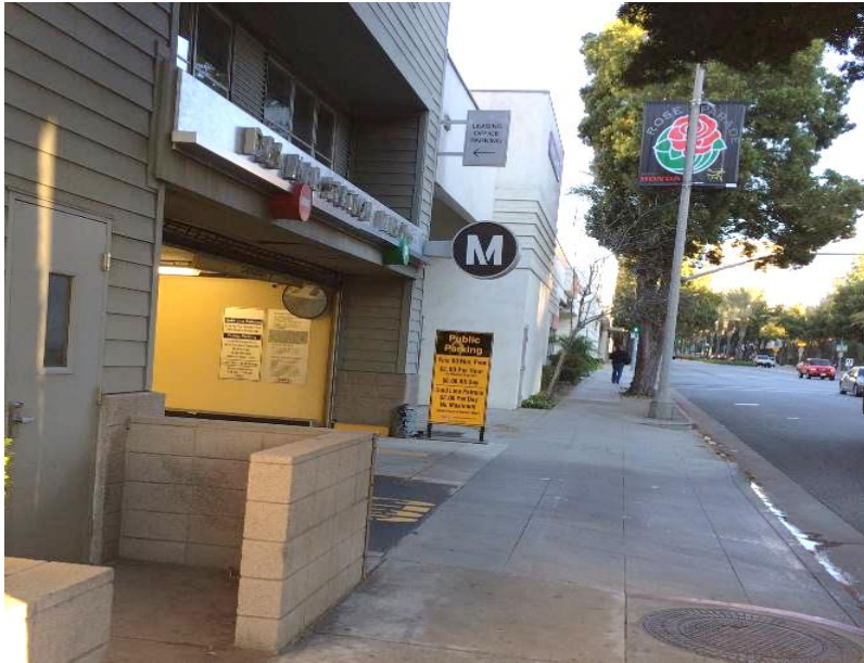
Photo 84: Metro Signage at Entrance to Parking Garage
