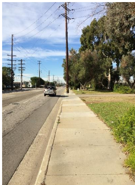
Photo 169: Sidewalk along Marine Ave. Facing West
