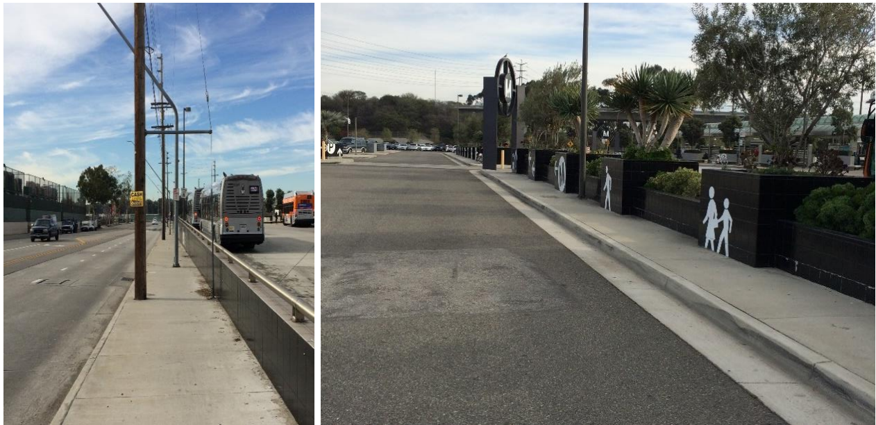
Photo 230: Sidewalk along West 182nd St. (L); Sidewalk within Parking Lot (R)
