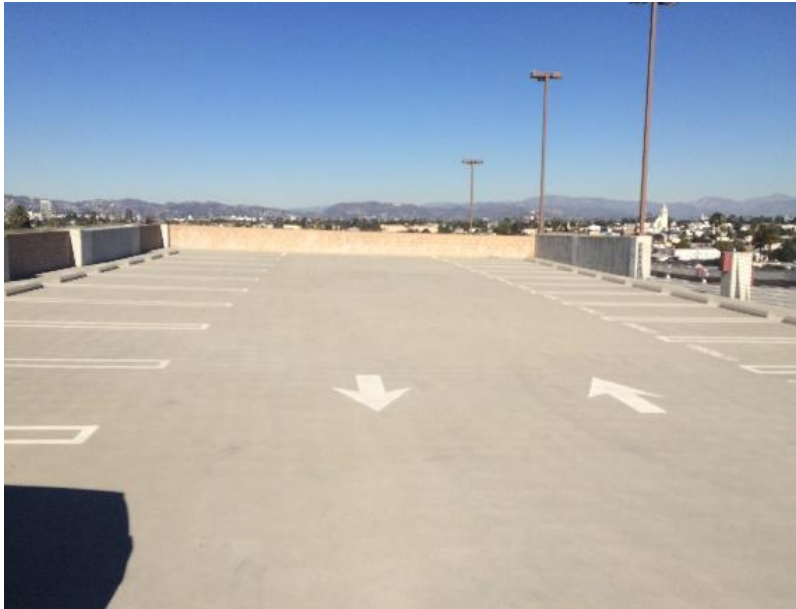
Photo 30: Roof of Parking Garage
