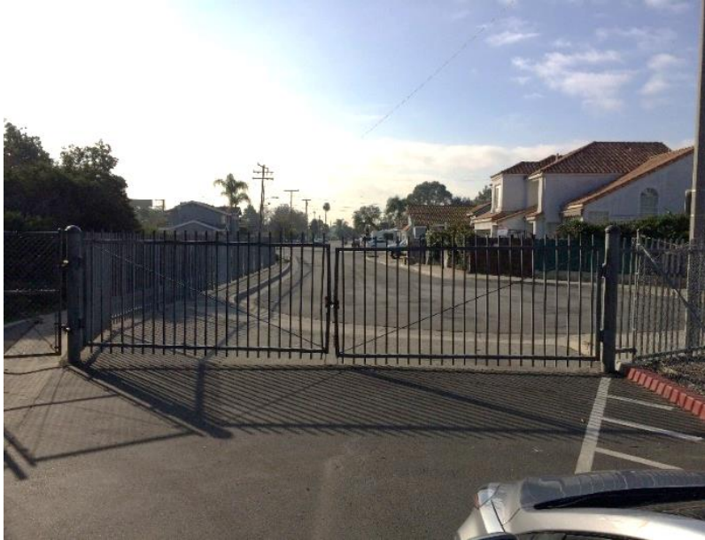
Photo 120: Barrier Gate at Flatbush Ave.
