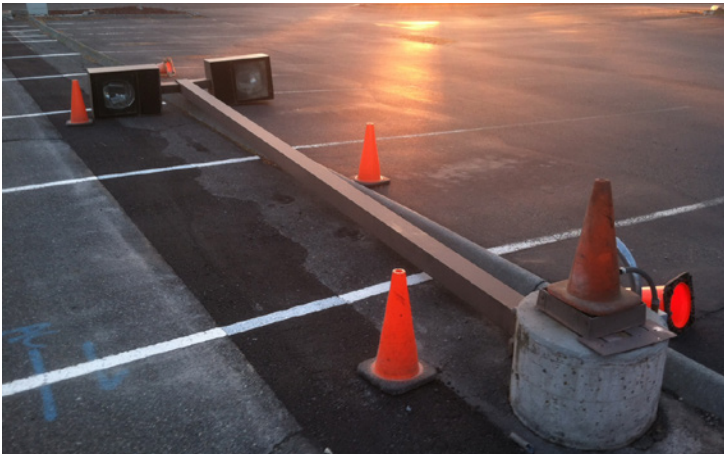
Figure 1. A pole and luminaires being removed and replaced with new equipment.
