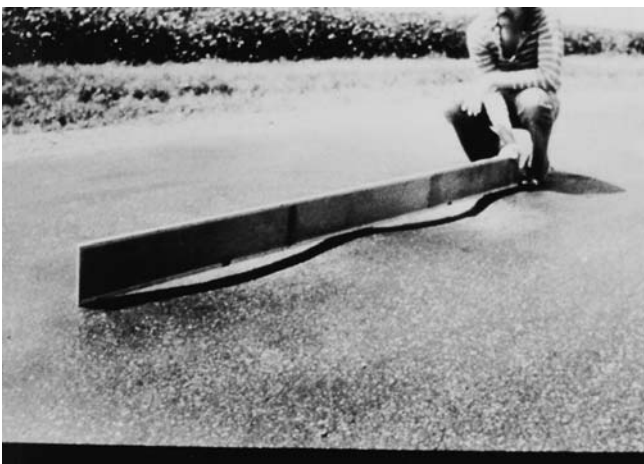
FIG. X1.15 High-Severity Corrugation
