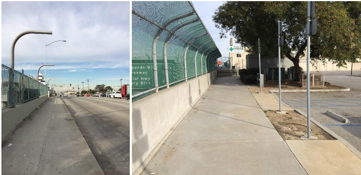
Photo 225: Trash on Sidewalk along Rosecrans Ave. (L); Sidewalk within Parking Lot (R)
