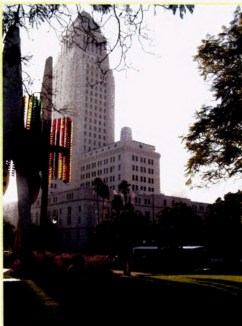
Los Angeles' historic City Hall, as seen from the corner of Main and Temple Streets, adjacent to the alignment of the At-Grade Emphasis LRT Alternative
