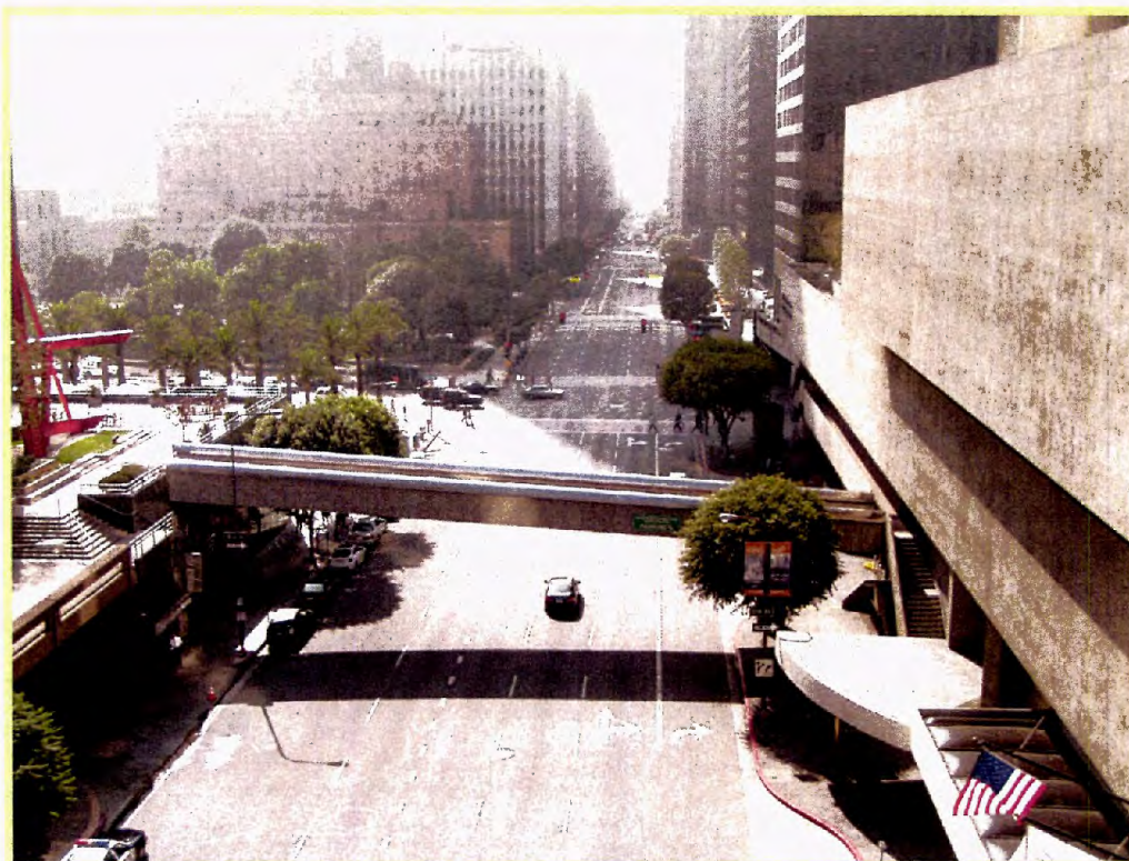
Wide roadway on Flower Street near 5 th Street, with six automobile traffic lanes and one curb lane of parking. This segment of Flower Street carries about 20,000 cars on a typical weekday.
