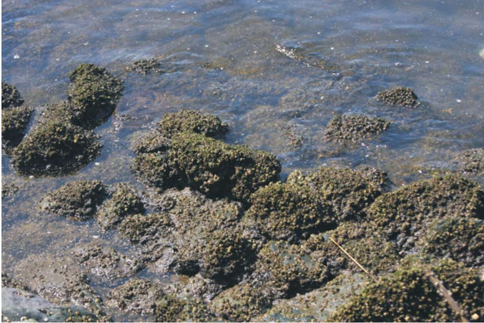
Figure 8 - Protective riprap at the water's edge.
