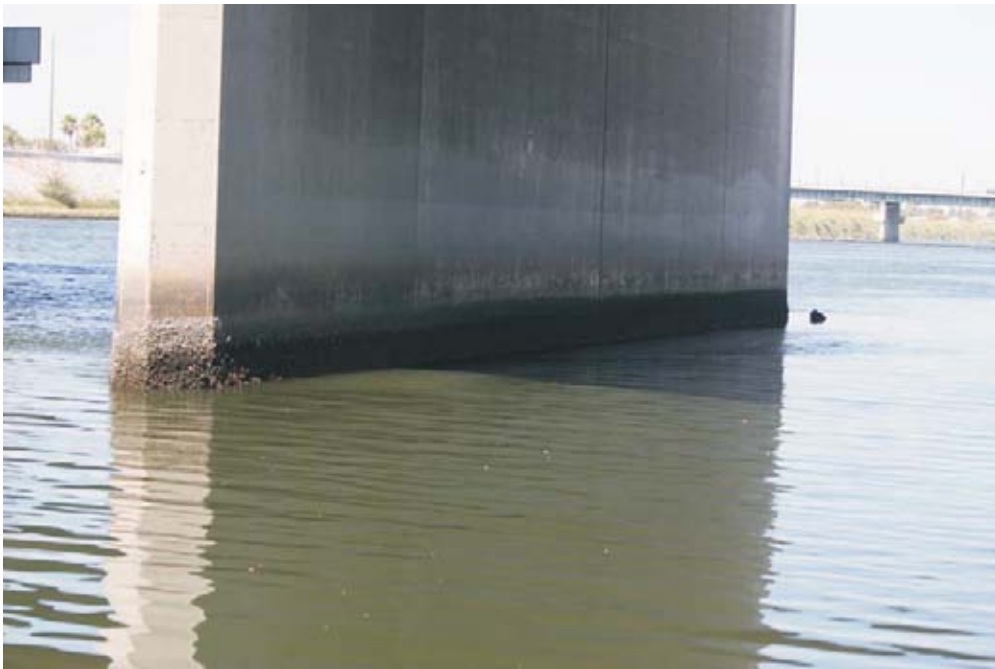
Figure 13 - Base of the bridge abutment at Anaheim Street, showing colonization by barnacles and other fouling species of invertebrates.
