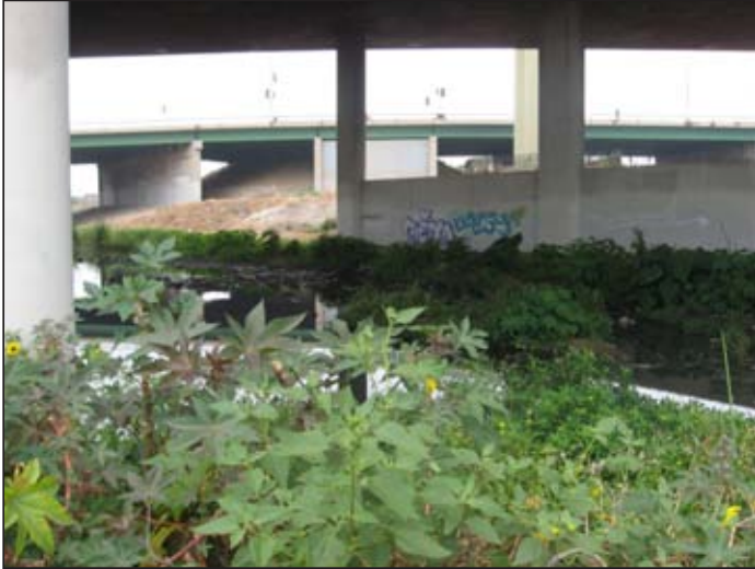
PHOTOGRAPH 5: View of wetland area located in Compton Creek (Drainage 7) at SR-91.
