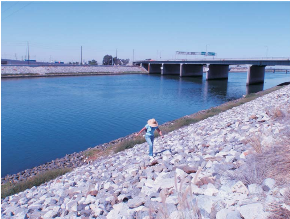
Figure 7 - Riprap shoreline south of Shoemaker Bridge (October 1, 2009).
