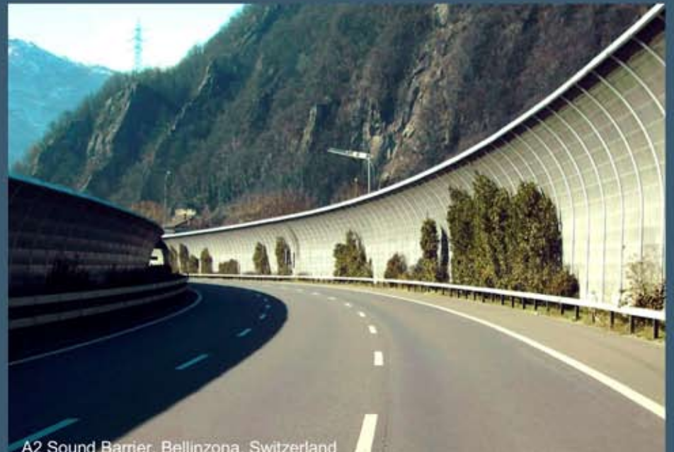
A2 Sound Barrier, Bellinzona, Switzerland
