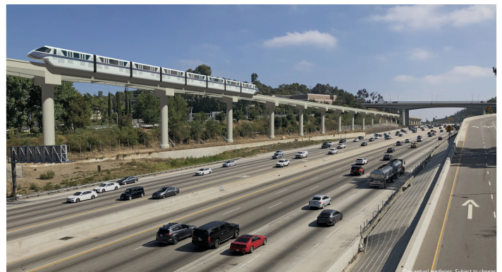
Figure 5-6. MRT 1, Looking North at Mulholland Drive Bridge
