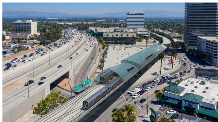
Figure 5-4. HRT 3, Looking North at Sepulveda Boulevard/Ventura Boulevard Station Source: Sepulveda Mobility Partners, 2019
