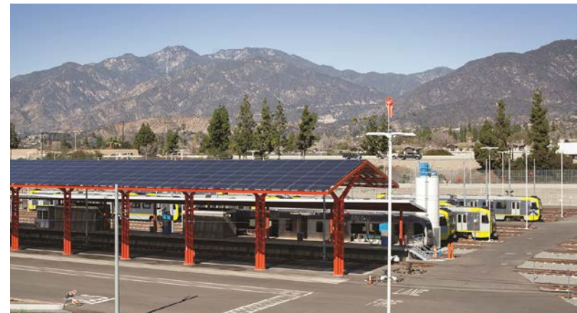
Gold Line Foothill Extension MSF Yard
