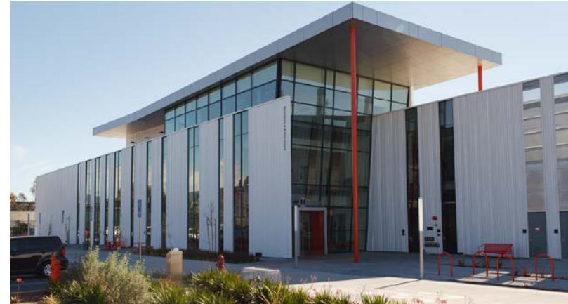
Gold Line Foothill Extension MSF Building
