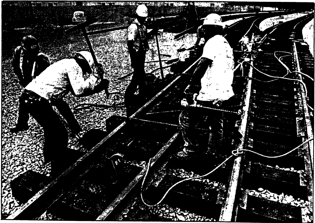
Workers with California Engineering Contractors Wednesday work to lay track for a Metrolink layover facility in Moorpark. DAVID HARTUNG/News Chronicle
