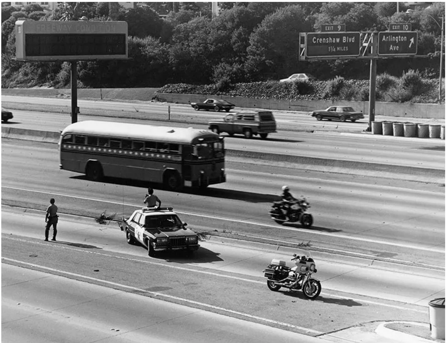
A bus carrying athletes travels down the 10 freeway during the games. In addition to sensors, giant digital signs were installed on major roads to relay messages to motorists. | Courtesy Los Angeles Public Library
