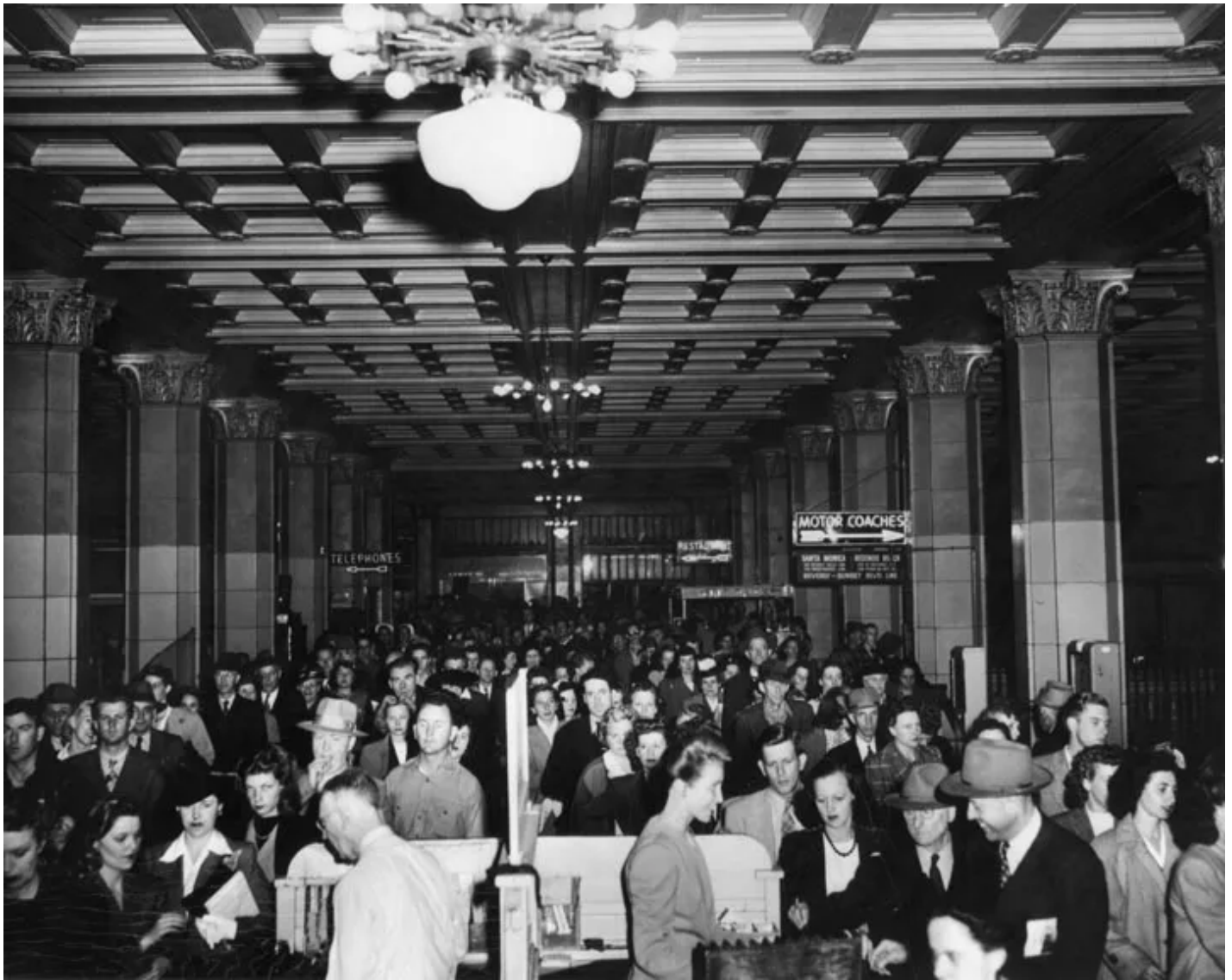
Inside the Subway Terminal Building.
