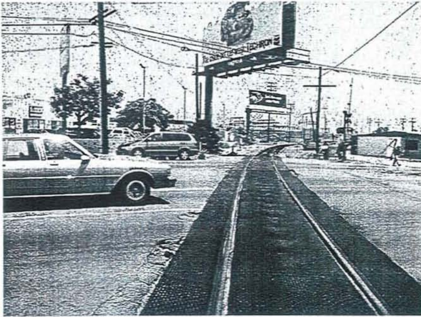
Figure 2.3: View of constrained right-of-way and utility overcrossings near the I-405 freeway in the City of Inglewood.
