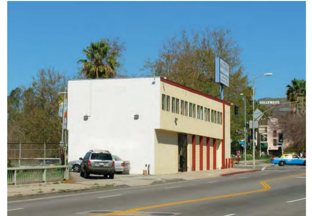
Buildings such as this one face away from the 101 freeway
