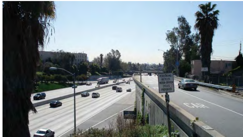
South-bound on-ramp from Hollywood Blvd
