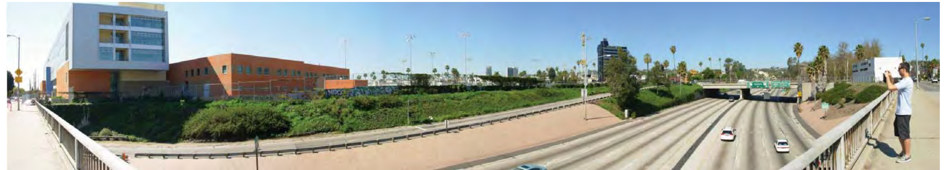
Panorama- View from Wilton Place overpass looking south-west to north west
