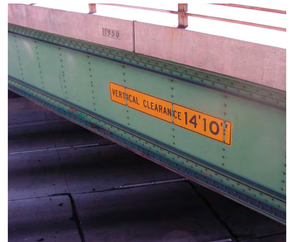
Figure 3.8 - Existing Western Avenue Overcrossing with Sub-standard Vertical Clearance
