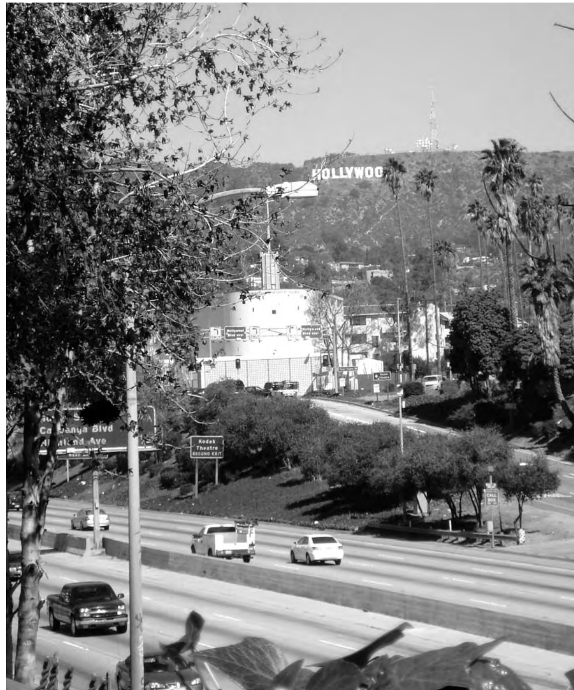
Existing ~ Hollywood Boulevard off-ramp and freeway
