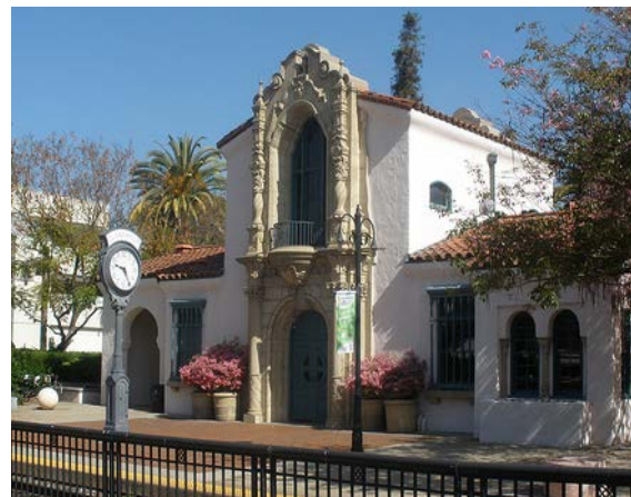
Claremont Metrolink Station (Category #6) Claremont, CA
