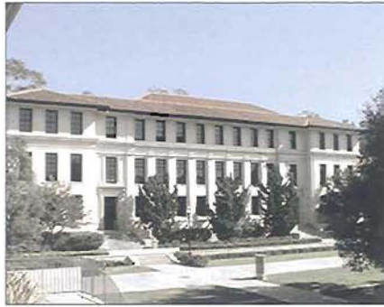
Institutional Building : Occidental College
