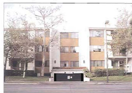
Typical apartment building
