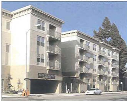
Commercial Housing, Pasadena
