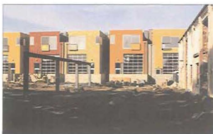
Architect : Mark Mack
