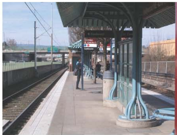
Figure 3 The Hollywood Station, Located Between Heavy Rail and the Freeway
