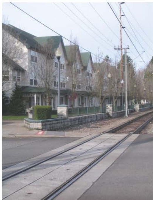
Figure 4 Looking at Both Sides of the Gresham Station
