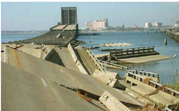
Louisiana Hurricane Katrina U.S. 90 Ocean Springs
