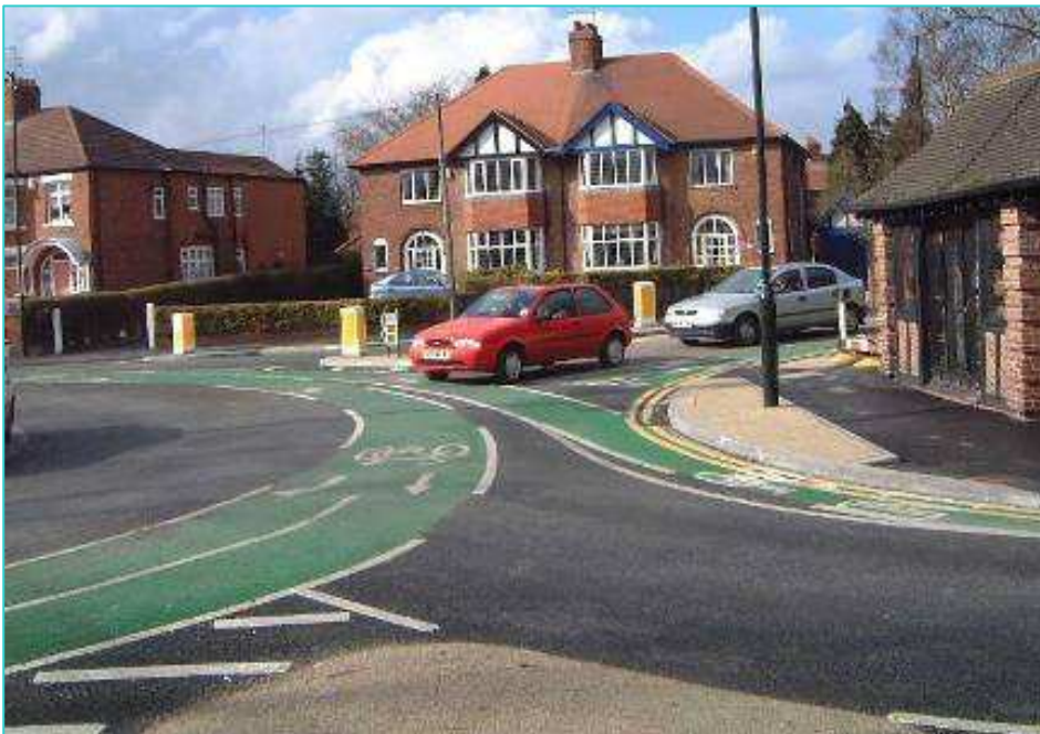
Figure 3.19 Directional cycle lanes around a roundabout in York, England (unknown source)
