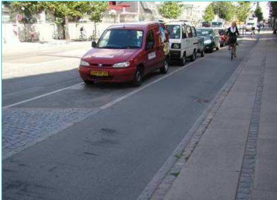
Figure 3.12 Cycle lane inside parking space, Denmark (H Barber)
