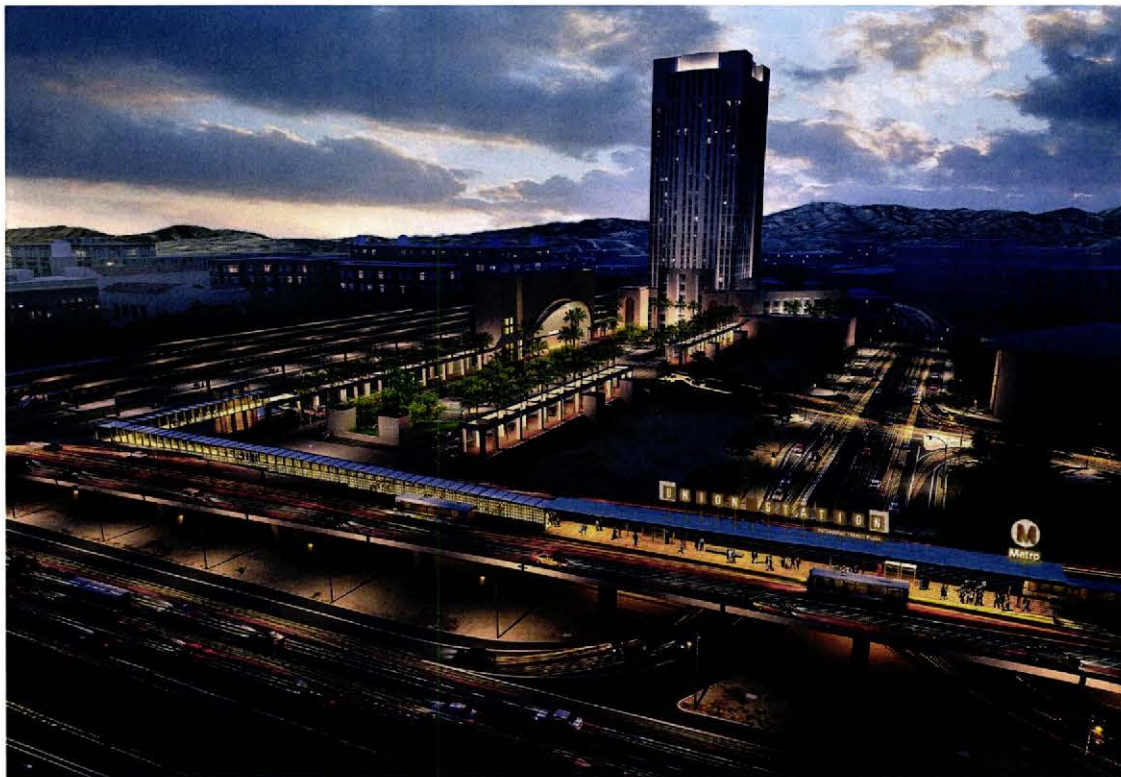
Figure 1.17 Patsaouras Plaza Busway Station
