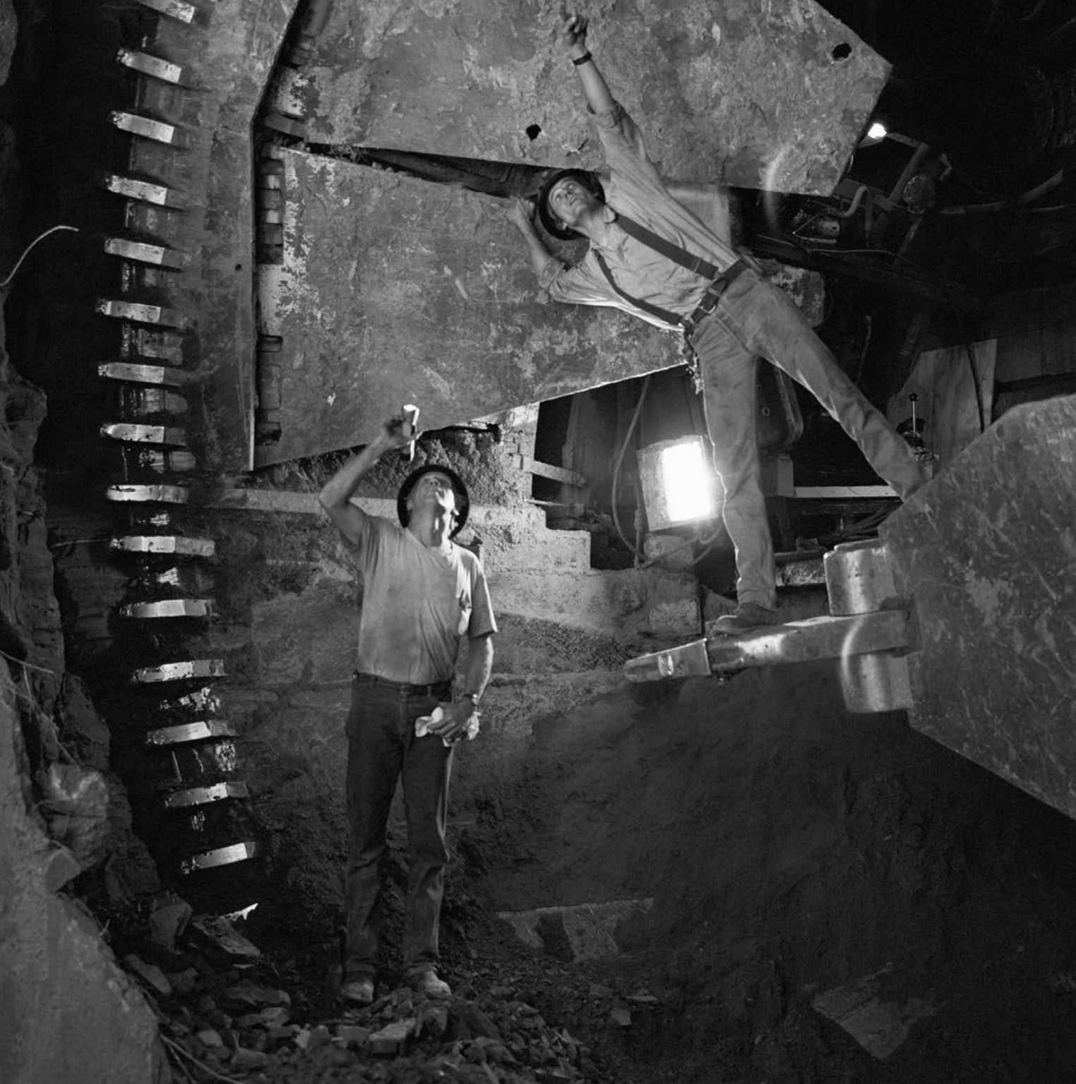
Two miners inspect the breasting plates and teeth of the shield machine soon after it broke through to the station at 6th St and Vermont St. Two tunnels were bored underground from the construction site at Barnsdall on Hollywood Bl.
