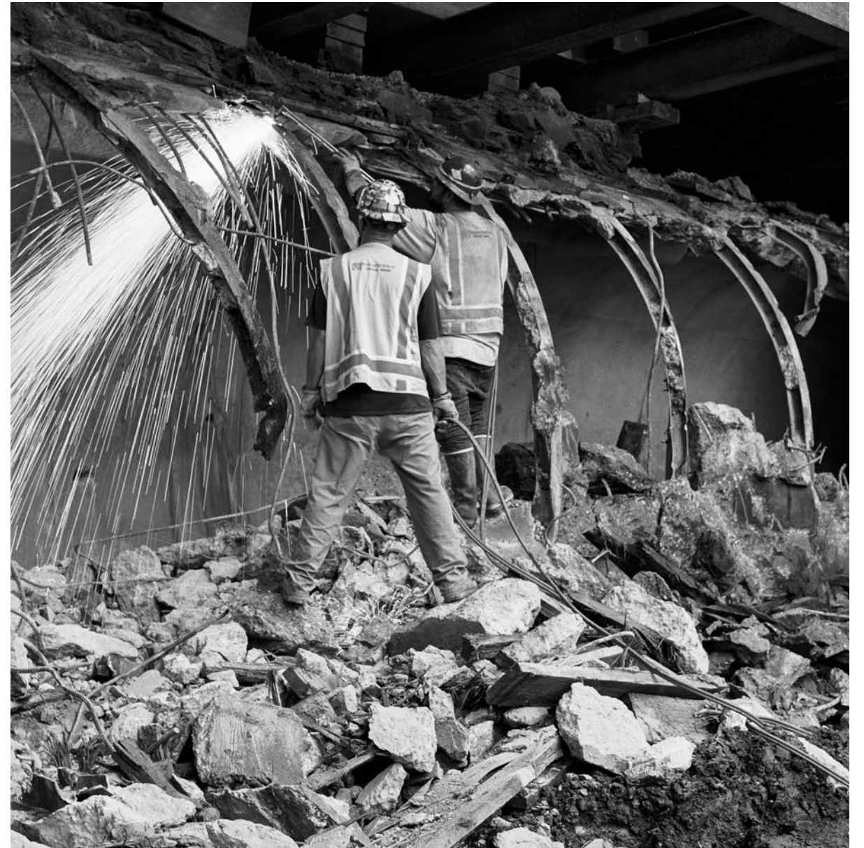
Construction workers dismantle a concrete storm drain under 2nd Street at the future station.
