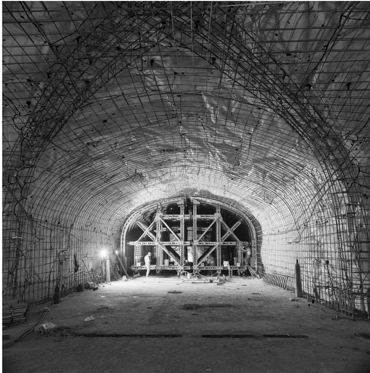
The concrete formwork assembly is shown within the Red Line Track Level Rooms excavated under the Santa Monica Mountains. These rooms house the gear controlling the crossover and the track and power equipment.
