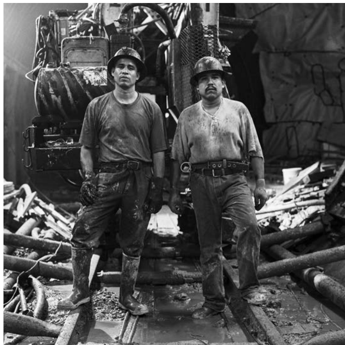
Karagozian relays, "In 1999, at the Red Line Subway Grand Opening weekend my photographs were on display and I met Hector and Alex Barajas' parents and siblings. The brothers were so proud to share that they were part of the construction crew that helped build the Metro Red Line."
