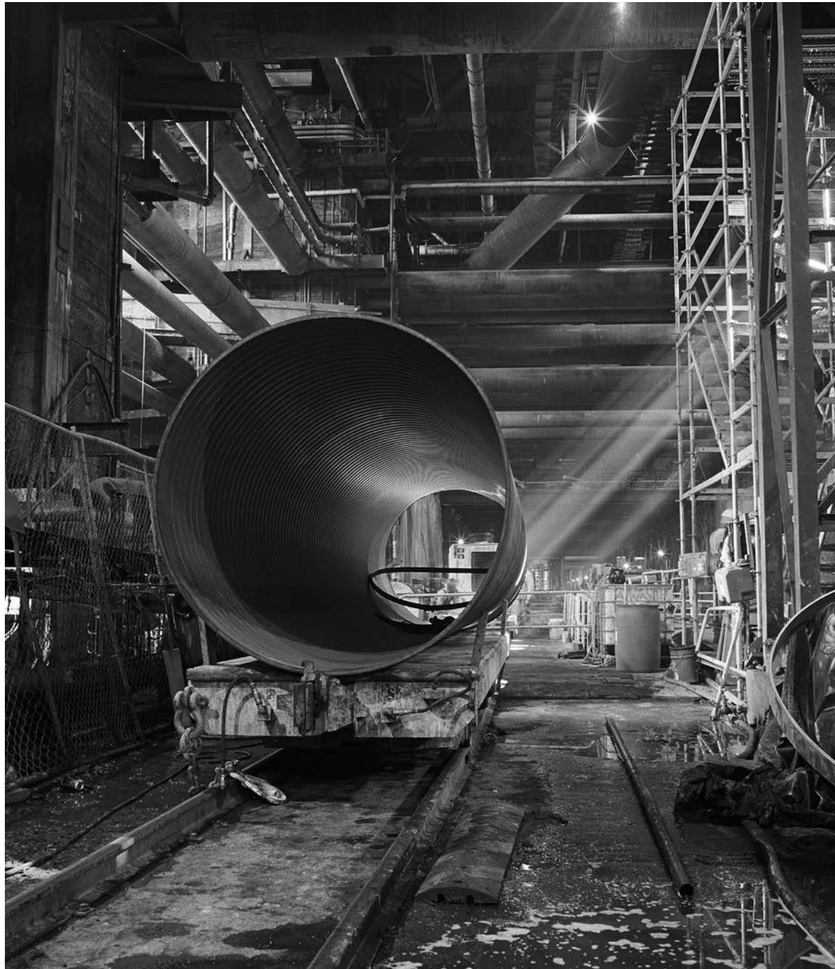
Sunlight filters into the bottom landing at the future station, where a section of air duct waits for transport into a tunnel. As the TBM advances, workers add air ducts, rail tracks and utilities, such as water and power.
