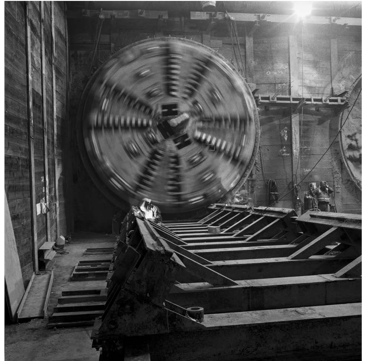
The TBM cutterhead is turning for a press event to showcase the 1.4-mile underground tunnel boring breakthrough in the Gold Line Soto Station. The construction worker is welding the steel cradle for the TBM to be moved onto.
