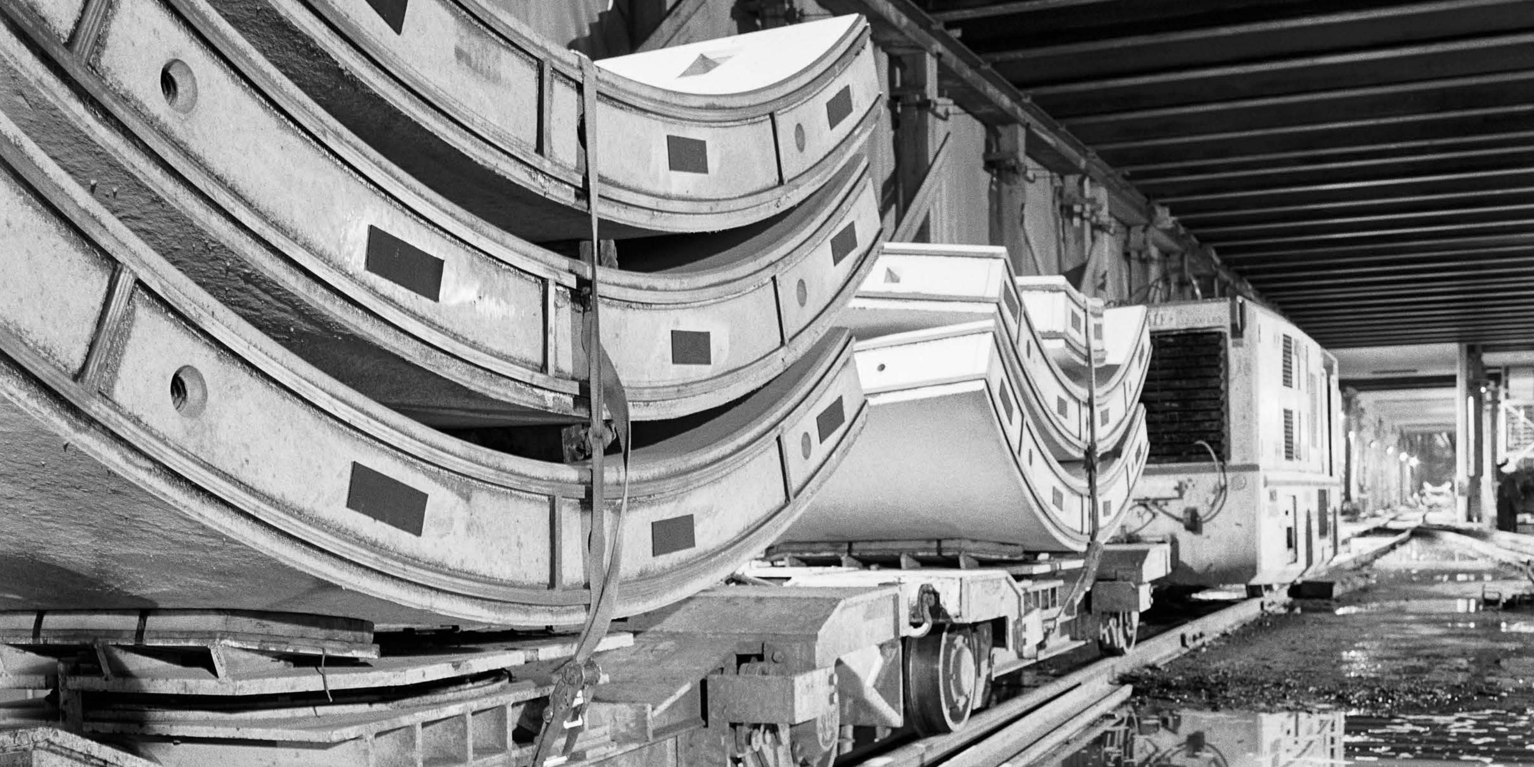
Concrete segment tunnel liners are reflected in puddles of rain water at the bottom landing of the future station. The rail cars deliver these tunnel segments to the TBM.
