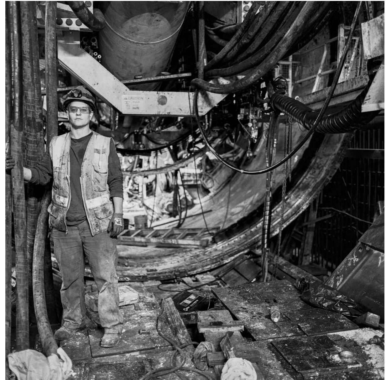
Ilana Feingold, Electrician, is pictured here inside the TBM.
