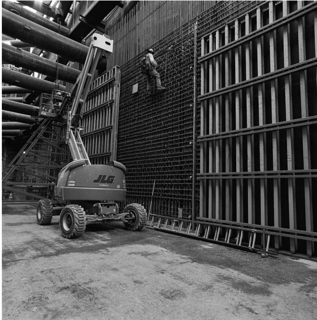
Karagozian shares, "A worker is weaving the rebar to reinforce the new concrete wall being built. Photographing ironworkers walking on the steel is like watching a trapeze artist at work."
