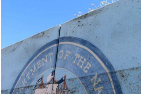
Photo 13: Detail of Navy insignia at northwest wall; note mural continues through vertical expansion joint.
