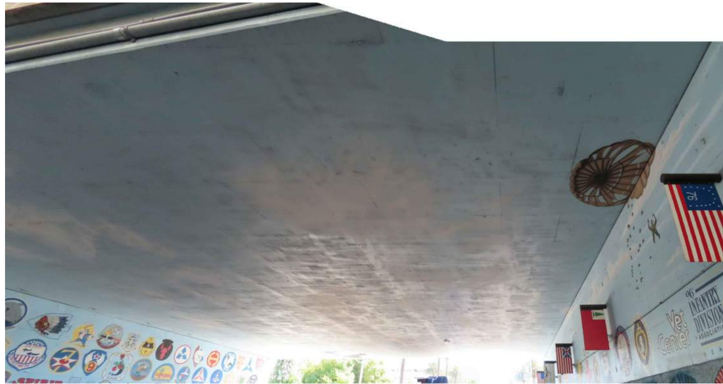
1 UNDERPASS CEILING - VIEW SOUTH NOT TO SCALE
