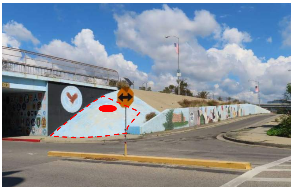
Figure 10 – Southeast retaining wall and corner slope (Wilshire Blvd. on-ramp, eastbound). Note proposed column location (in red) and proposed area of concrete slope to be removed (dashed lines). (source: ARG)
