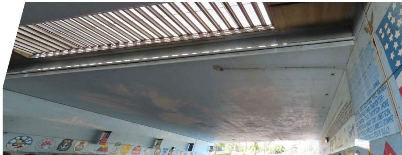
1 UNDERPASS CEILING - VIEW NORTH NOT TO SCALE
