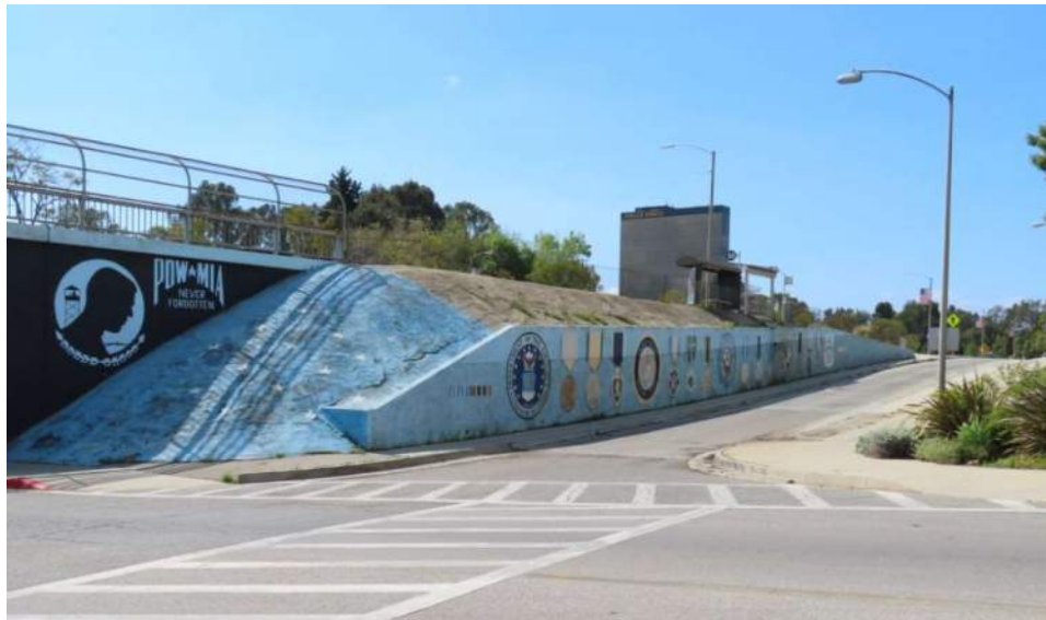
Figure 5 – Northwest retaining wall (Wilshire Blvd. on-ramp, westbound). (source: ARG)
