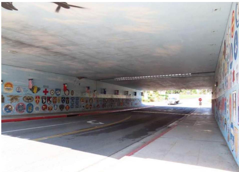
Figure 4 – Bonsall Avenue Underpass, view north (source: ARG)
