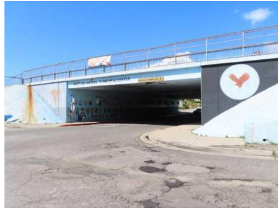
Photo 2: Wilshire Blvd. bridge, south elevation.
