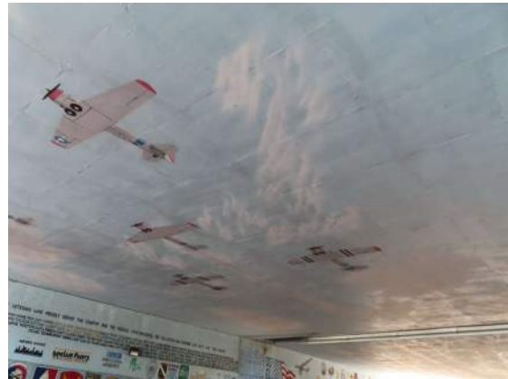
Photo 4: Bonsall Ave. underpass ceiling; note biplanes and clouds. Also note plywood sheet form lines at concrete slab.
