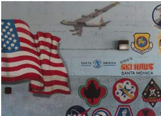
Photo 37: Detail of east elevation of underpass; note light fixture and surface-mounted conduit.
