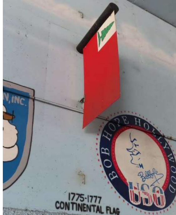
Photo 36: Flag on stanchion at west elevation of Bonsall Ave. underpass; note cut off angle below, indicating flag was raised.
