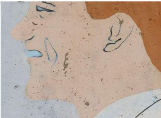
Photo 21: Detail at southwest wall; note paint loss at face.
