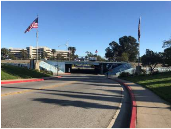
Photo 1: Wilshire Blvd. bridge crossing at Bonsall Ave. view south.
