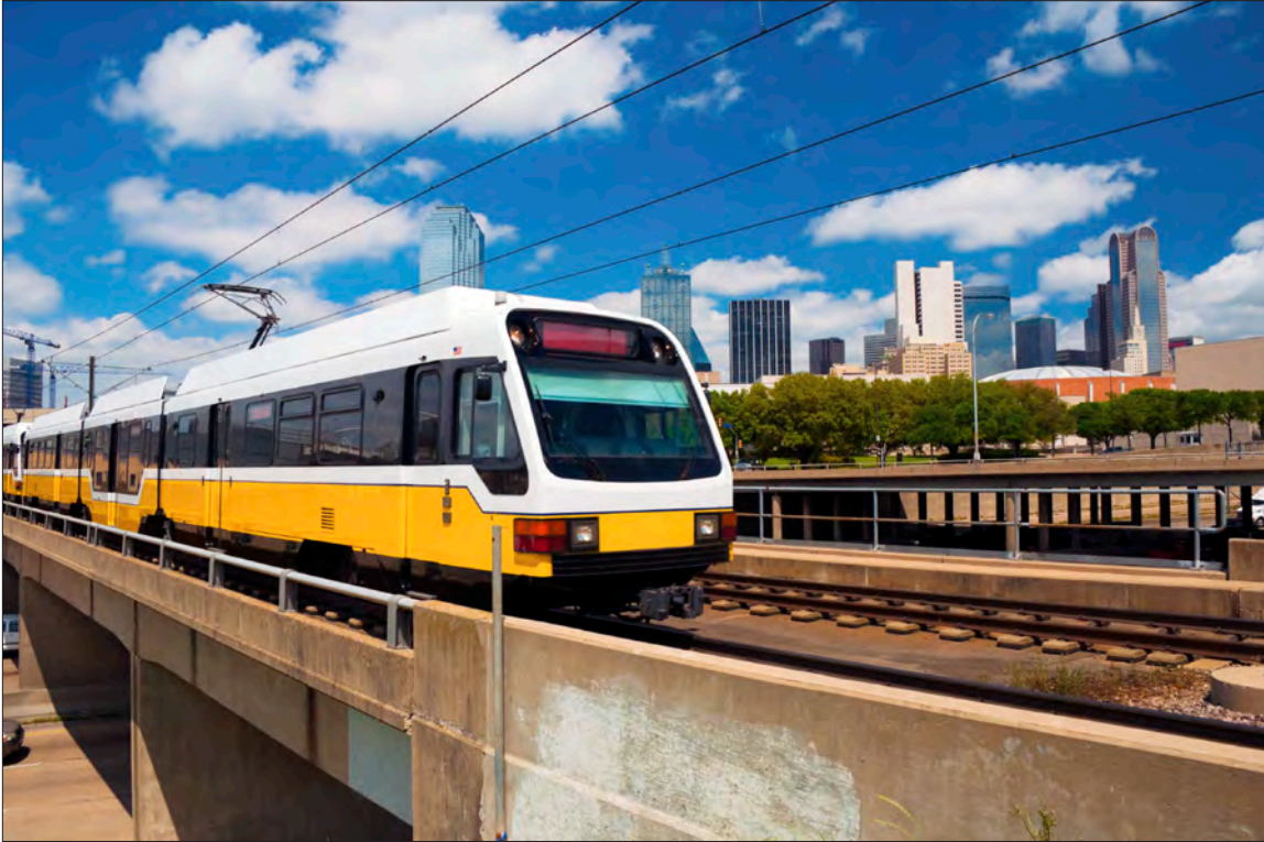
The extension of the Dallas Area Rapid Transit's (DART) orange line received $5 million as a TIGER III project.
