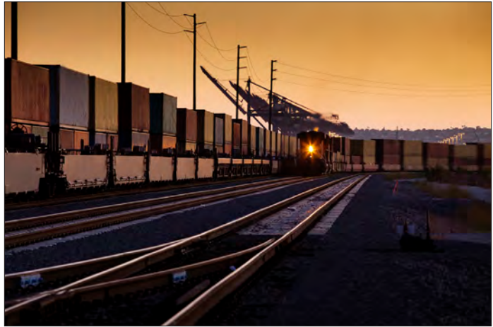
The West Basin Railyard at the Port of Los Angeles received $16 million in funding as a TIGER II project.
