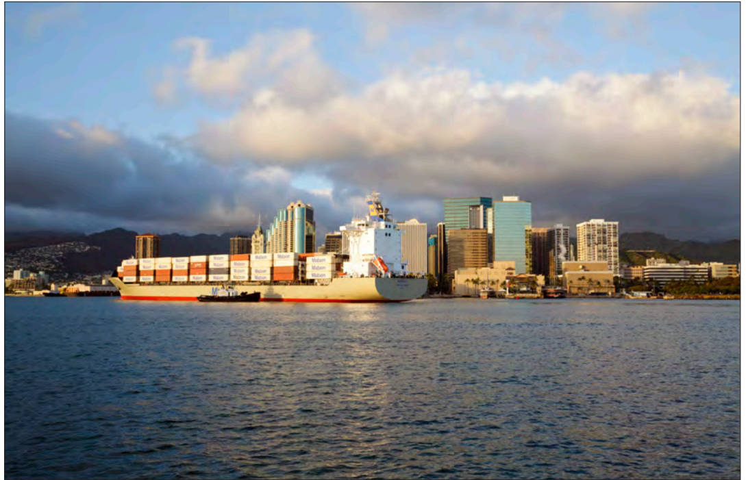
The reconstruction of Pier 20 in Honolulu Harbor was included in TIGER I and received $24.5 million in funding.
