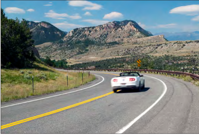
Wyoming's Beartooth Highway Reconstruction Project was included in TIGER I and received $6 million in funding.
